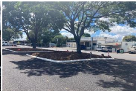
Mulched tree surrounds
