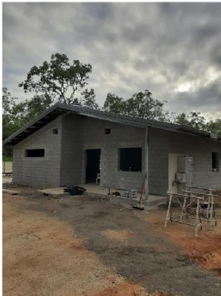
Blockwork and roof works completed
