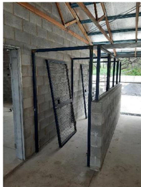
Steel fabricated cage
