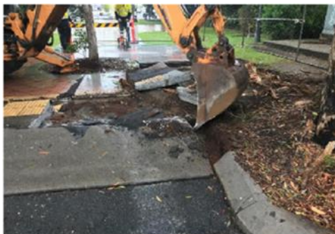
Removal of damaged concrete and tiles at Anzac Park
