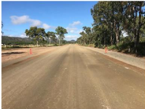
Package 1 prior to bitumen sealing
