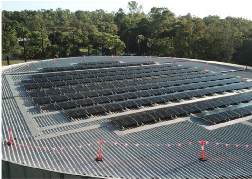
New panels installed on the clearwater reservoir at Mareeba WTP.
