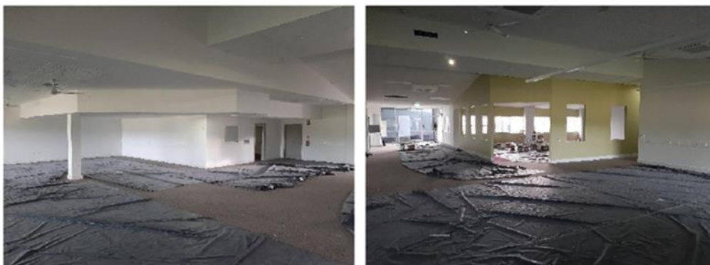
Internal painting complete
