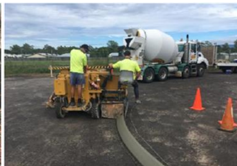
Installation of traffic islands and garden edging
