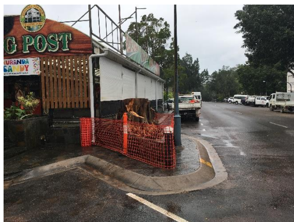
Stump ready for removal by crane
