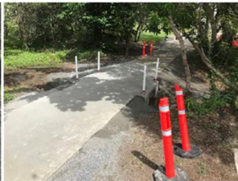
Culvert crossing 80m south-west of MMSS (after)
