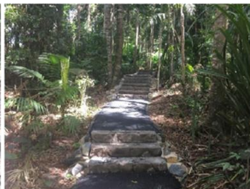
Jungle Trail - Replacement Stone Look Steps
