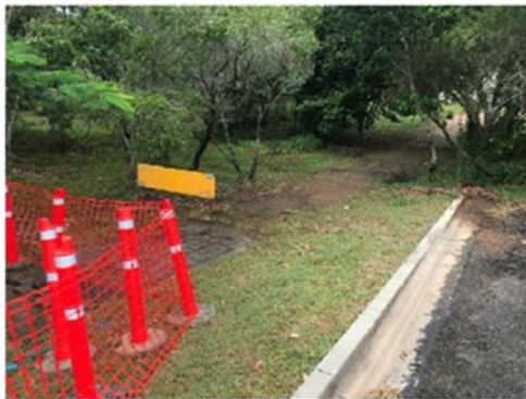
Culvert crossing 80m south-west of MMSS (before)
