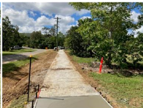
Trees subject to concerns regarding damage from path construction (after)
