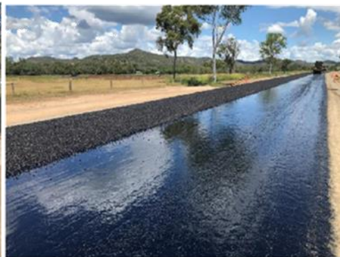
Package 1 during bitumen sealing
