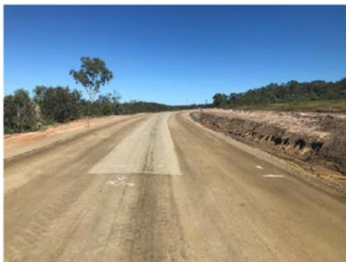
Package 2 Prior To Bitumen Sealing
