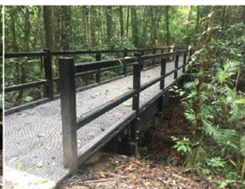
Bridge 6 National Park Section
