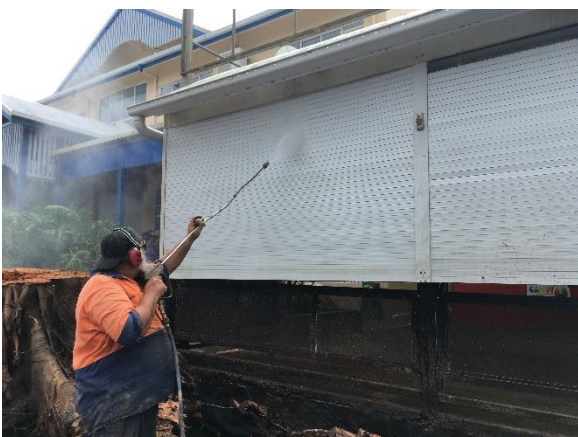
Clean-up after vacuum truck work
