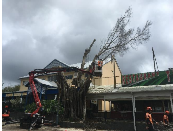
Removal in progress
