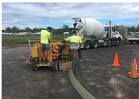
Installation of traffic islands and garden edging
