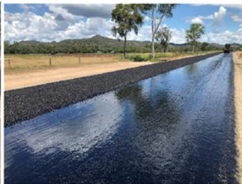
Package 1 during bitumen sealing
