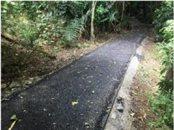
Jungle Trail - Refurbished edge stanchion & asphalt overlay
