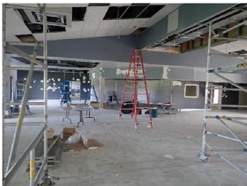
Electrical works underway
