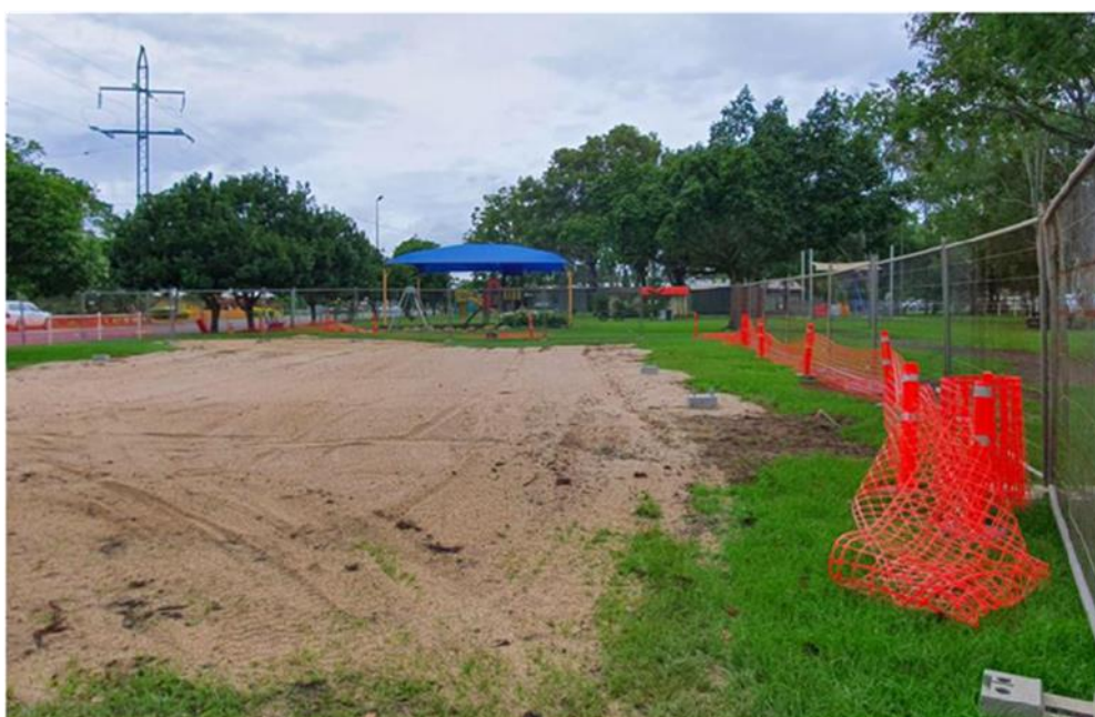
Centenary Park - Earthworks and footings for new structure
