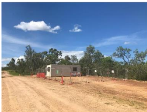
Site office and Compound
