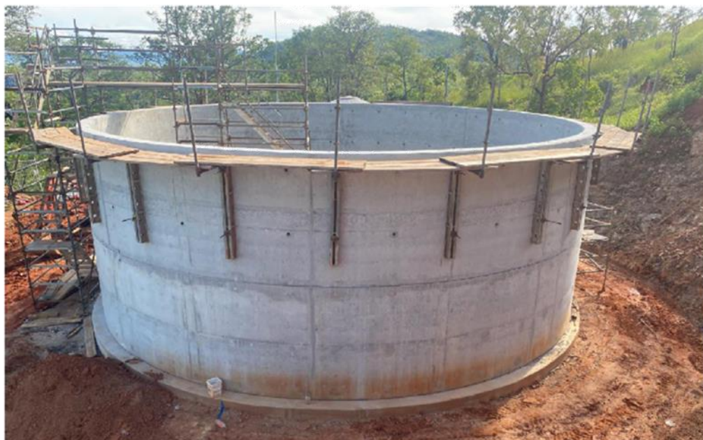
Formwork removed follow curing of concrete
