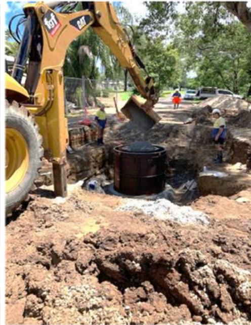
Construction of new sewer manhole at Abbott Street
