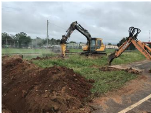
Removing Slabs and Footings - Old Railway
