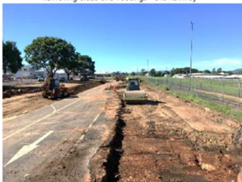
Compacting Select Fill
