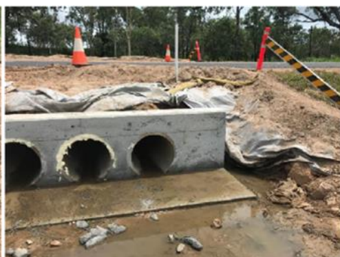
Completed Apron and Headwall
