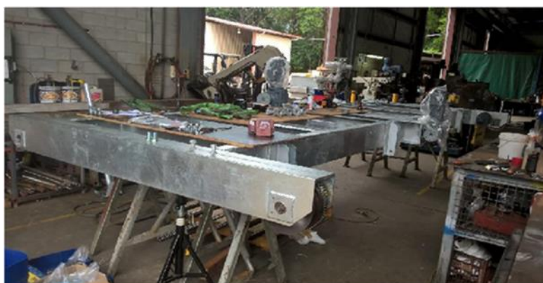
Clarifier trolley assembly
