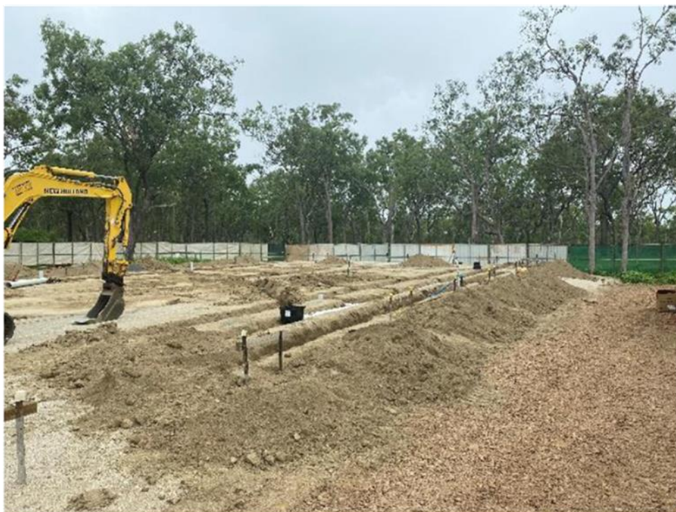
Building Pad partially prepared for substructure
