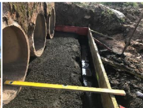
Preparation for Apron
