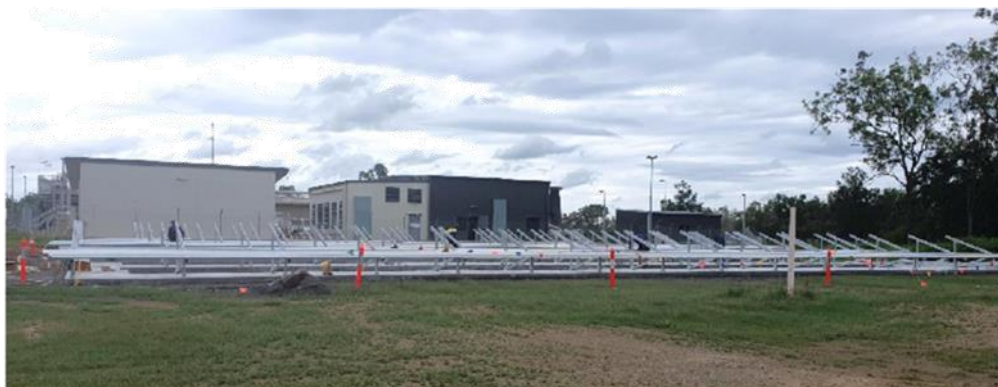
Mareeba Sewage Treatment Plant - Ground Mounted Framework
