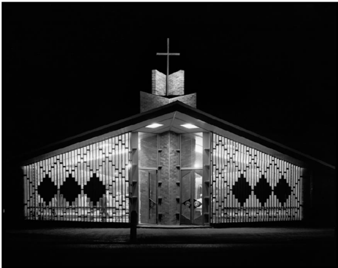
Figure 1: Mareeba Methodist Church (Photograph: Richard Stringer, Sunday 18 August 1968, 7.30pm )
