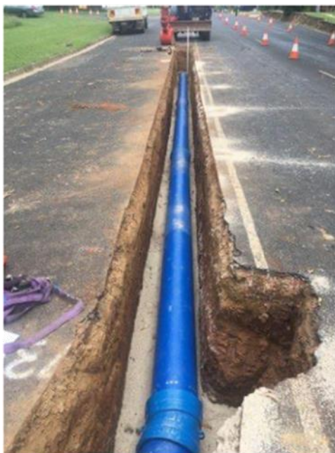
Installation of the new 300mm diameter ductile iron water main
