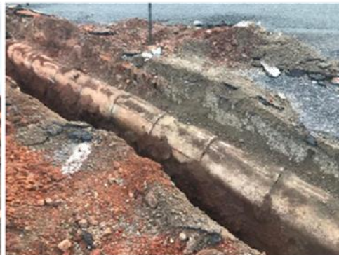
Failing Existing Stormwater System
