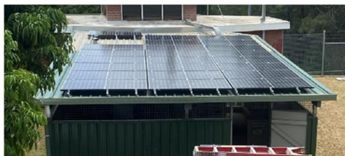
Granite Creek Pump Station
