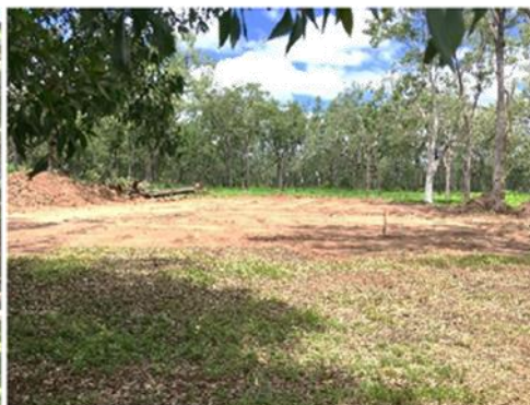
Cleared site for new pound facility
