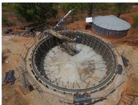
Ring beam formed up in preparation for concreting
