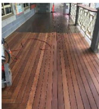
Front Deck Partially Sanded
