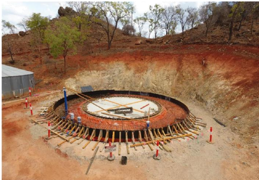
Ring beam formed up in preparation for concreting
