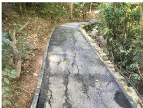
Jum Rum Trail - Pressure Washed Prior to Overlay
