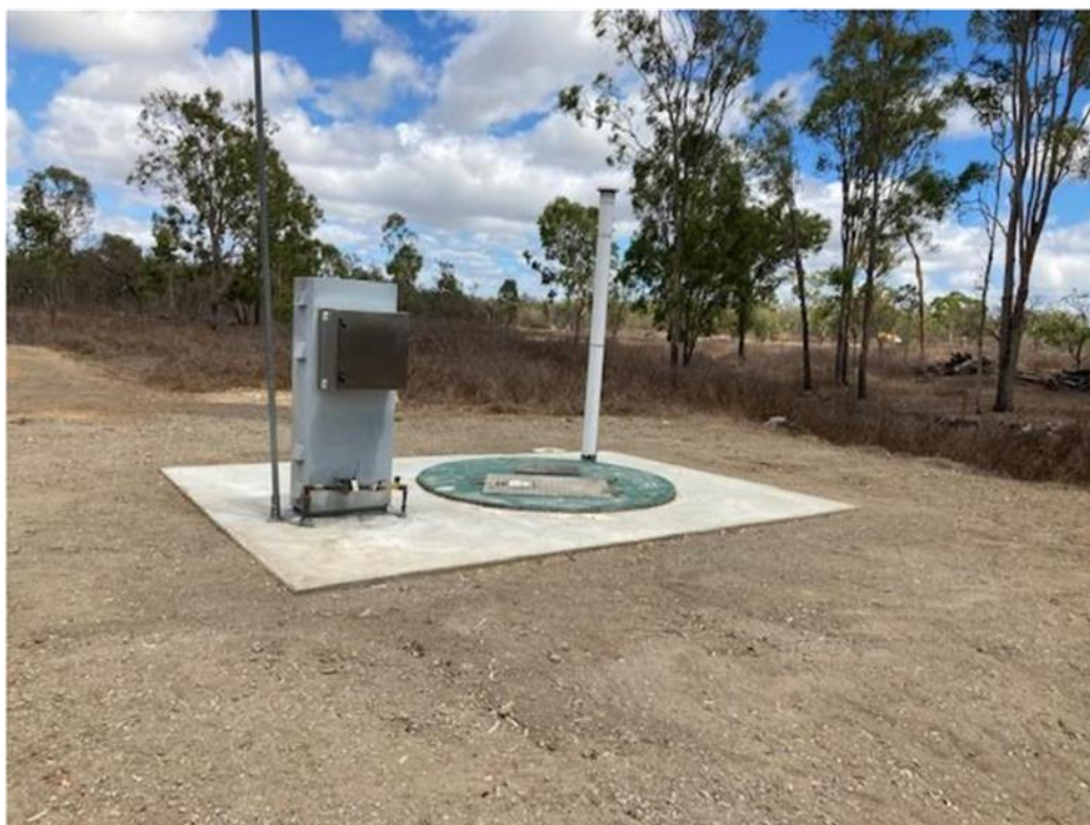
Installation and construction of new cement slab and bypass system at Industrial Park SPS
