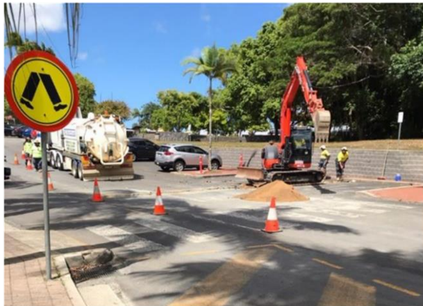
Installation of new water services from the new water main on Rob Veivers Drive
