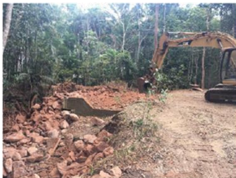
Rock Armouring the Re-shaped Drain
