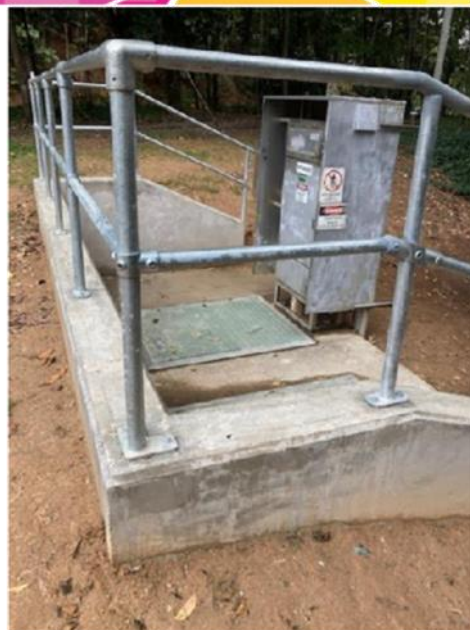
Installation and construction of new access retaining wall at Honey House SPS
