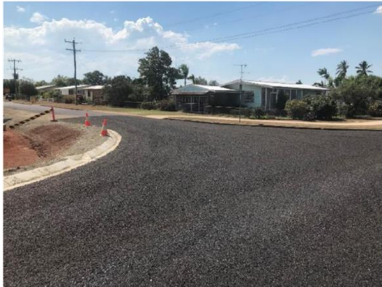
Chewko/Fenwick Streets intersection after 10mm second coat
