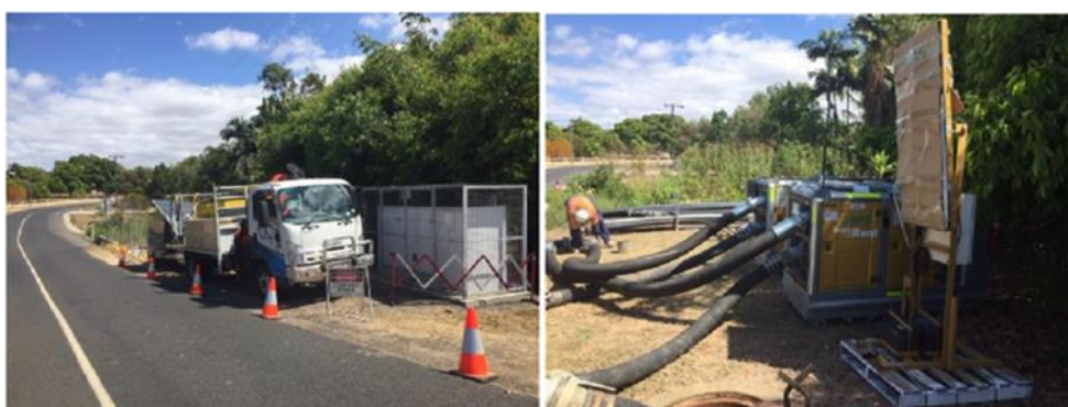
Installation and construction of new bypass system at Kenneally Road SPS
