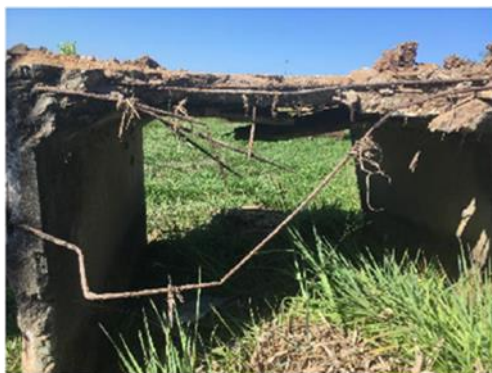
Replaced Existing Box Culvert
