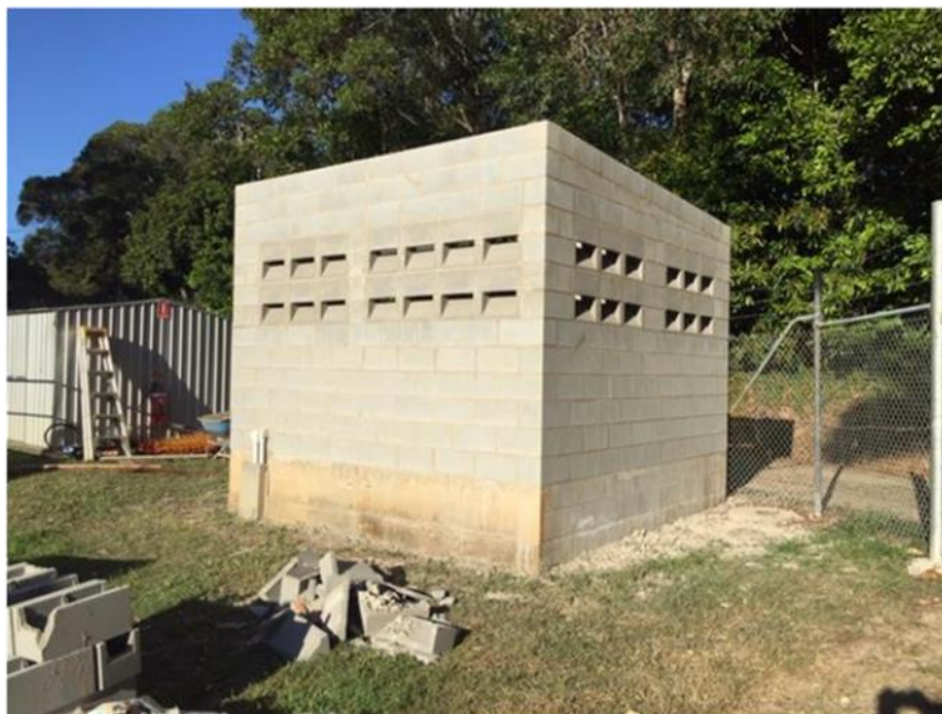
Construction of new SMBS Chemical Storage Shed at Kuranda WWTP
