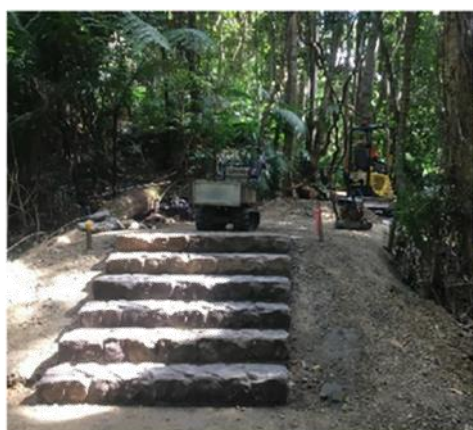
Bridge 7 Approach Steps Under Construction
