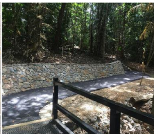
Bridge 10 Batter Protection
