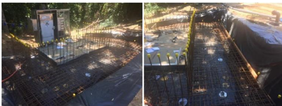
Installation and construction of new access retaining wall at Honey House SPS
