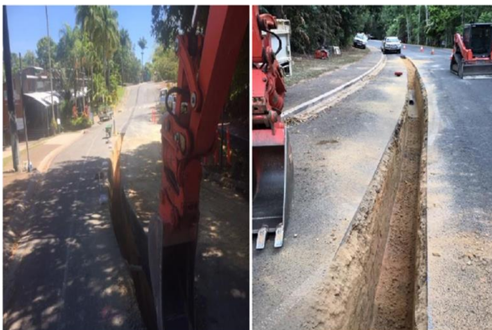
Installation of new water main on Rob Veivers Drive prior to backfilling
