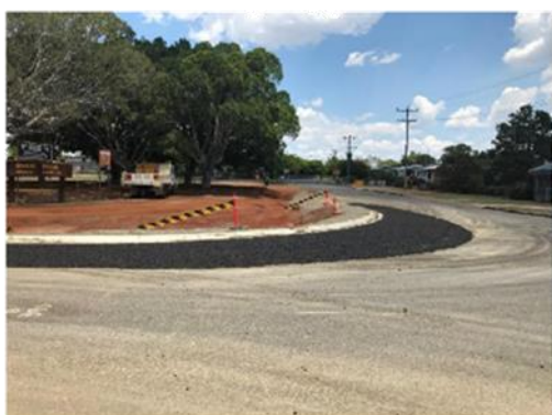
Chewko/Fenwick Streets intersection prior to 10mm second coat
