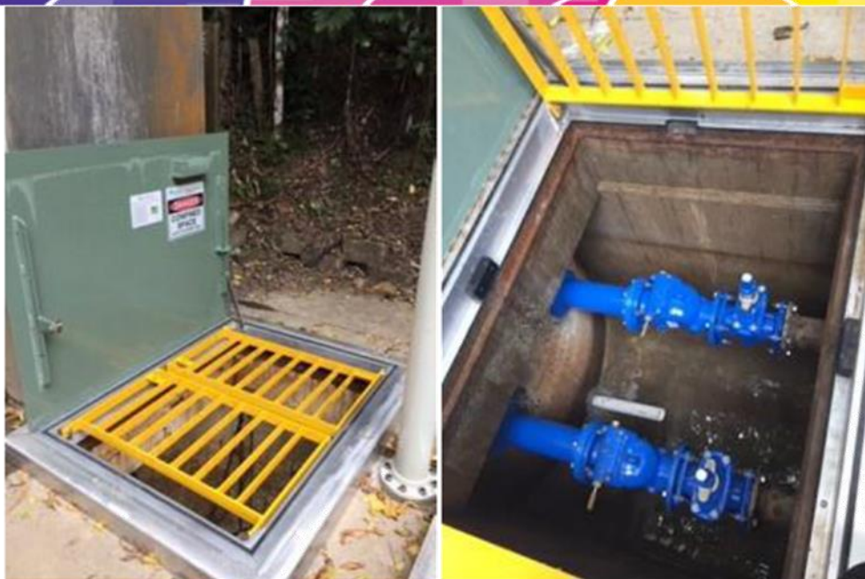
Installation of new access lids and valve and piping at Kullaroo SPS
