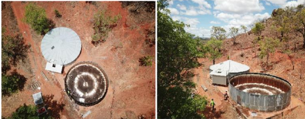
Demolition of the existing No 2 Reservoir
