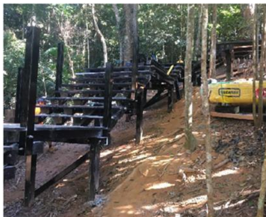
Bridge 11 Stair Approach Under Construction
