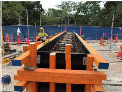
Pier 2 Reinforcing and Formwork
