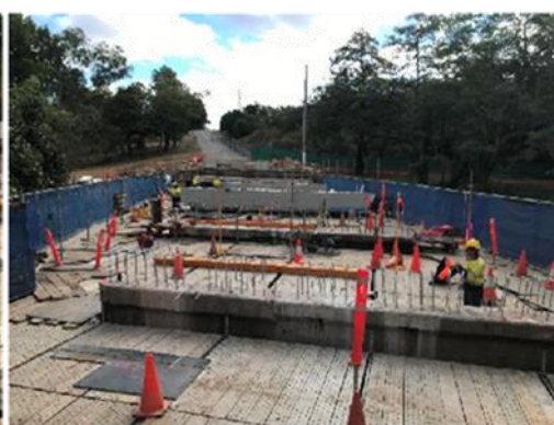
Installing Reinforcement Pier 3 and 4
