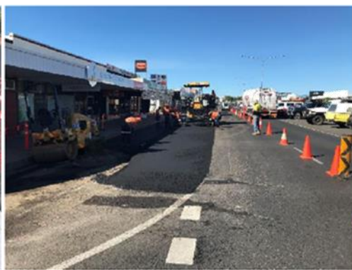
Section 6 - Asphalt Sealing
