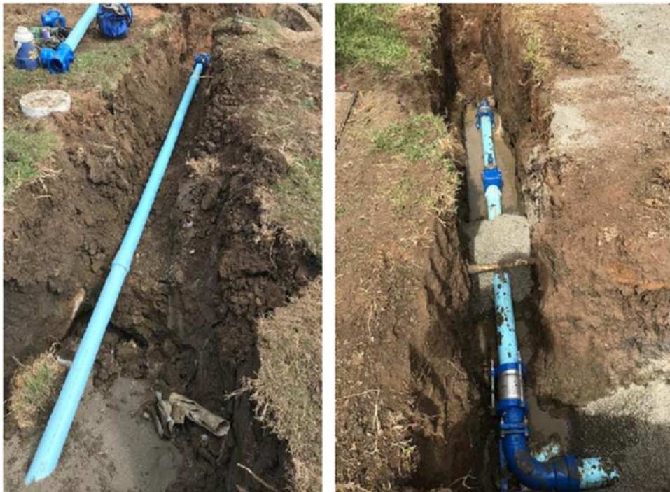
Installation of new water main on Costin Street prior to backfilling
