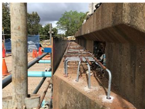
Abutment 1 Reinforcing
