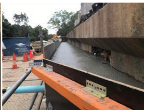
Abutment 1 After Pouring
