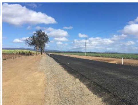
Chainage. 0.2km (after)
