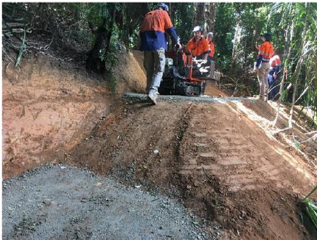
Transporting prefabricated stair units
