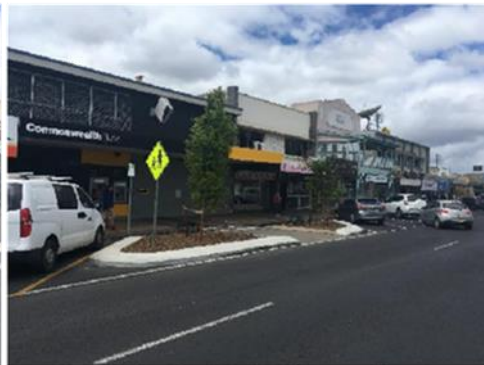
Completed work - C'bank Pedestrian Refuge
