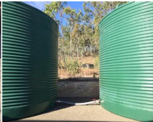
New water storage tanks
