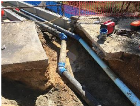
Water and Sewerage Services - Eastern Side
