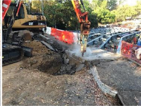
Preparing Relieving Slab for Services - Eastern Side
