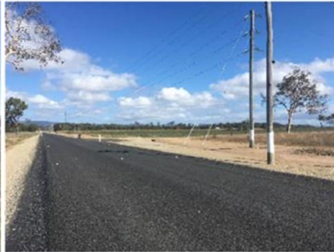
Chainage. 1.2km (after)
