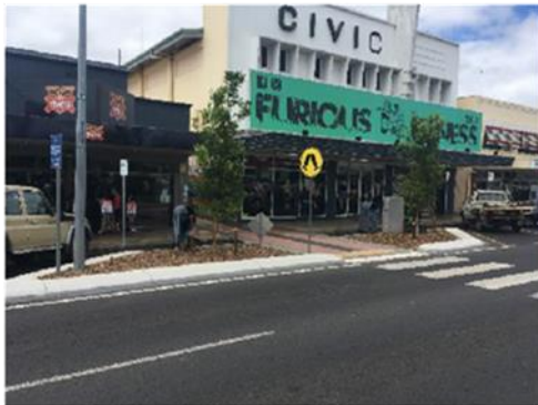
Completed work - Post Office Pedestrian Crossing
