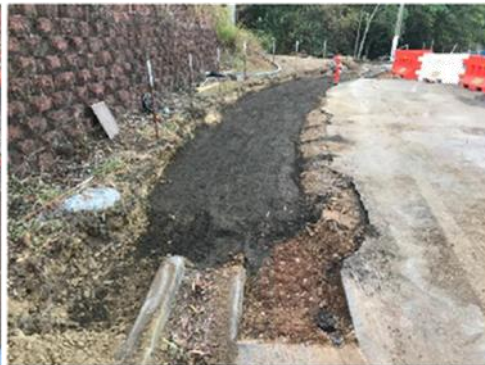
Prepared base for Kerb and Channel - Eastern Side
