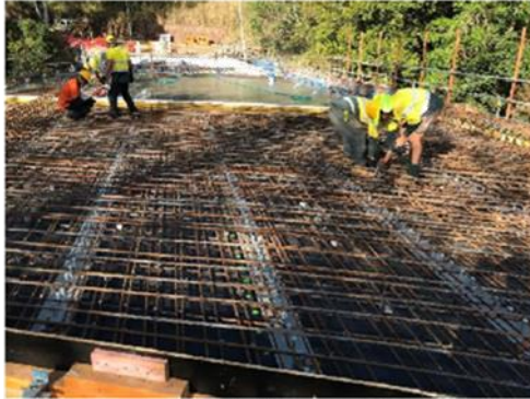
Installing Reinforcement - Span 1
