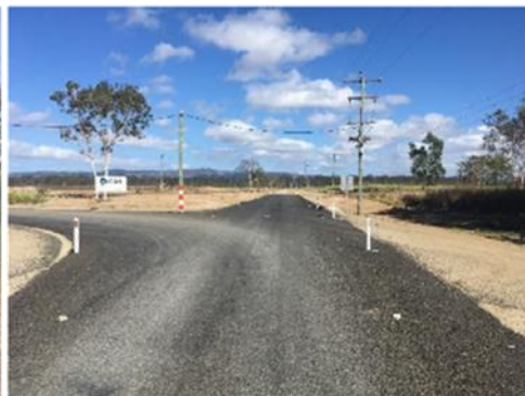
Chainage. 2.1km (after)
