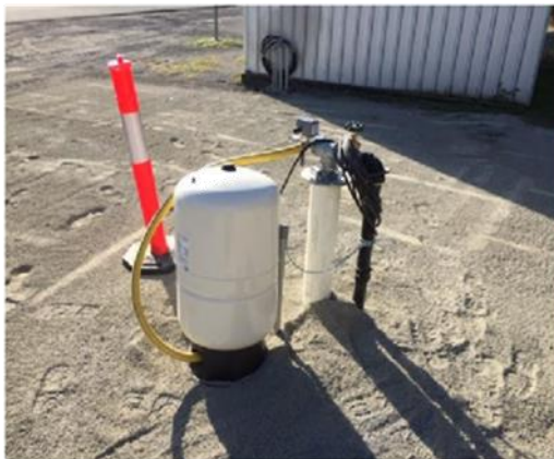
Newly installed bore
