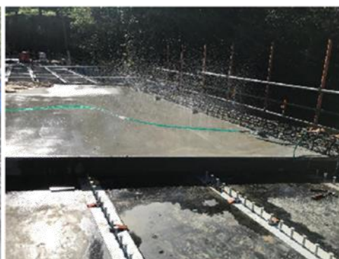
Span 2 Moist Curing
