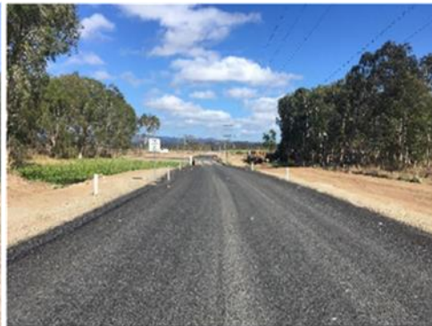
Chainage. 1.8km (after)
