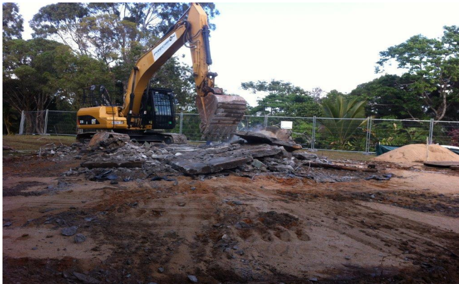
Hilltop Close Water Reservoir Demolition works
