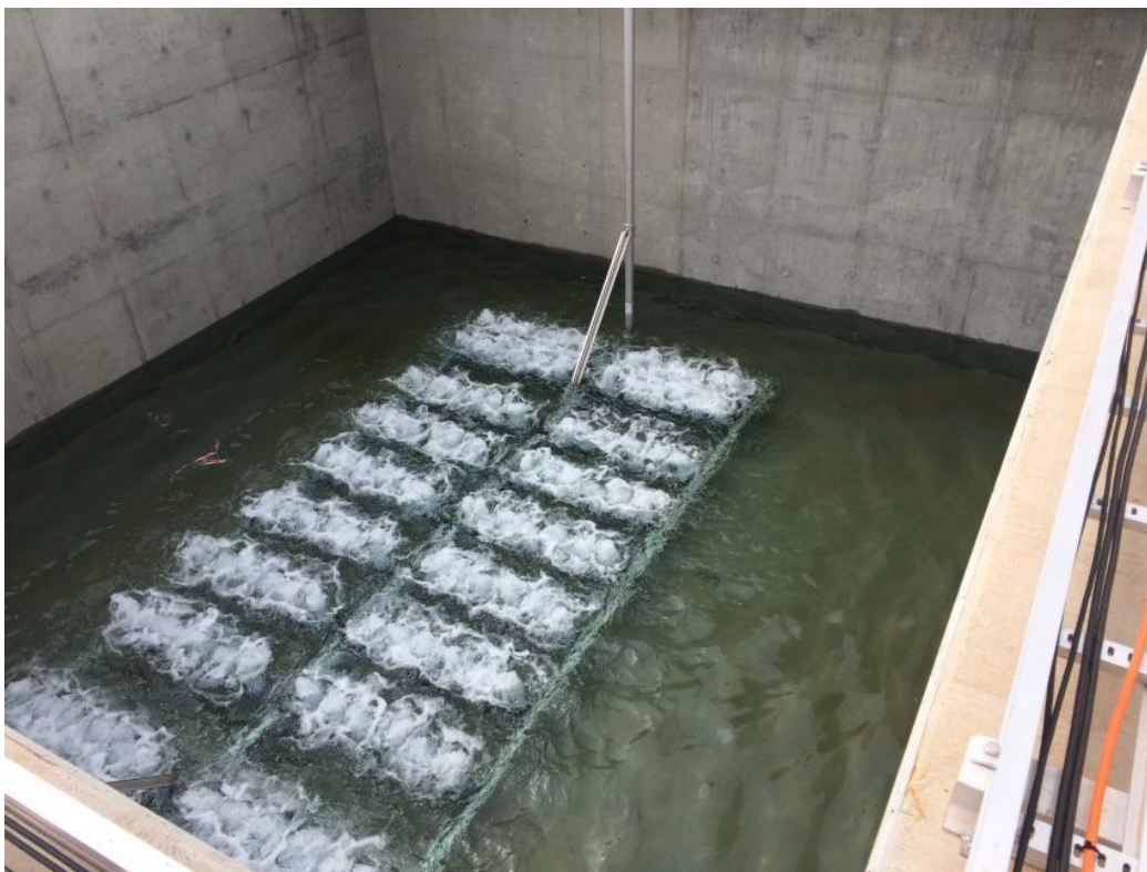
15 June 2017 - Bubble-testing the diffusers in the digesters successfully completed
