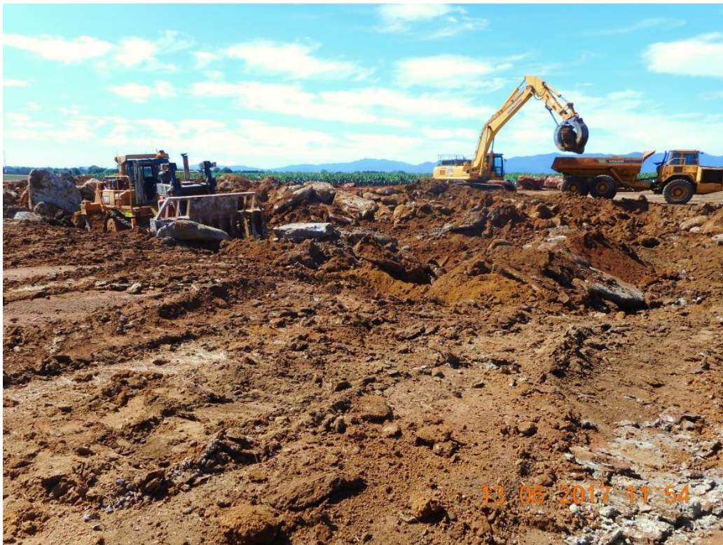
13 June 2017 - Excavation of rock for roads in aviation commercial precinct
