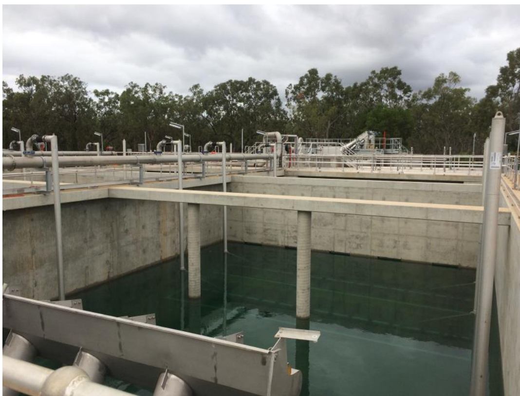
23 June 2017 - Hydrostatic testing of basins to sequential batch reactor (SBR)
