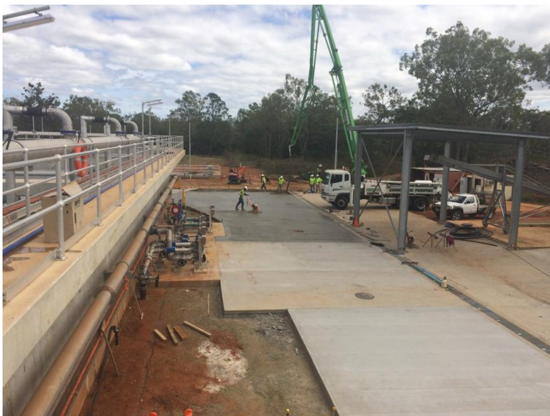
20 June 2017 - Construction of concrete site roads
