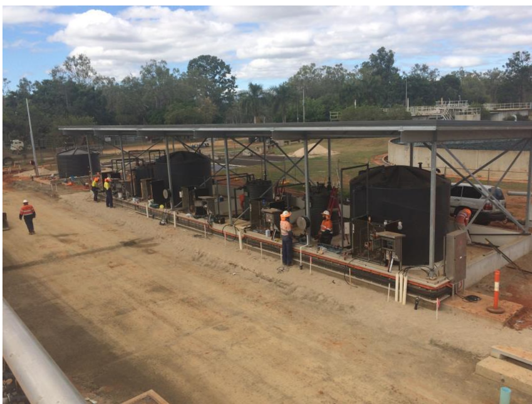
20 June 2017 - Electrical cabling to chemical dosing area
