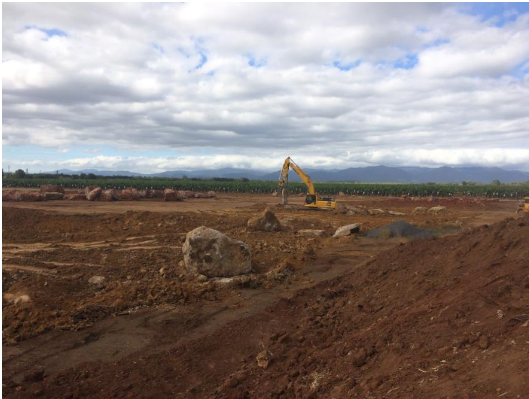
20 June 2017 - Large rocks are set aside for rockbreaking prior to transporting to stockpile.
