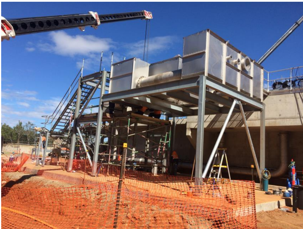
6 June 2017 - Mechanical installation for inlet works by Aqseptence Group
