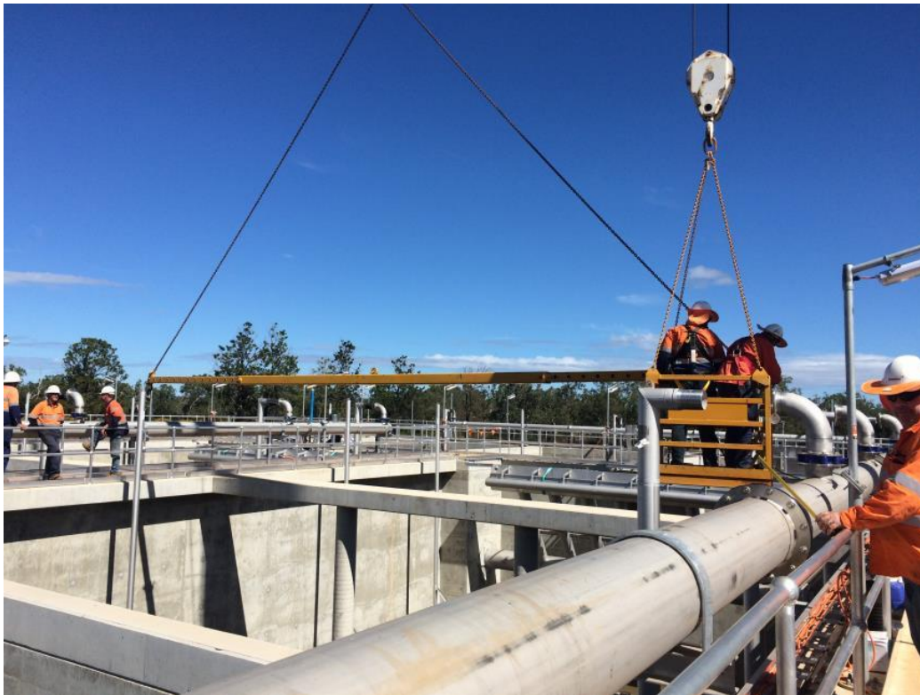
6 June 2017 - Trial-lift of diffusers in sequential batch reactor (SBR)
