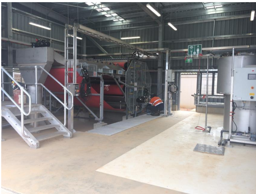
20 June 2017 - Connection of compressed air lines to sludge dewatering press in preparation for commissioning
