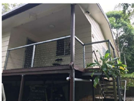
Unit 2E - After Deck Refurbishment
