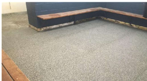
New Flooring, mid installation
