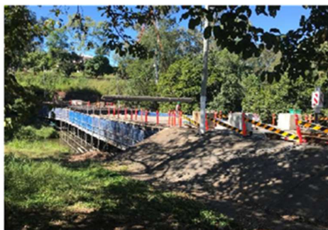
Removing Steel Beams, Steel Deck and Asphalt
