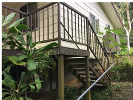
Unit 2E - Before Deck Refurbishment
