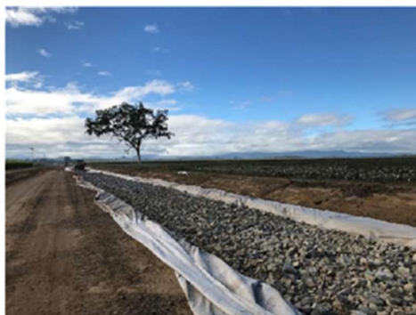
Unsuitable Subgrade Treatment
