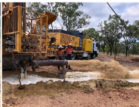
Bore drilled at location 3km west of Chillagoe
