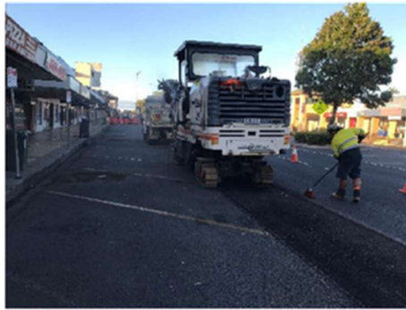
Section 2 - Pavement Milling
