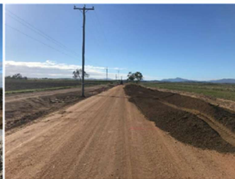
Imported Type 2.4 Subbase
