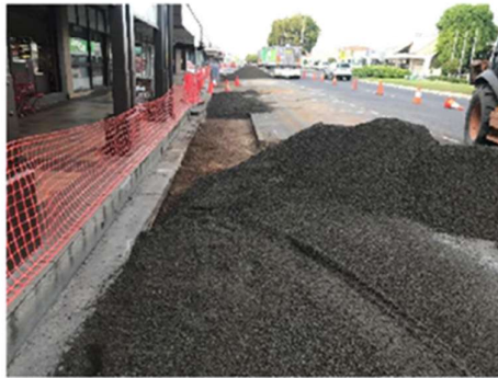
Section 3 - Cement-treated gravel placement
