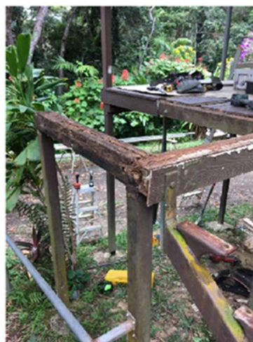
Unit 2E - During Deck Refurbishment
