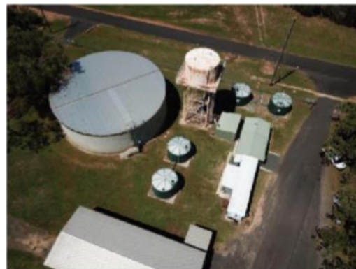
Aerial view of Dimbulah Water Treatment Plant
