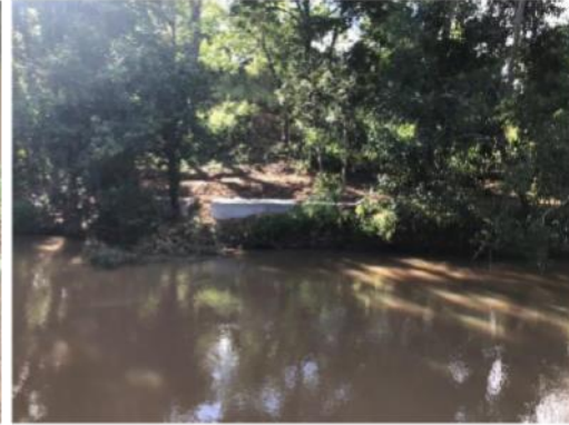
Temporary Pedestrian Bridge Footings
