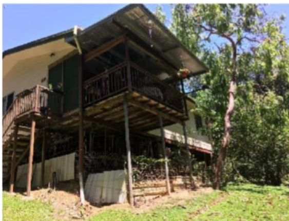
Unit 2D - Before - Deck Refurbishment
