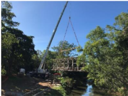
Temporary Pedestrian Bridge Placement
