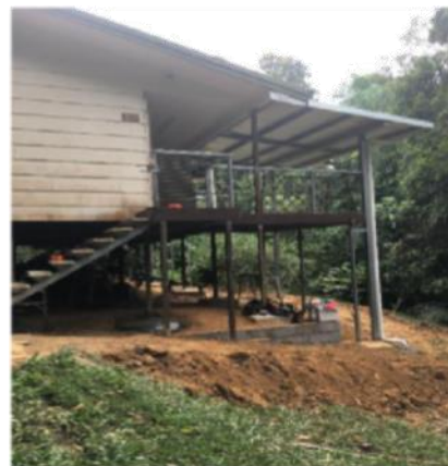
Unit 2D - In-process - Deck Refurbishment
