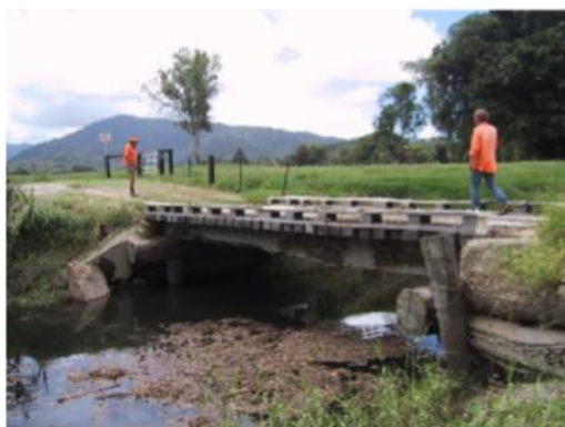
Chapmans Road Bridge prior to commencement
