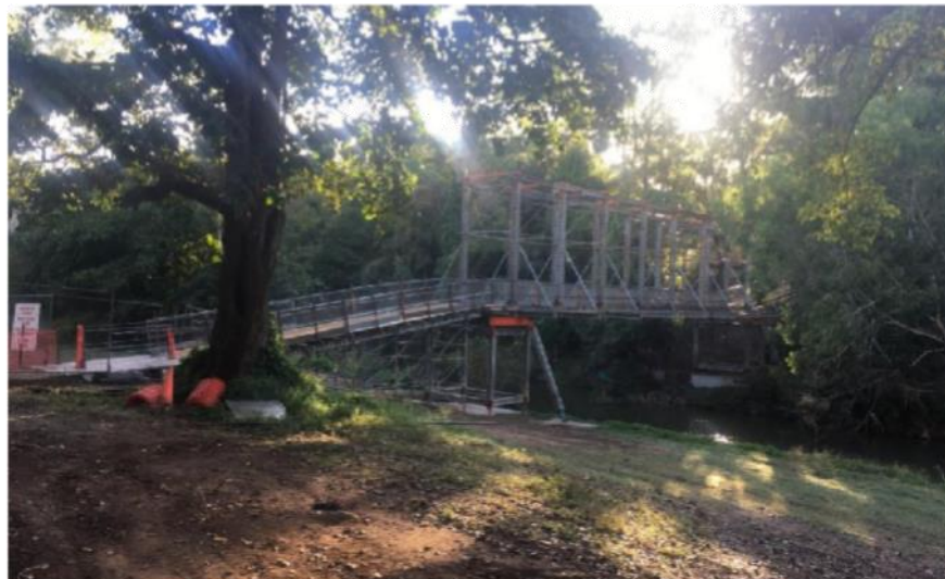
Temporary Pedestrian Bridge
