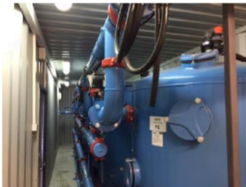
Filters at Dimbulah Water Treatment Plant
