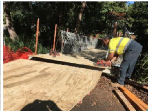
Temporary Pedestrian Bridge Finishing
