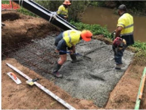
Temporary Pedestrian Bridge Footings
