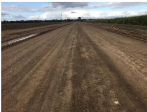
Section of road at subgrade level
