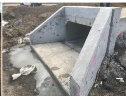
New Culvert Installation
