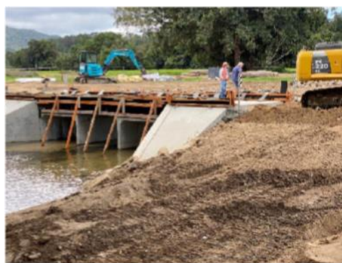
Replacement box culvert structure under construction
