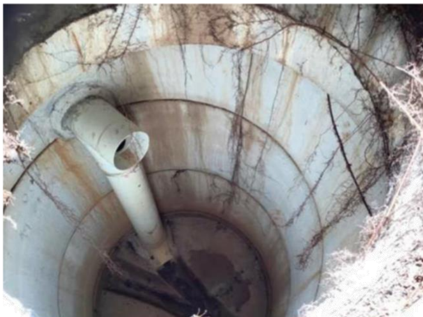
Example of Tree roots entering pump station due to defects: Arara Street, Kuranda
