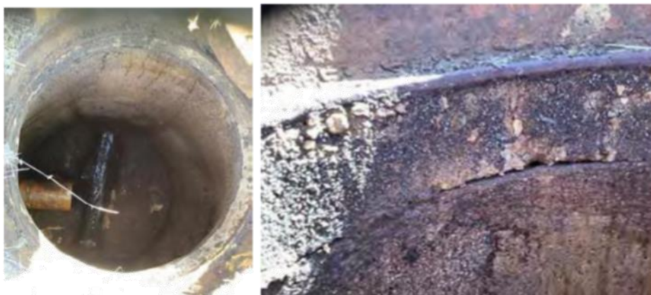
Example of Manhole to be rehabilitated in Palm Close, Mareeba
