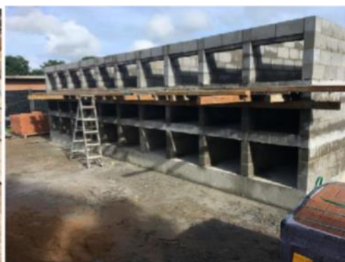
Masonry block wall construction
