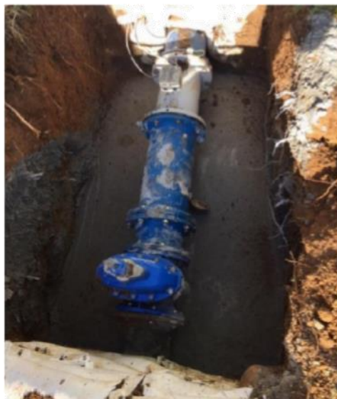
New connection for bulk flow meter installation
