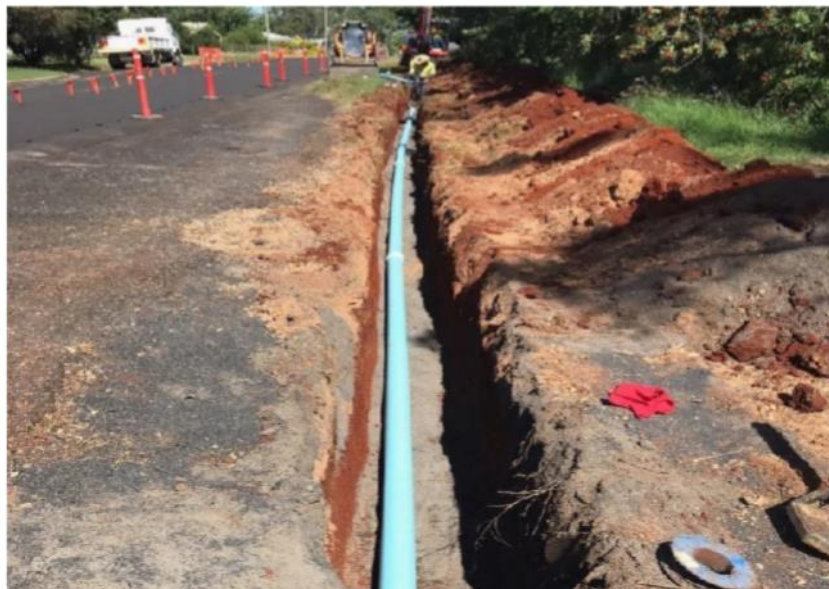
Installation of new water main on Costin Street prior to backfilling
