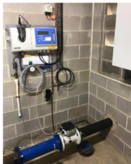
Newly installed bulk water flow meter at Mason Rd
