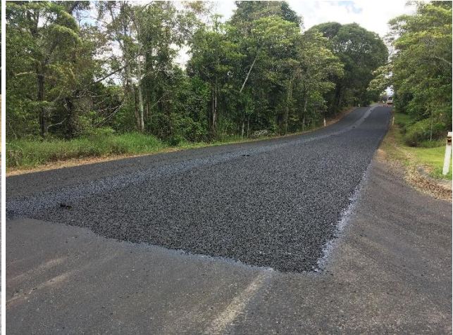
Euluma Creek Road - Before and After Reseal
