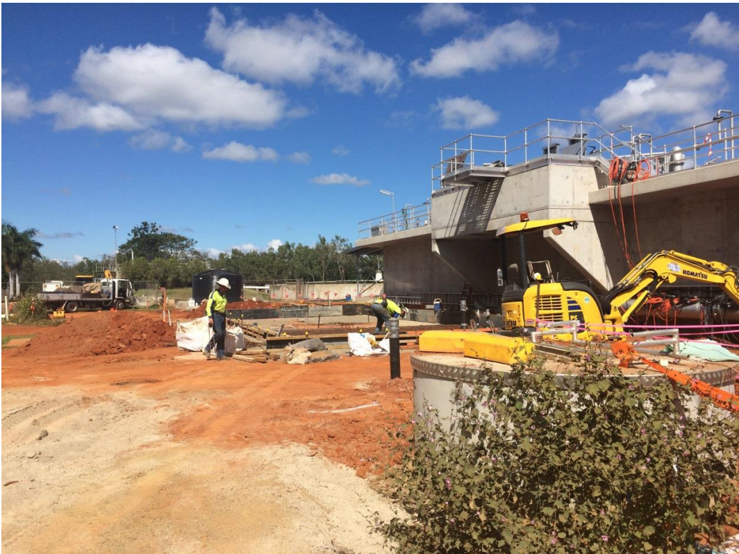
10 May 2017 - Commencement of slab for inlet works
