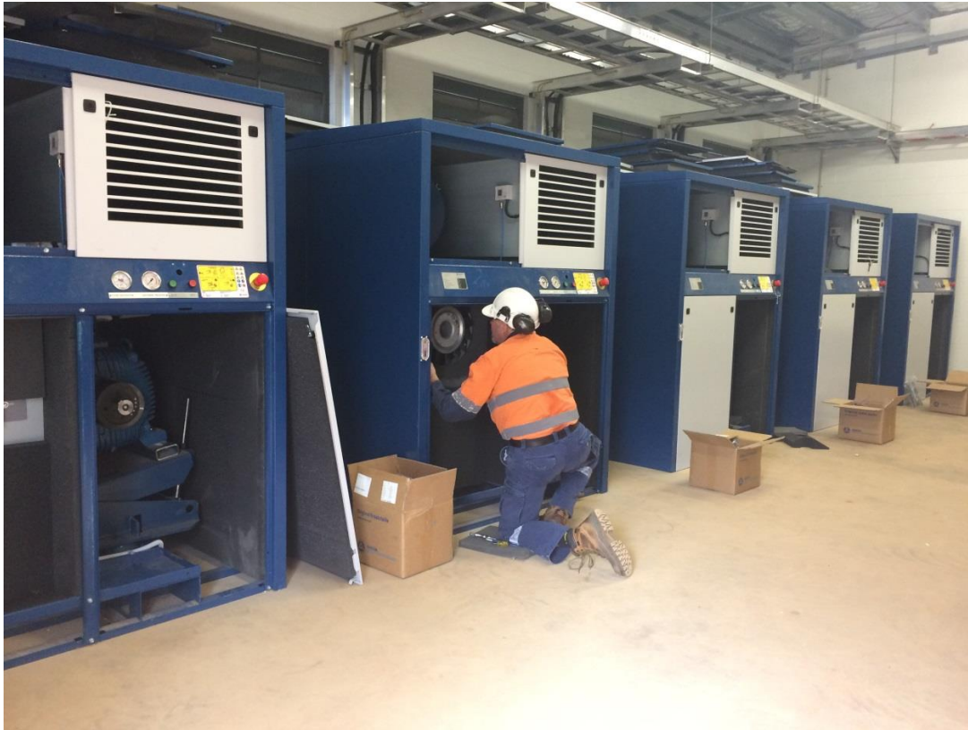
24 May 2017 - Aeration blowers powered-up and run-in
