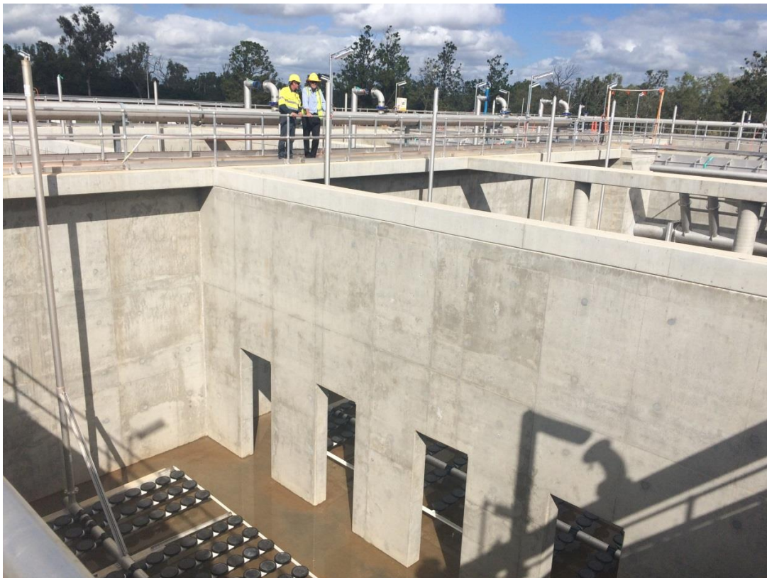
26 May 2017 - Council's Water & Wastewater Engineer and treatment plant operator inspect the recently installed diffusers
