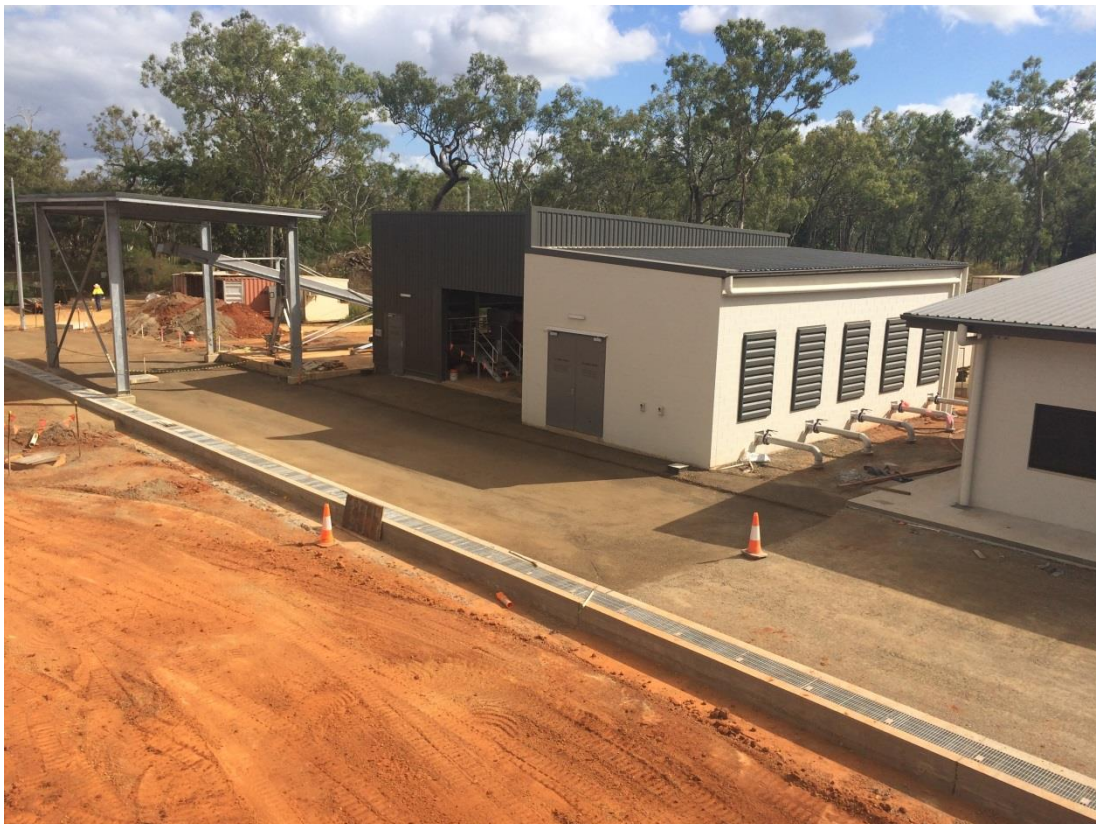
26 May 2017 - Sub-base prepared ready for construction of concrete road in front of sludge dewatering building, blower building and administration building
