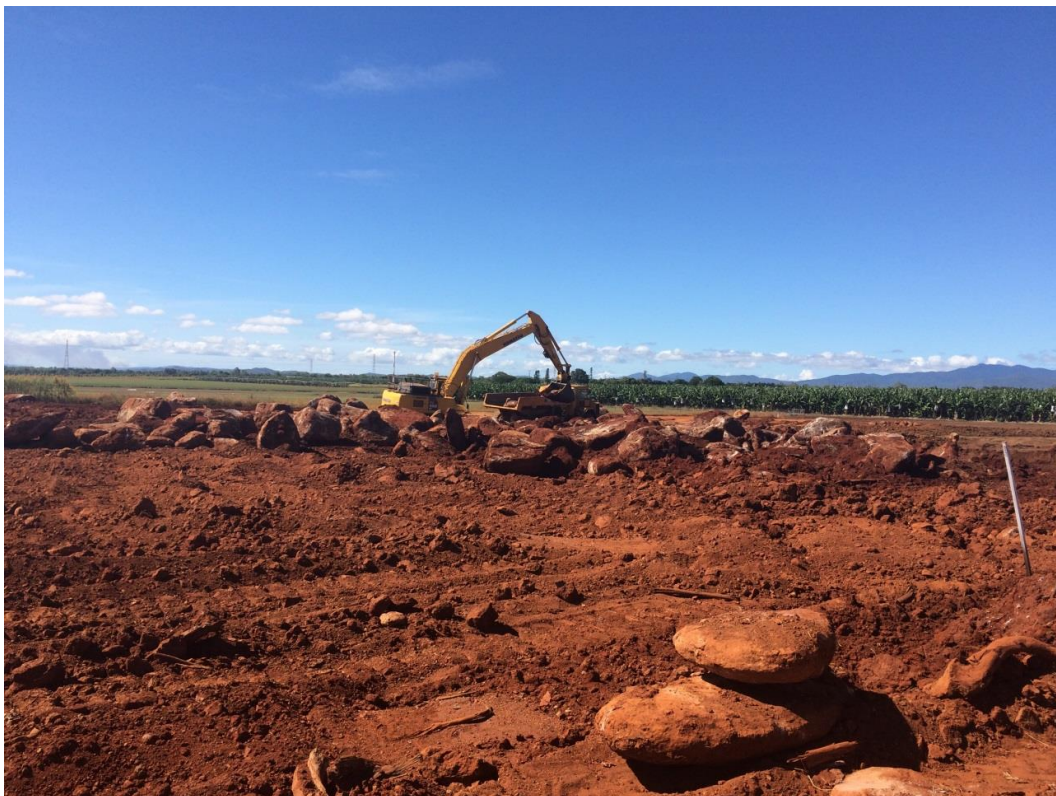
16 May 2017 - Excavation of rock for aviation commercial precinct
