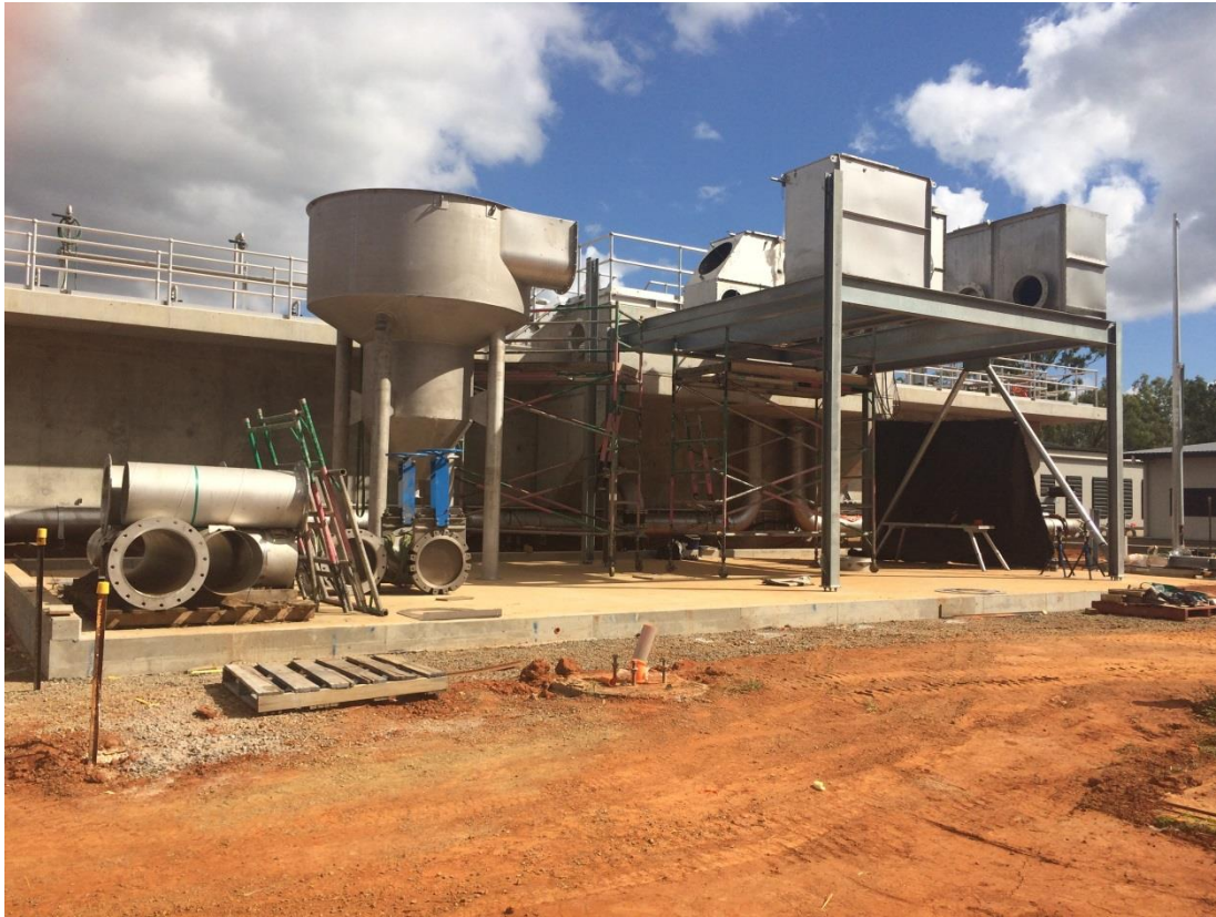
26 May 2017 - Installation of the packaged inlet works underway
