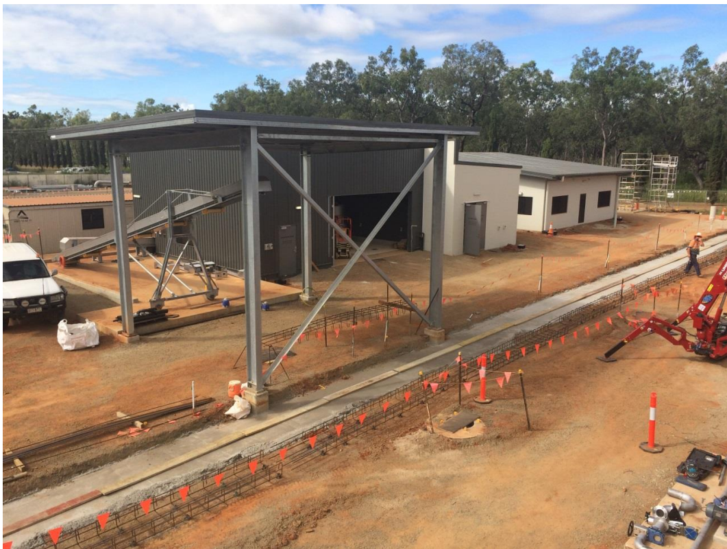
4 May 2017 - Commencement of road drainage works
