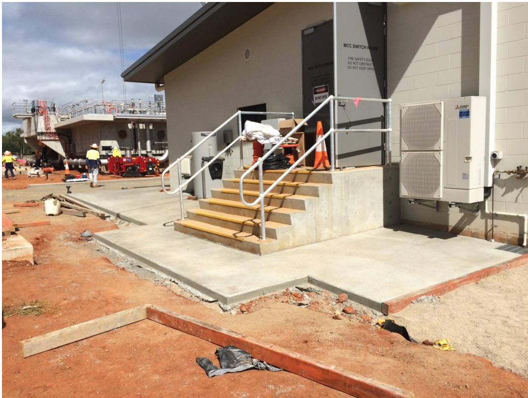
23 May 2017 - Concrete pathway constructed to Control Room
