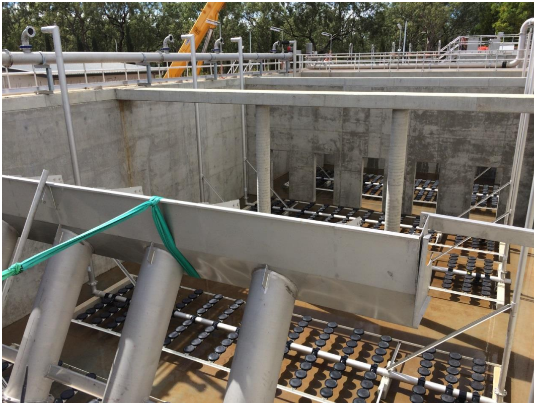
23 May 2017 - Diffusers installed to sequential batch reactor (SBR)
