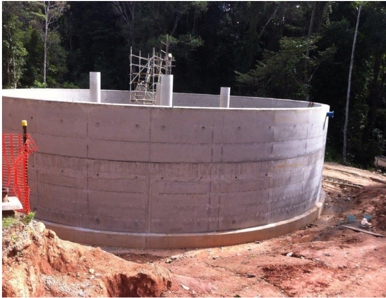
Platypus Close Water Reservoir Construction
