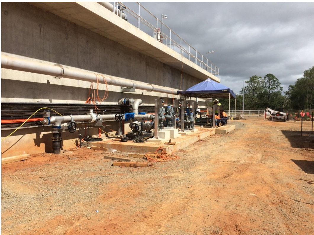
23 May 2017 - Installation of pumps for return activated sludge (RAS) and waste activated sludge (WAS)
