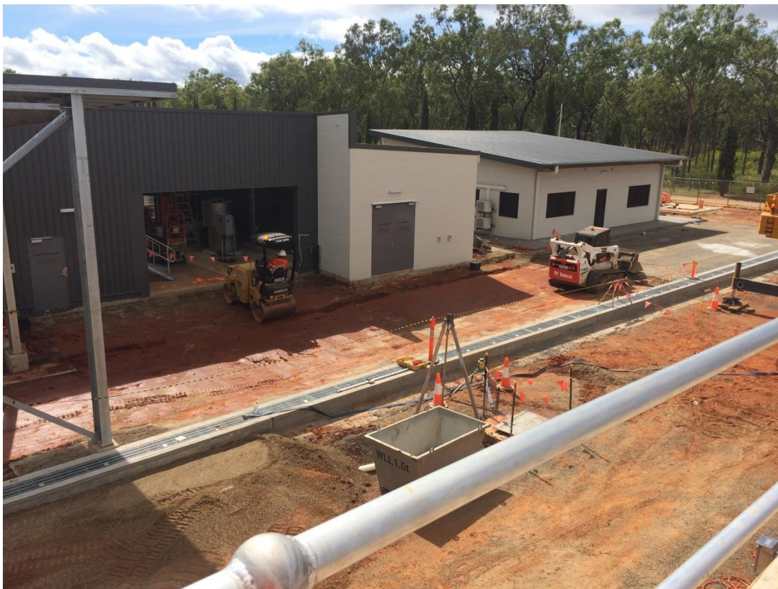
23 May 2017 - Construction of site roads
