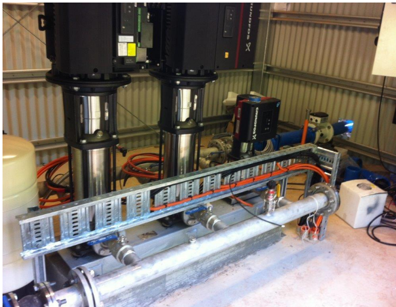
New water pressure pump shed and pressure pumps Warril Drive
