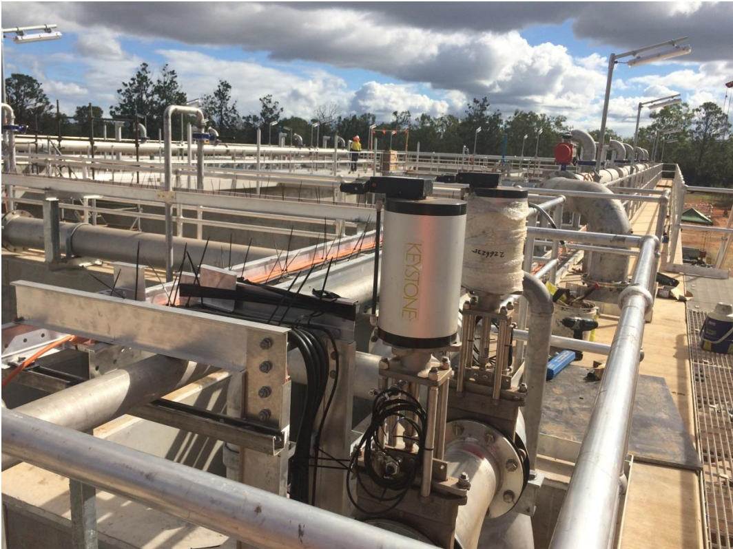
4 May 2017 - Mechanical equipment, pipework, handrails and lighting installed to sequential batch reactor (SBR)
