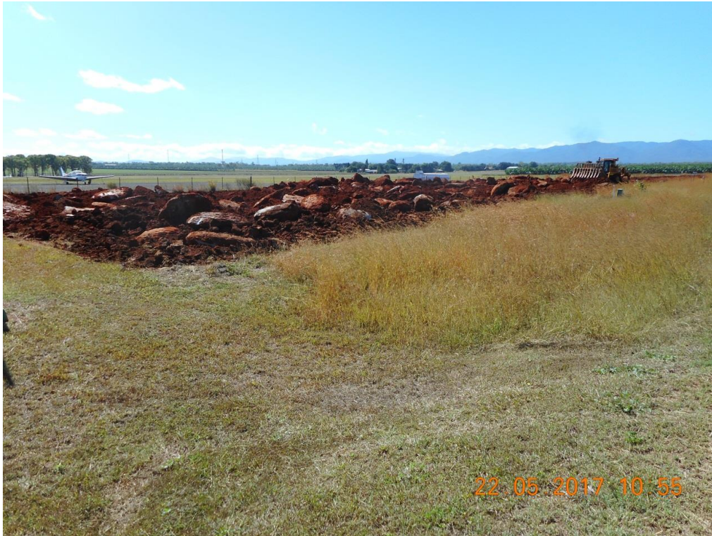
22 May 2017 - Excavation of rock for leases and taxilanes adjacent existing western apron
