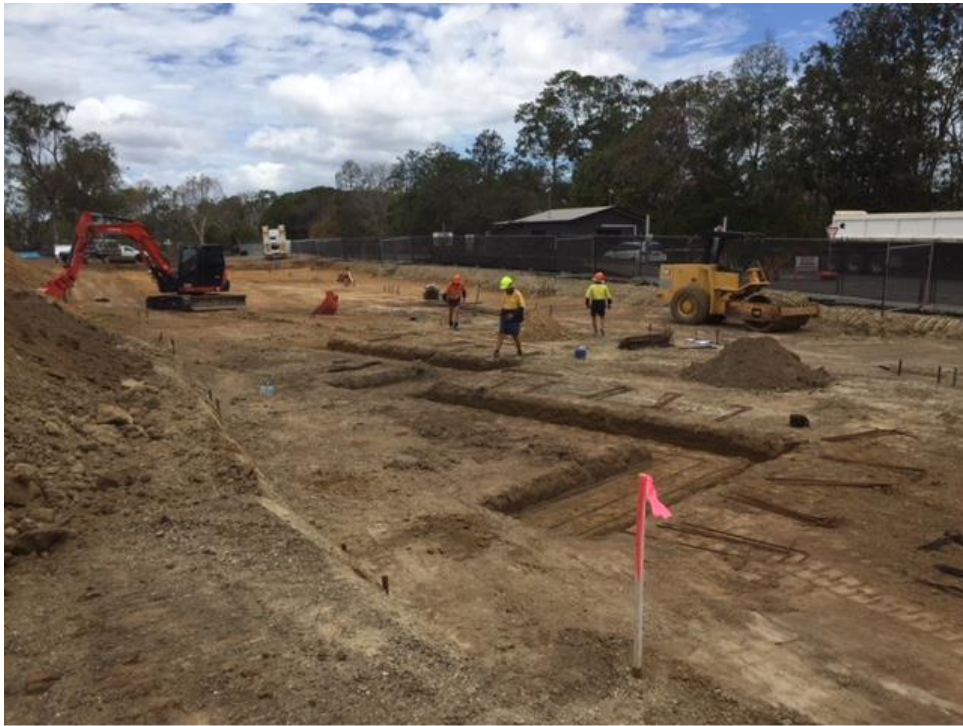
Figure 1 Mareeba Waste Transfer Station Upgrade east view
