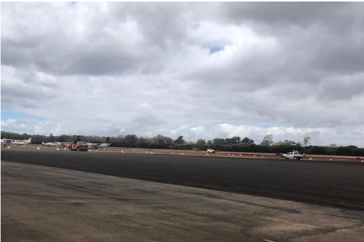
23 September 2019 - Sealing of Eastern Apron and Taxiway.
