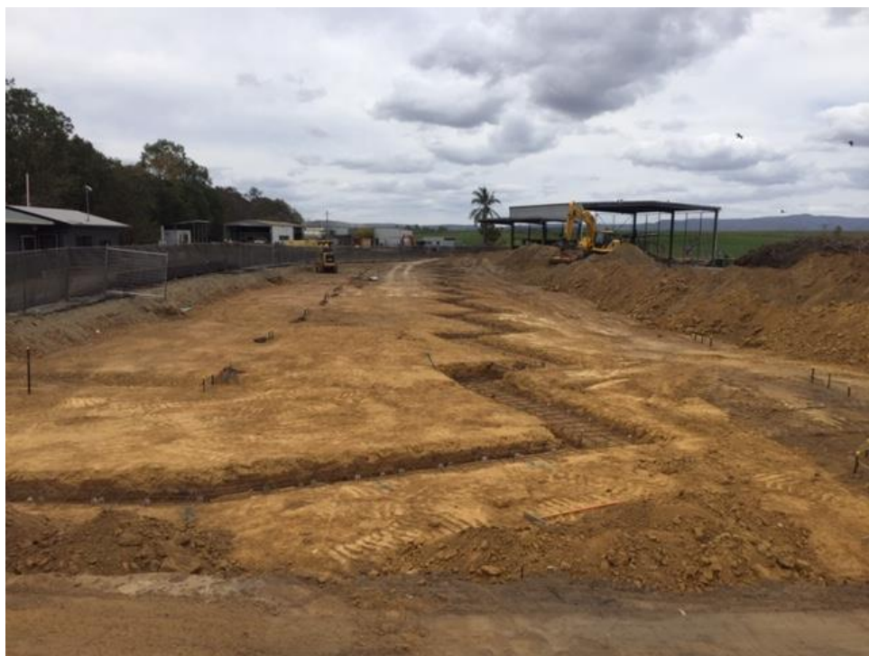
Figure 2 Mareeba Waste Transfer Station Upgrade west view
