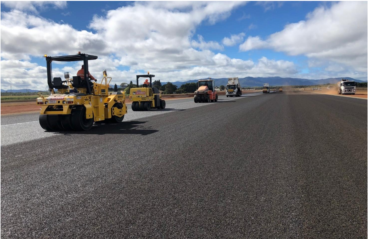
8 July 2019 - Sealing Western Section of Runway
