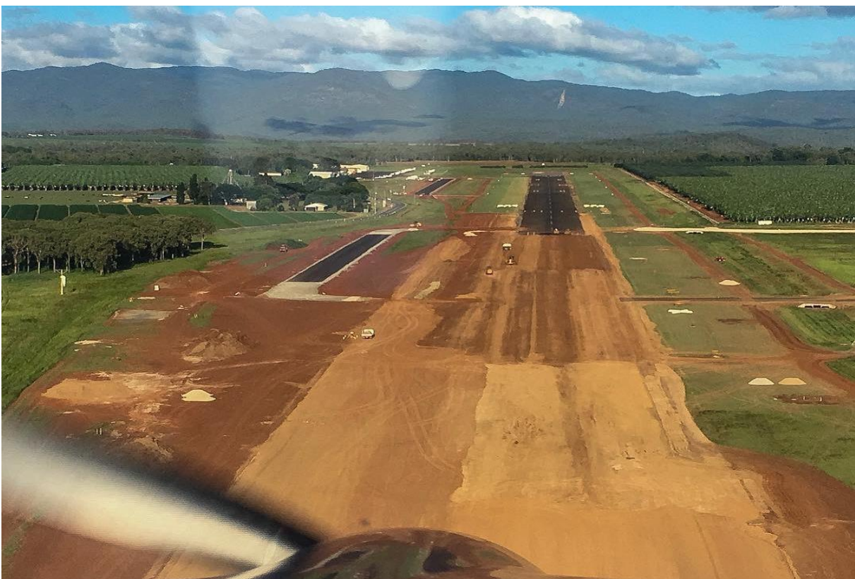
15 April 2019 - Aerial photograph of construction showing western runway strengthening and extension in foreground and construction of parallel taxiways
