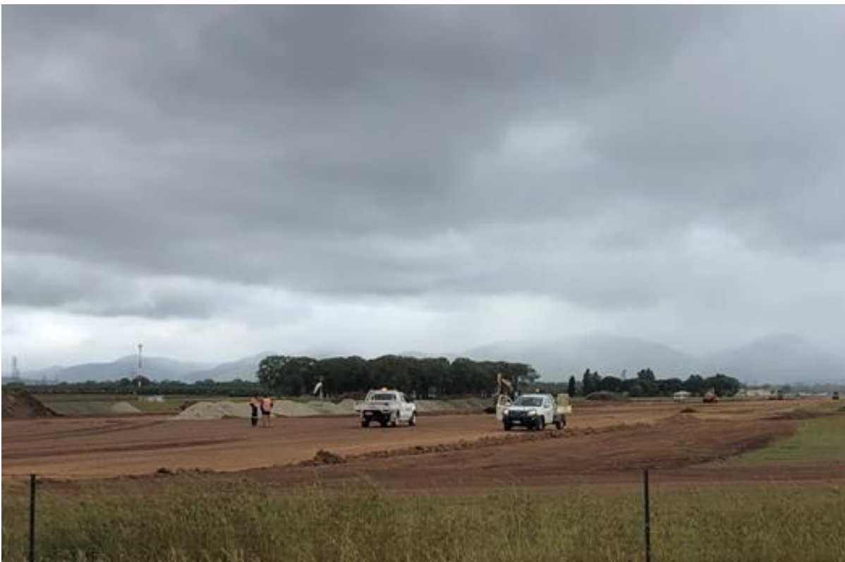
30 April 2019 - Works underway for western runway extension
