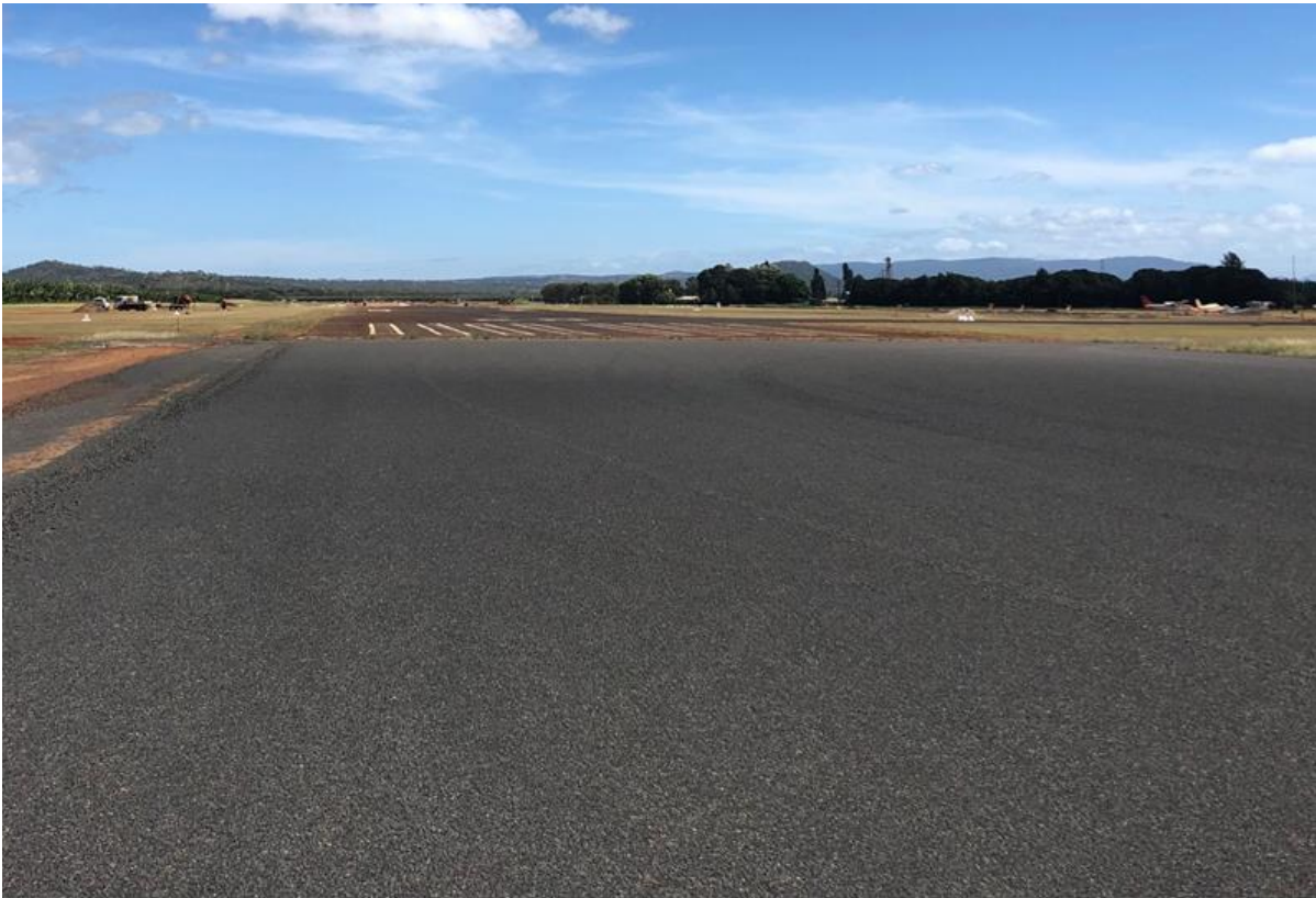
26 April 2019 - Sub-base course constructed for eastern runway extension
