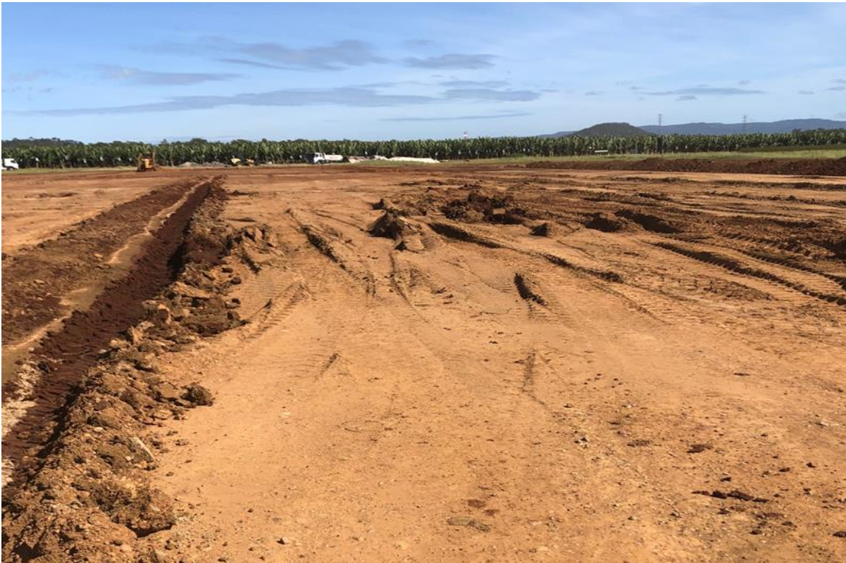
11 April 2019 - Unsuitable subgrade material encountered at western end of runway extension
