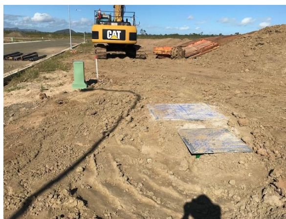
Backfilling of pump station completed
