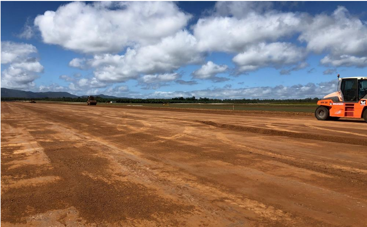
2 May 2019 - Subgrade preparation for strengthening of existing runway (western section)
