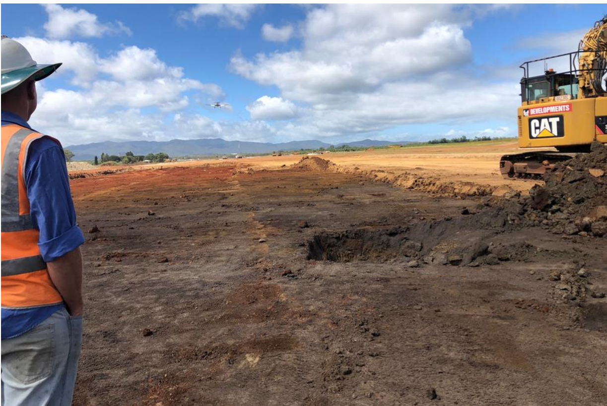
2 May 2019 - Further unsuitable material exposed at western runway extension
