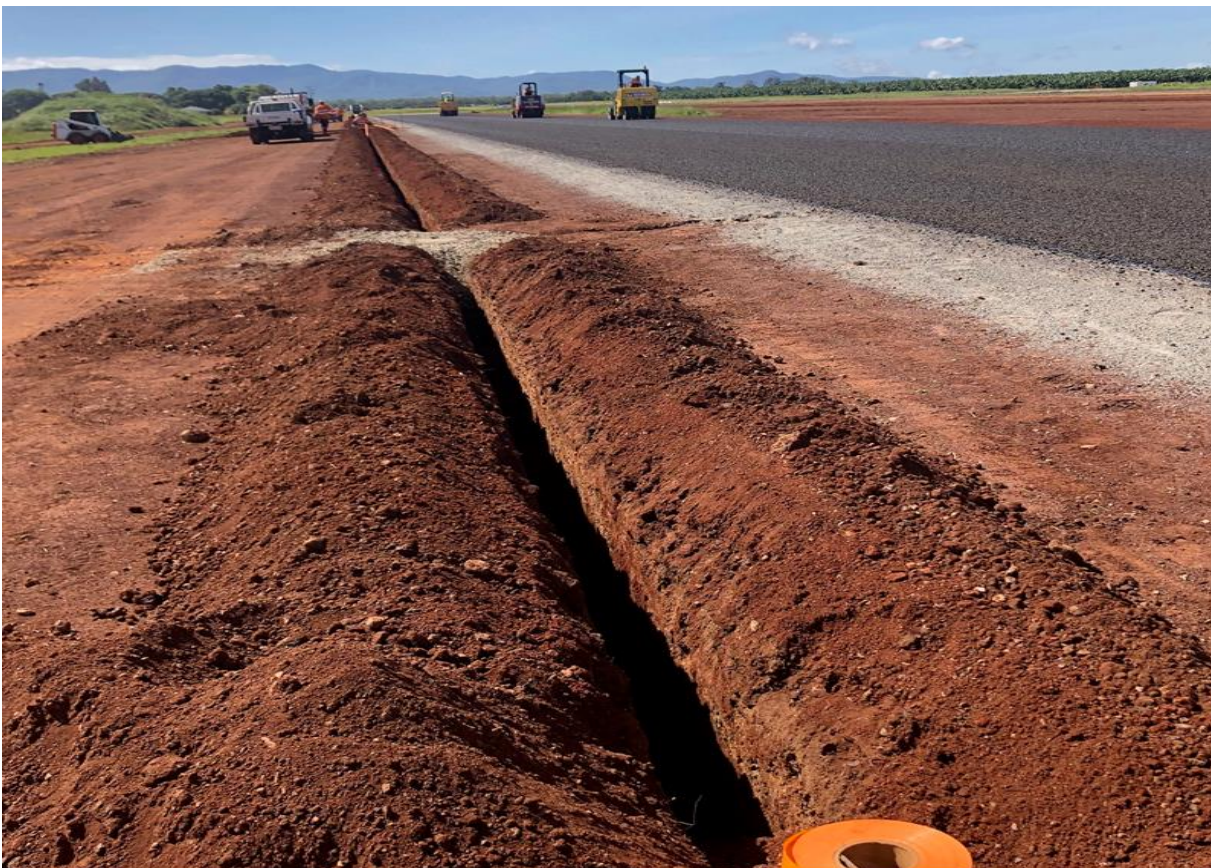
11 April 2019 - Installation of conduit for lighting and bitumen seal for new Taxiway C
