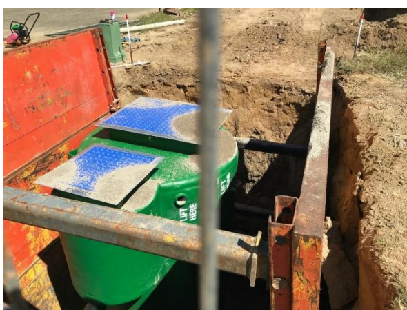
Pump station prior to backfilling
