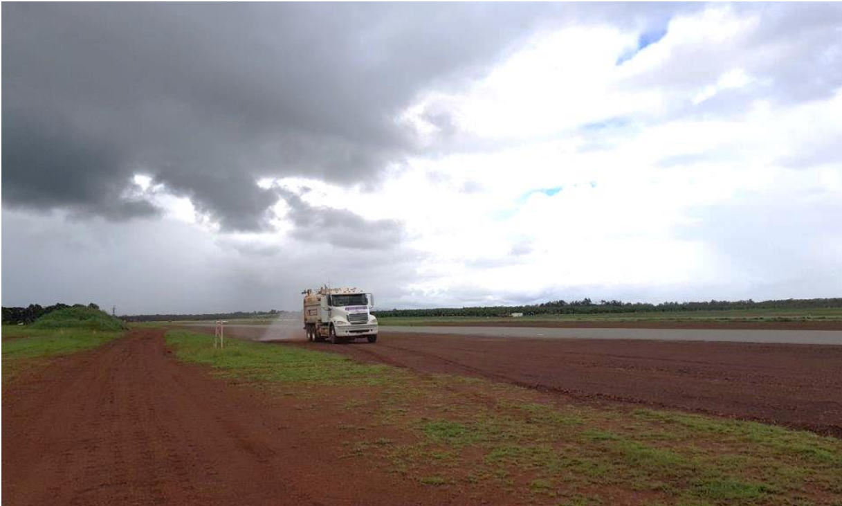
1 April 2019 - construction base course for new Taxiway C
