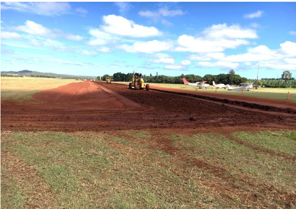
7 March 2019 - Subgrade preparation for parallel taxiway
