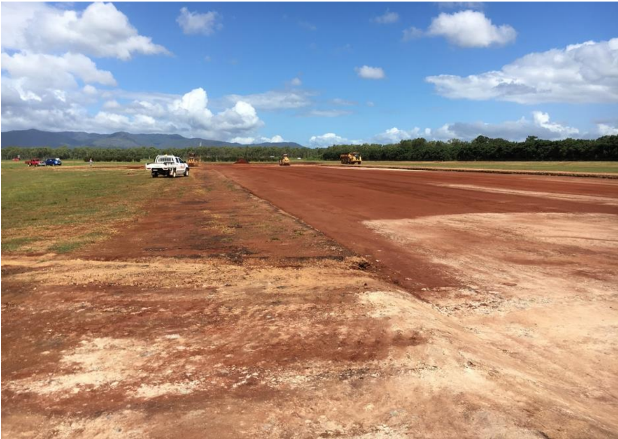
1 March 2019 - Subgrade preparation for eastern runway extension
