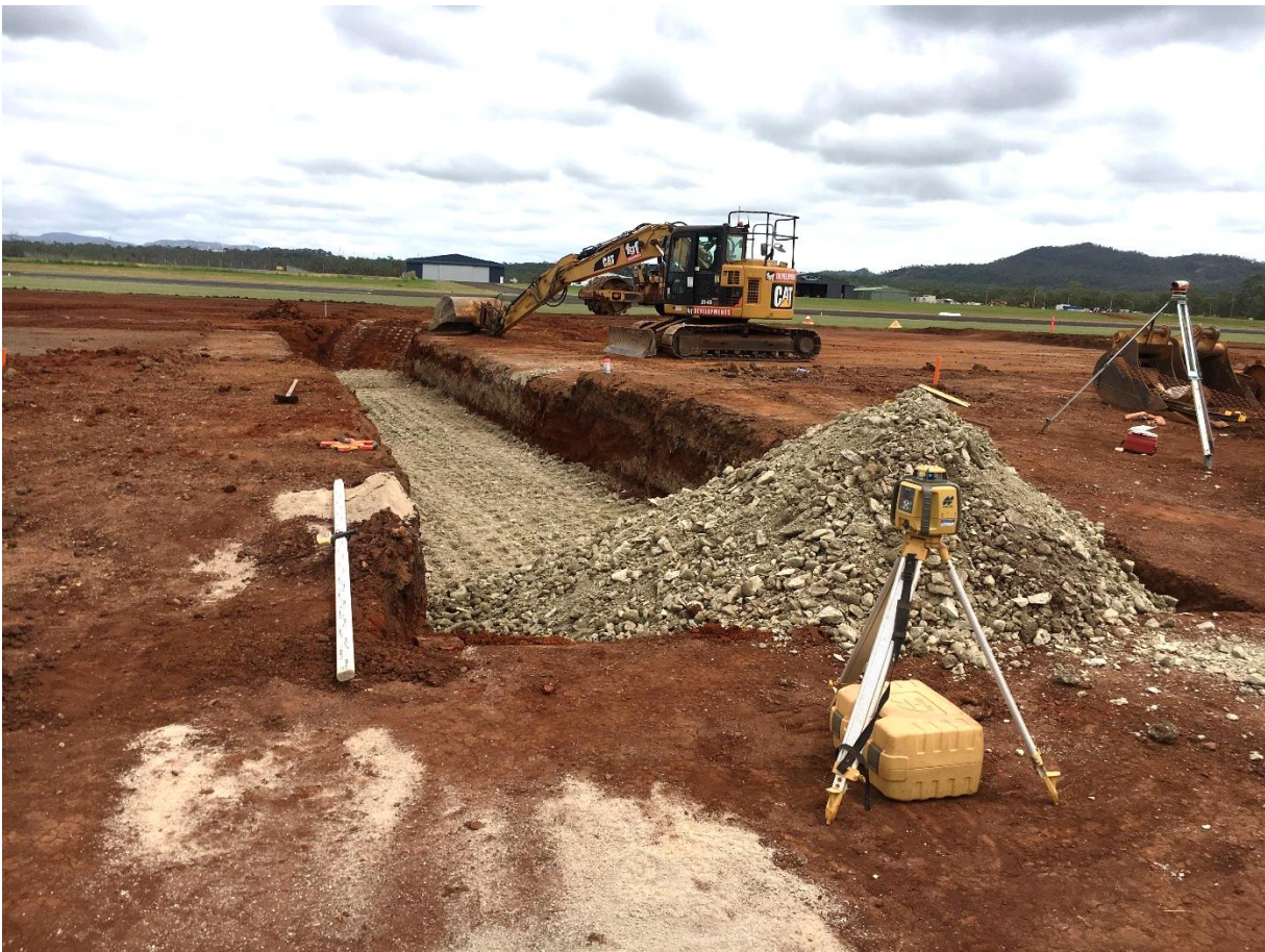
15 March 2019 - Preparation of culvert base for new taxiway
