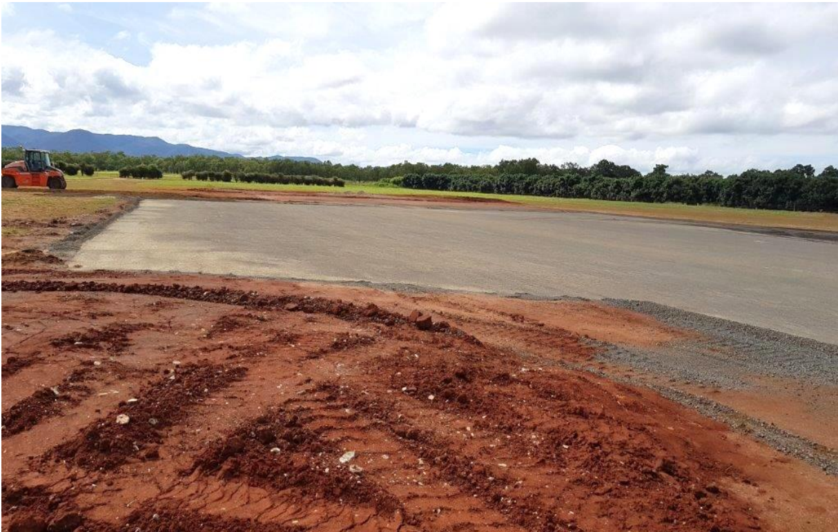
15 March 2019 - Base course prepared for eastern runway extension
