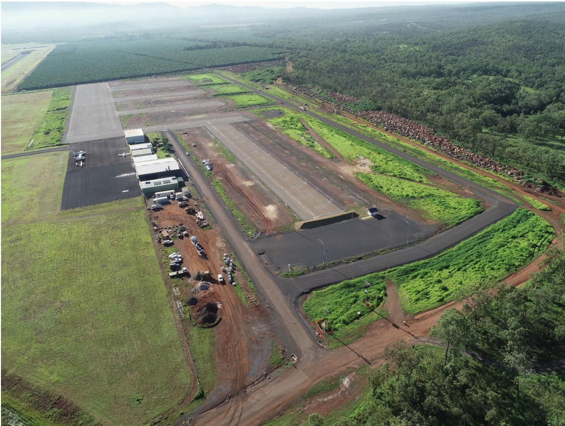
22 February 2018 - Aviation Park completed
