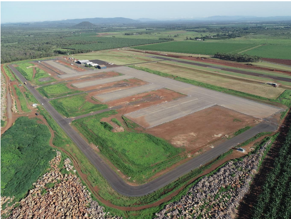
22 February 2018 - Aviation Park completed, with commencement of Stage 2 works underway
