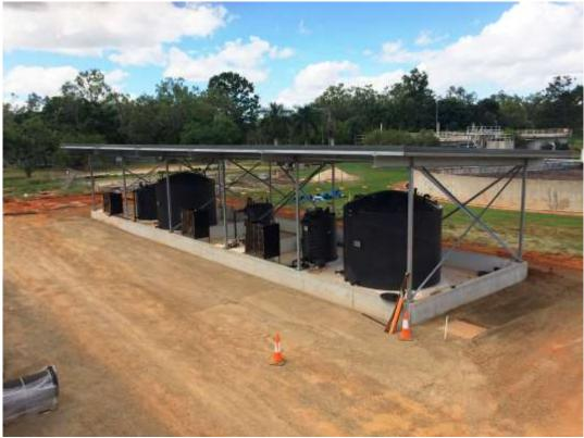
11 April 2017 - Installation of chemical storage tanks and dosing equipment
