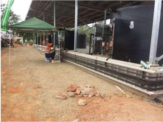
26 April 2017 - Installation of electrical cabling to chemical dosing area
