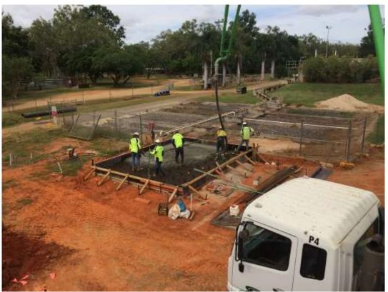
26 April 2017 - Pouring concrete base slab for trade waste receival facility
