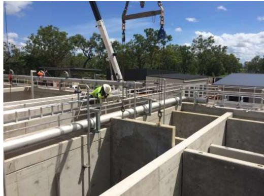
11 April 2017 - Lifting pre-cast concrete panels into bio-selector section of the sequential batch reactor (SBR)
