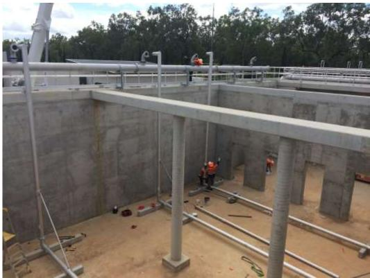
11 April 2017 - Installation of aeration pipework to sequential batch reactor (SBR)
