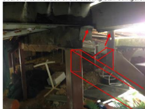
Joist & stringer inadequately connected. Make good all connections. Recommend 125x75x3 RHS bearer welded between columns & connecting 100x50x3 RHS tie fully welded to the bearer & to the face of the existing stair stringers.
