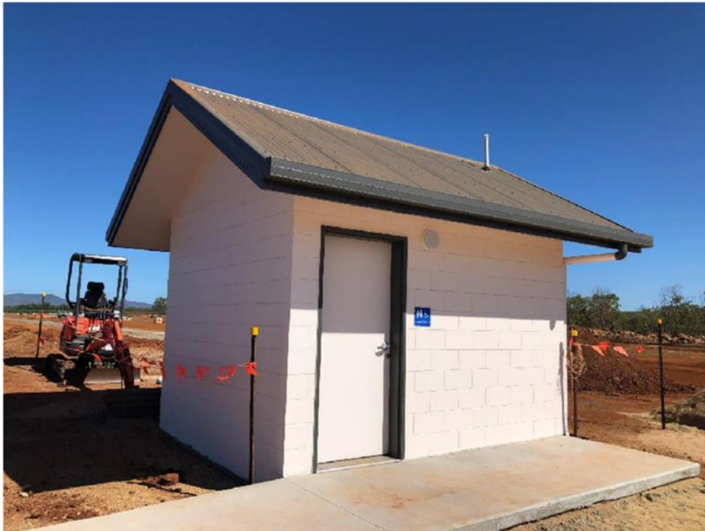
6 November 2018 - completion of amenities block for aviation industrial park
