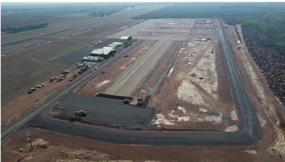
4 December 2018 - aerial imagery showing progress on aviation industrial park.
