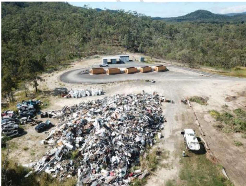
Figure 15 Upgraded Kuranda Waste Transfer Station 2017
