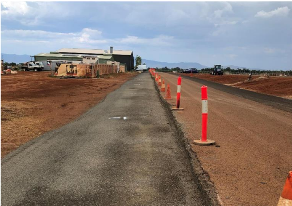
27 November 2018 - widening of JRM Braes Rd
