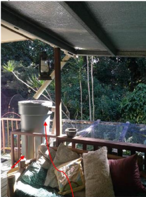
Corrosion to water tank stand, repair/replace &/or rust treat as required.
