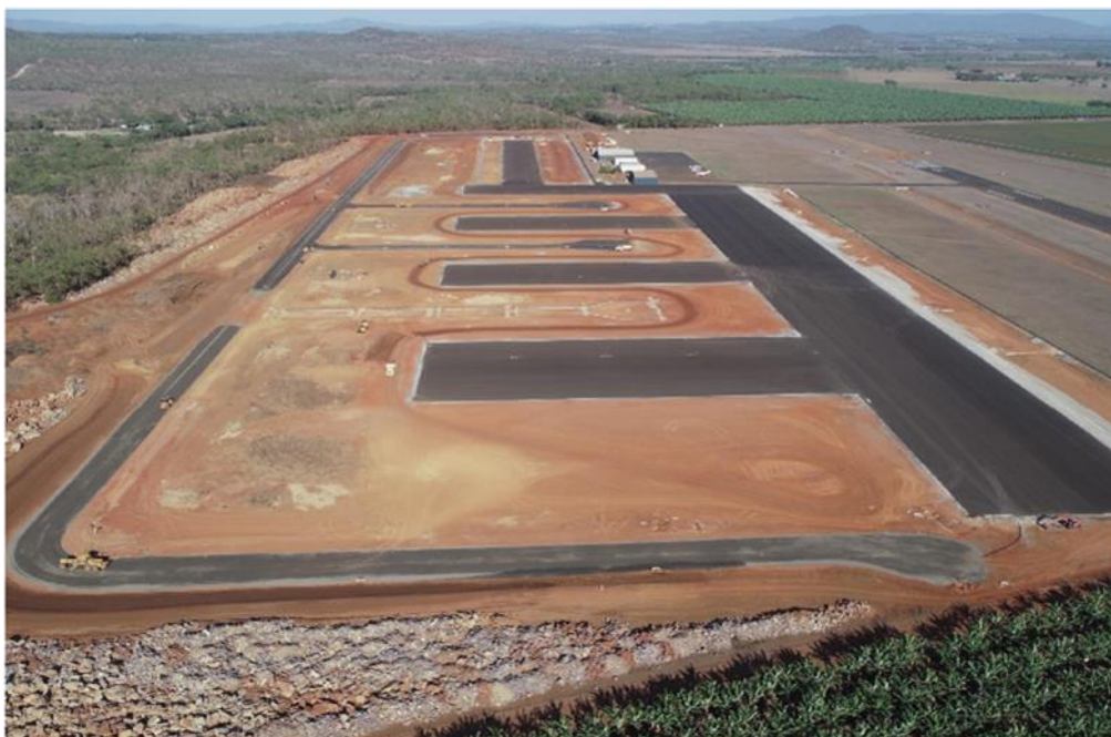
9 November 2018 - aerial imagery showing progress on aviation industrial park.
