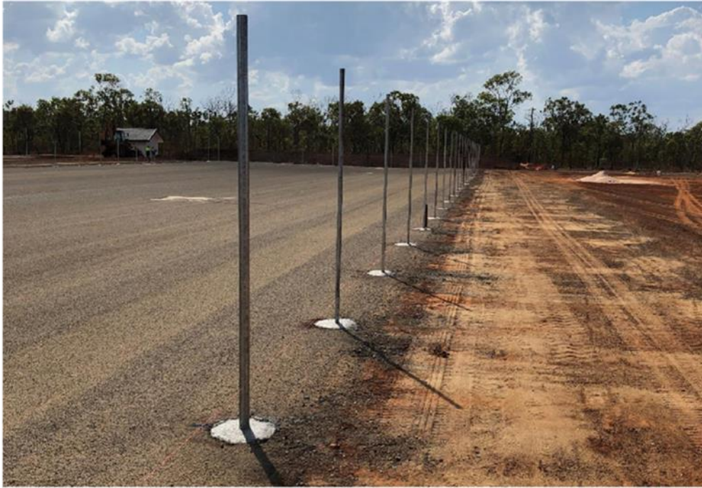
22 November 2018 - Installation of perimeter fencing to aviation industrial park
