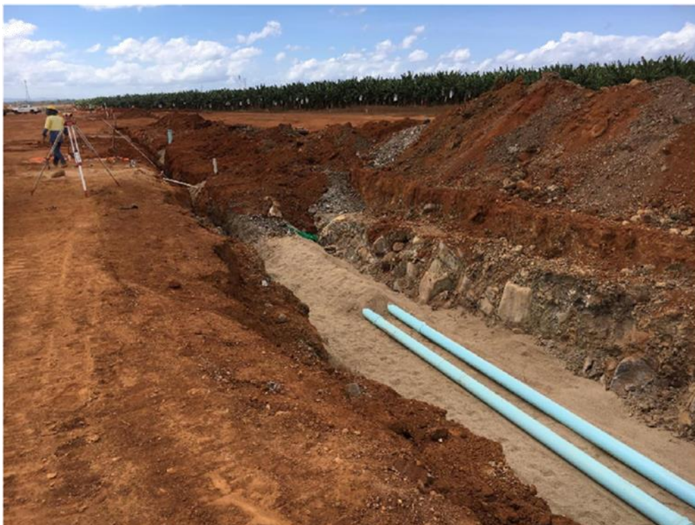
15 August 2018 - water main and fire water service installation
