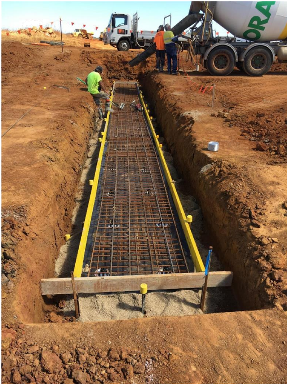
24 August 2018 - construction of box culvert base at carpark entrance
