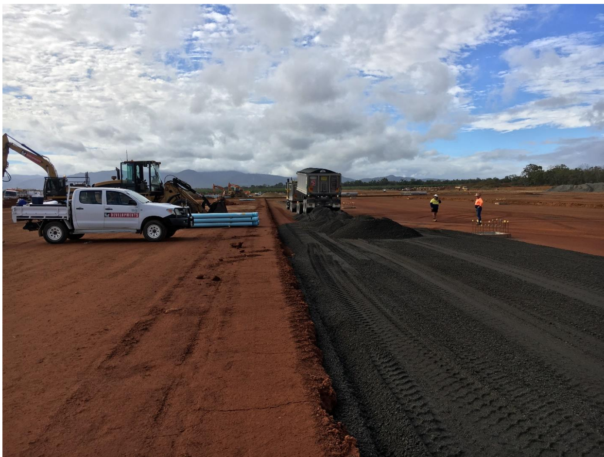
17 July 2018 - photograph showing pavement materials being delivered to site
