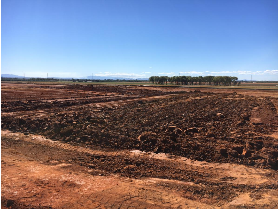
5 June 2018 - Earthworks on Taxiway E
