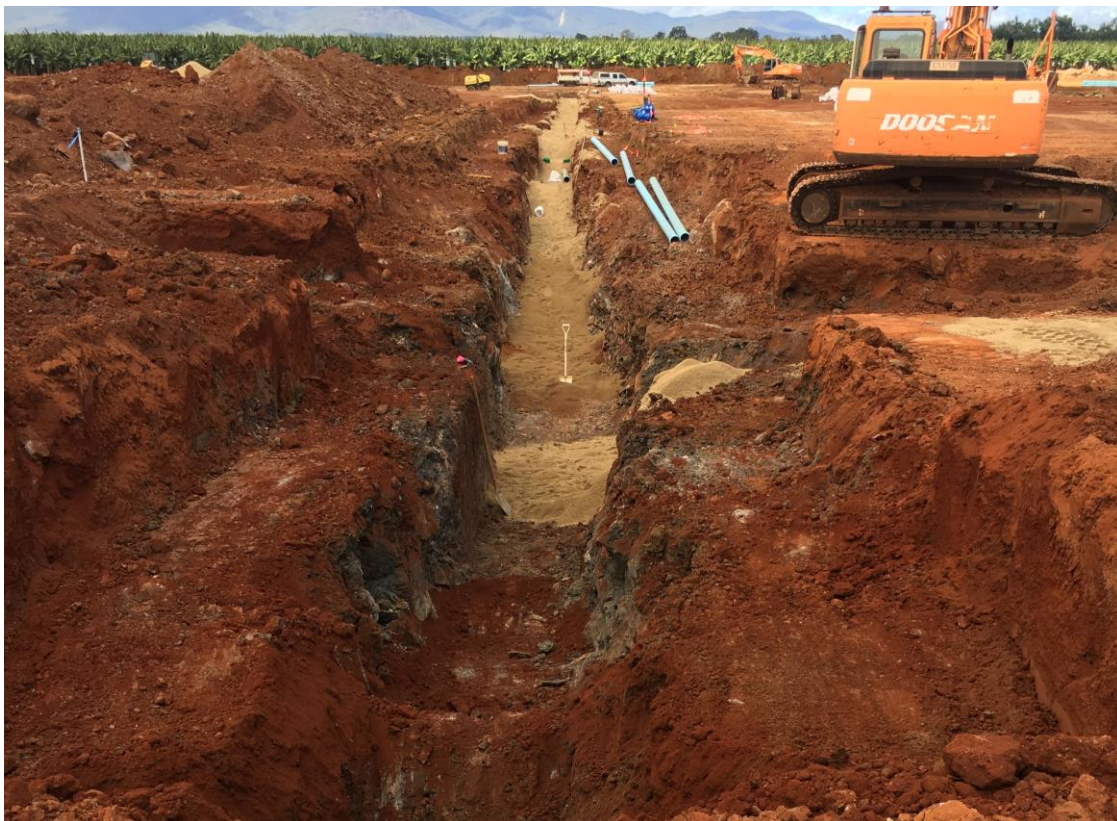
8 June 2018 - Trenching for potable and firefighting water
