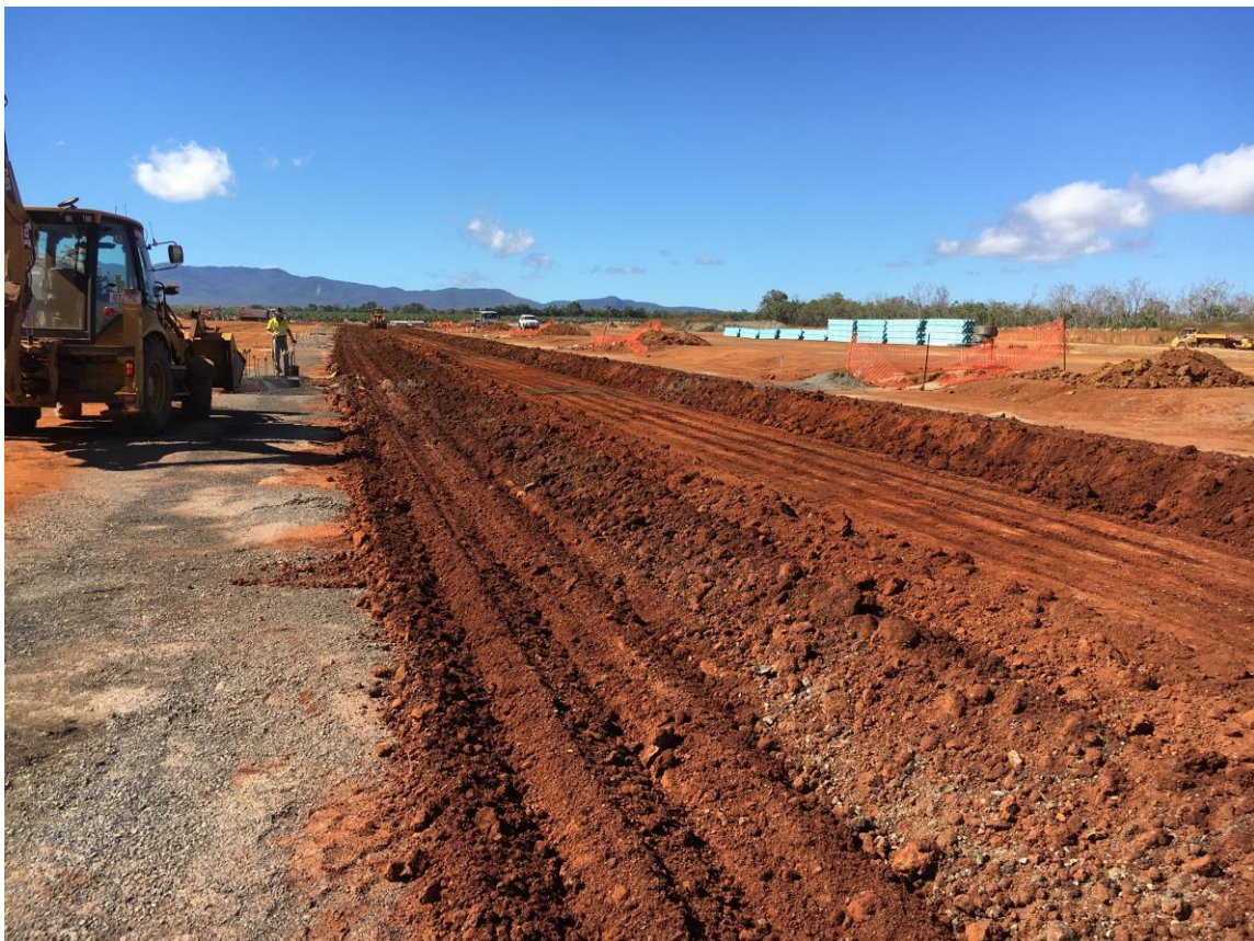
June 2016 - Subgrade construction for Taxiway F
