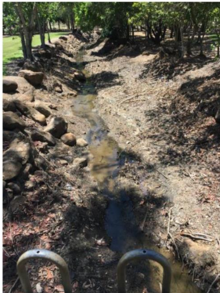
The weir removal has resulted in a lower detention time and water is flowing clear downstream. Upstream (photo RHS) water is flowing clear in a smaller channel.
