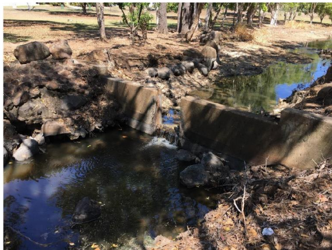
Weir with slats removed
