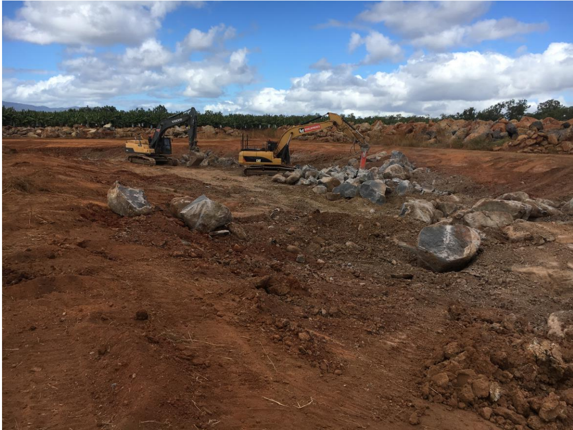
8 June 2018 - Excavation for Road 1 and rock removal
