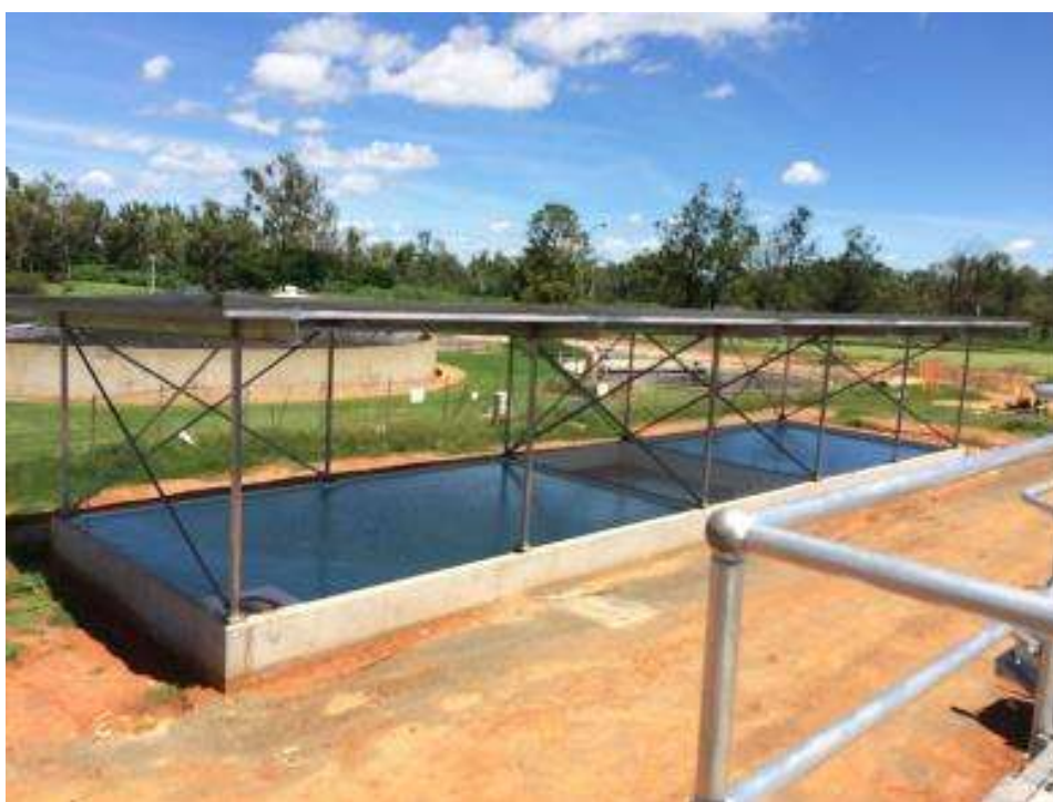
27 March 2017 - Hydrostatic testing of bunds in chemical dosing area
