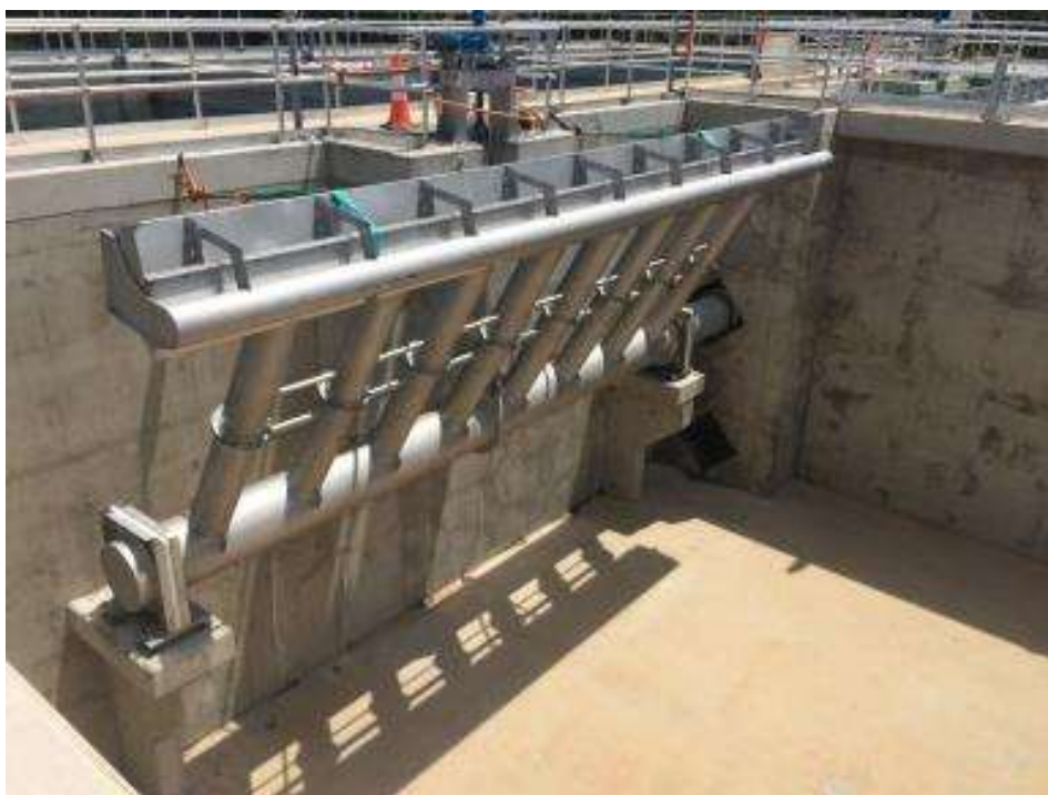
20 March 2017 - Decanter installed to SBR
