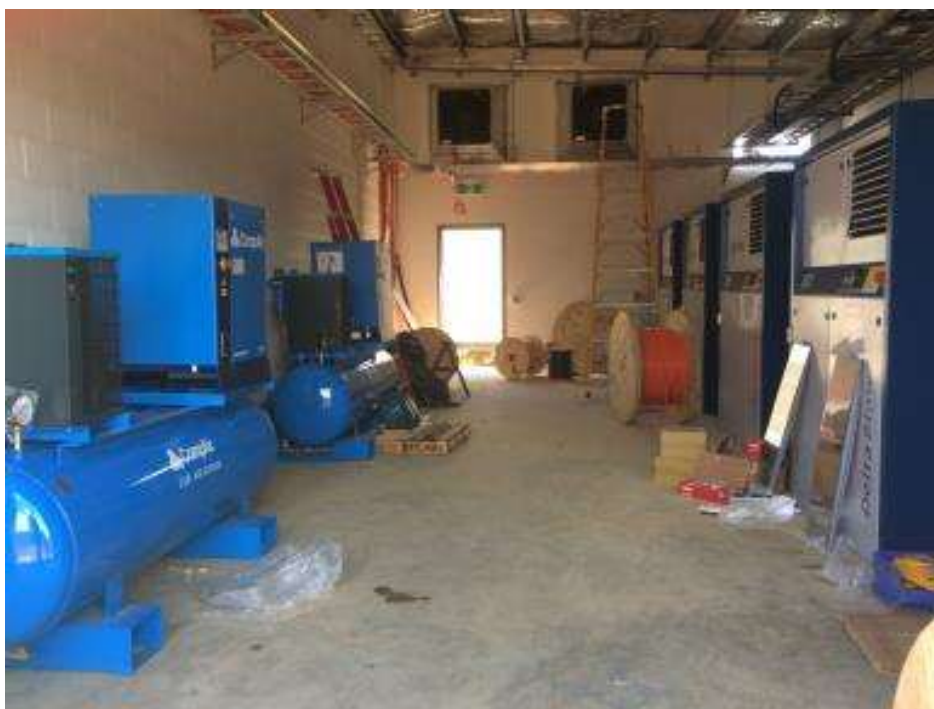
20 March 2017 - Compressors and blowers installed
