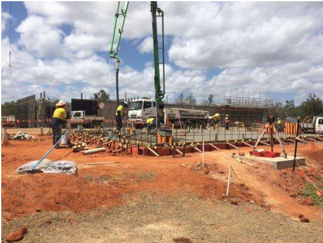
22 November 2016 - Concrete floor slab for Administration and Motor Control Centre (MCC) building being poured
