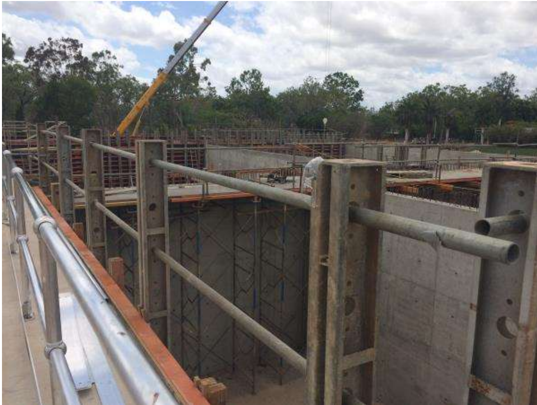
22 November 2016 - Progress on construction of Sequential Batch Reactor (SBR) walls and installation of walkway handrails commenced
