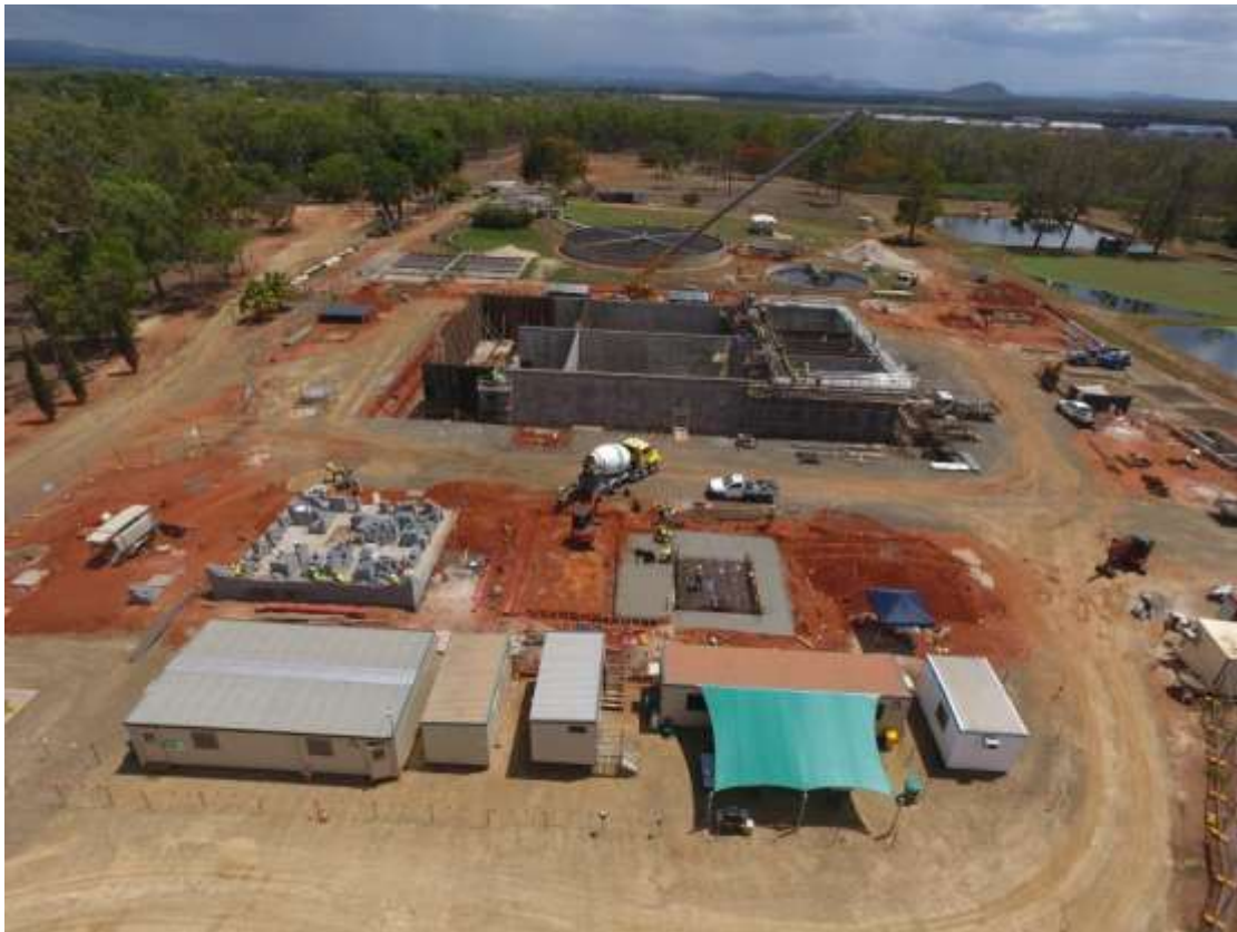
30 November 2016 - Aerial photograph of the project site showing construction of the site buildings
