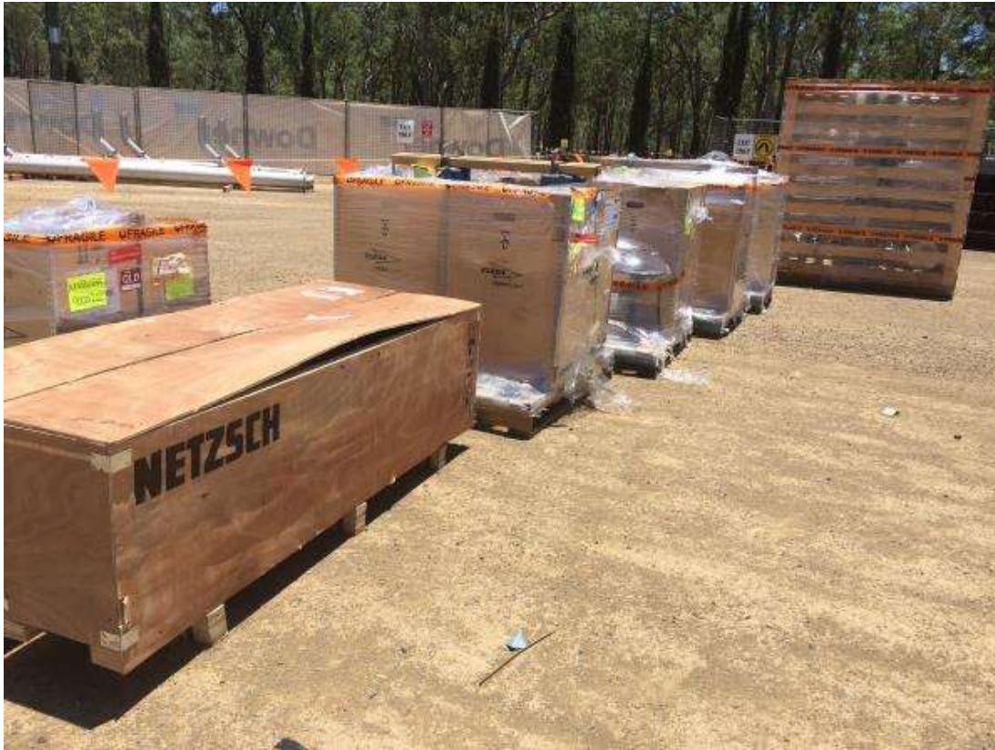
15 November 2016 - Pumps received on-site
