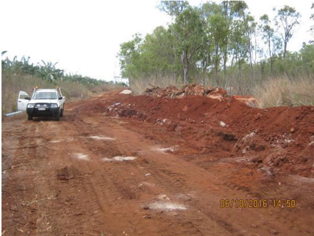
6 October 2016 - Rock encountered during trenching for potable water main from Wylandra Reservoir
