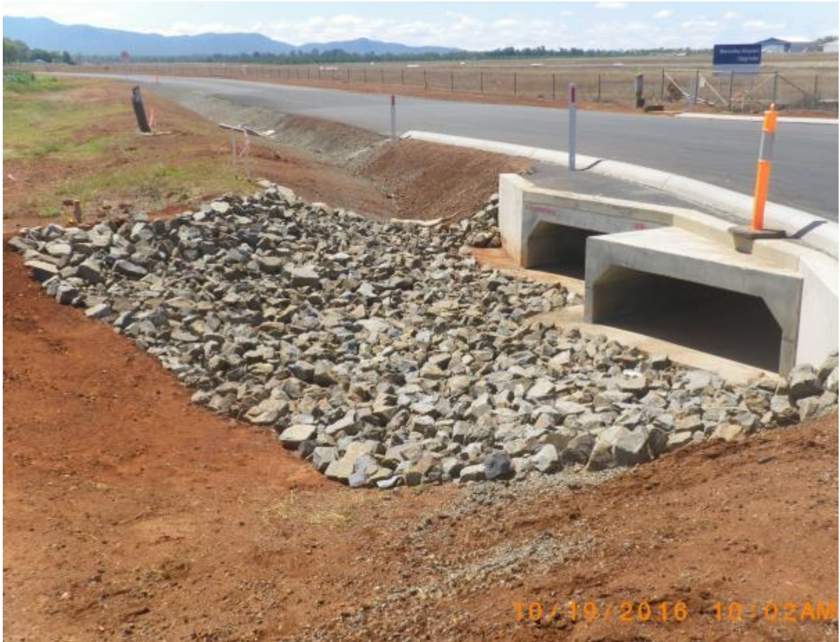
19 October 2016 - Completed culvert and surfacing at Intersection of Vicary Road and Ray Road
