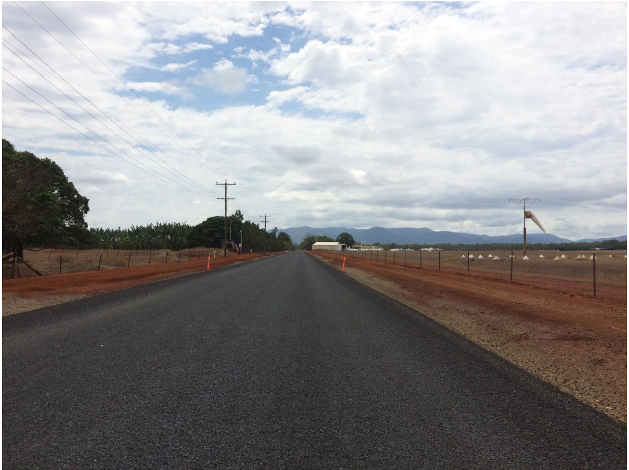
5 November 2016 - Vicary Road widening following completion of two-coat bitumen seal
