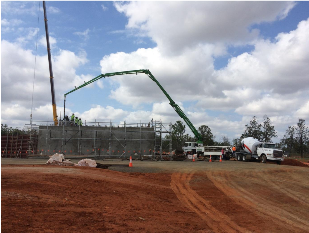
13 October 2016 - Concrete pour for Sequential Batch Reactor (SBR) Walls
