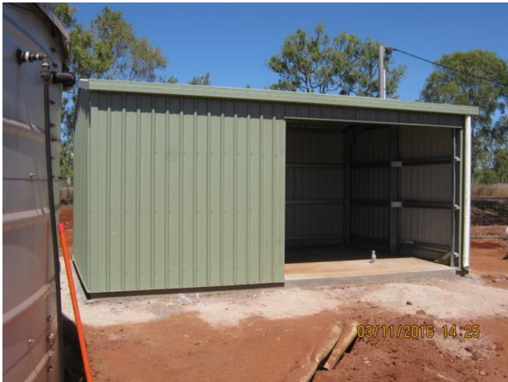
3 November 2016 - Structure installed for new potable water pumps and back-up generator
