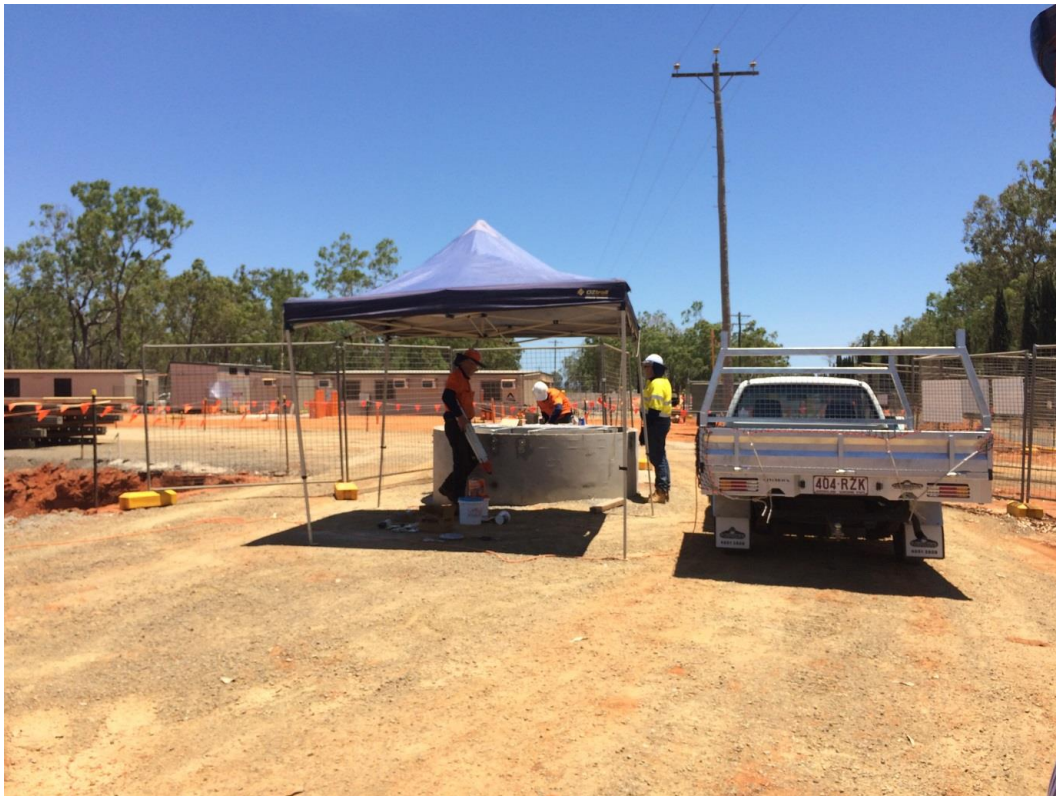
1 November 2016 - Installation of Cover to General Purpose Pumping Station (GPPS)
