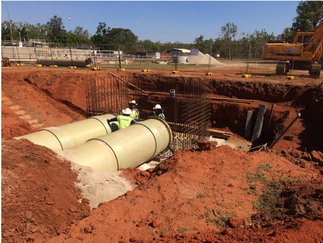
19 October 2016 - Installation of wall reinforcement for Chlorine Contact Tank (CCT)
