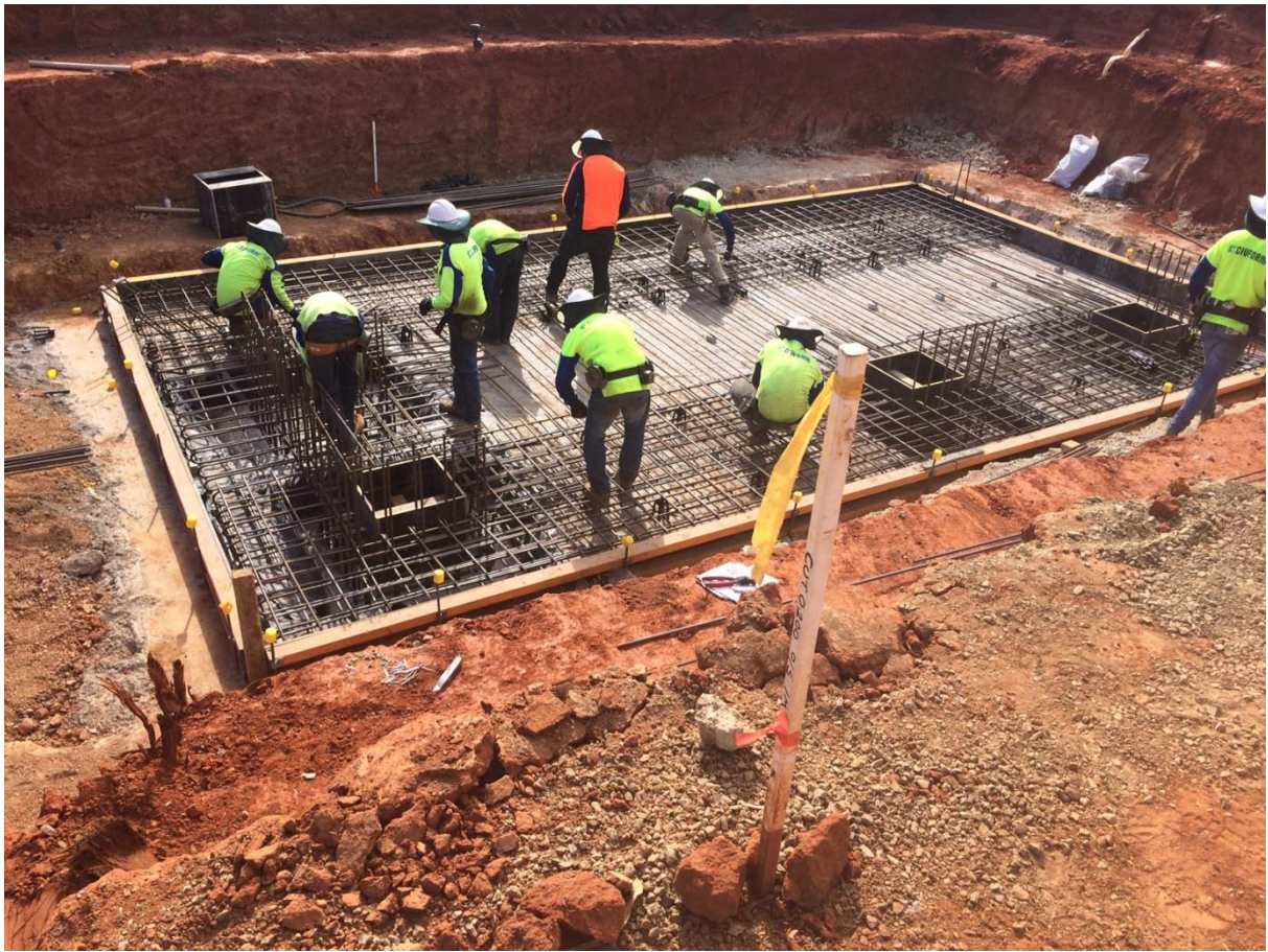
1 September 2016 - Installation of reinforcement for chlorine contact tank (CCT) base slab
