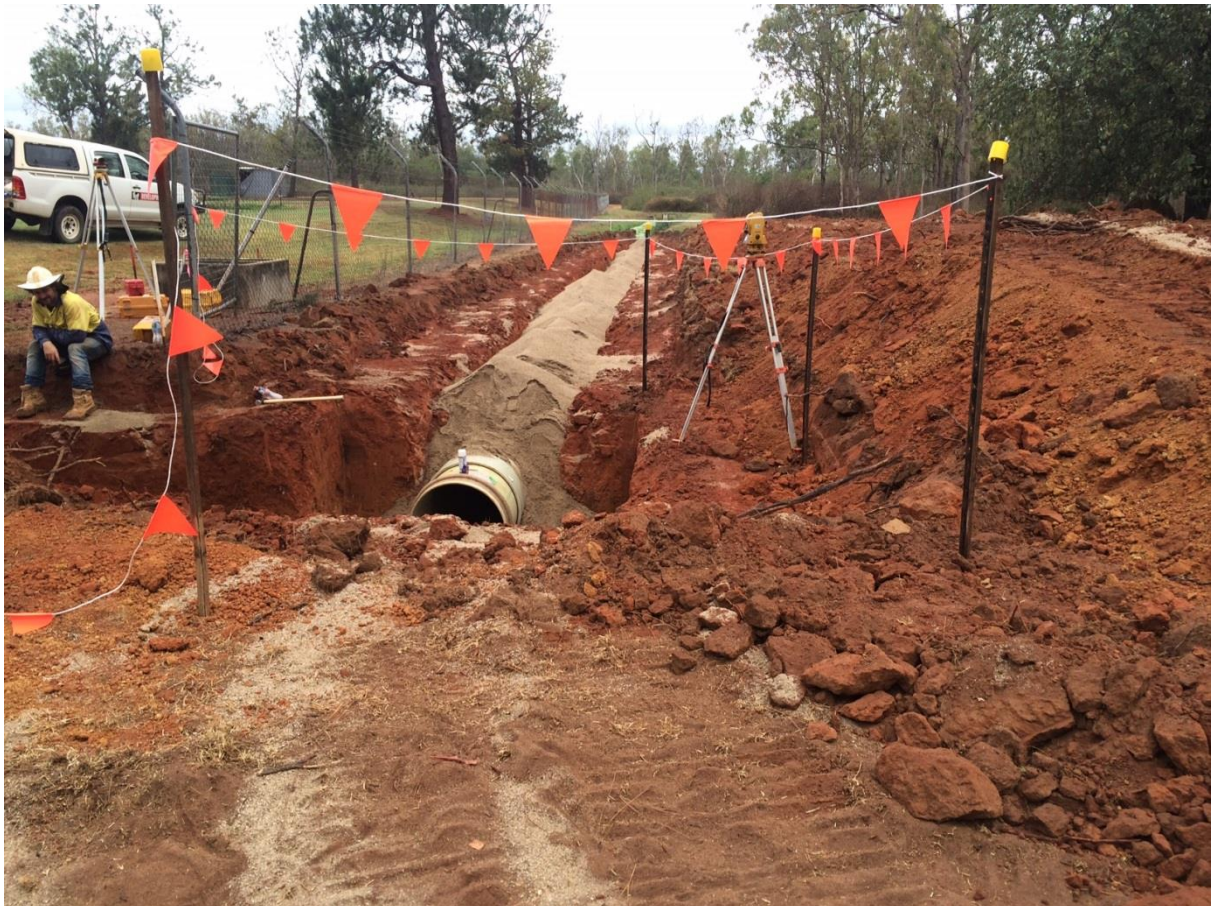
12 September 2016 - Installation of outfall pipework
