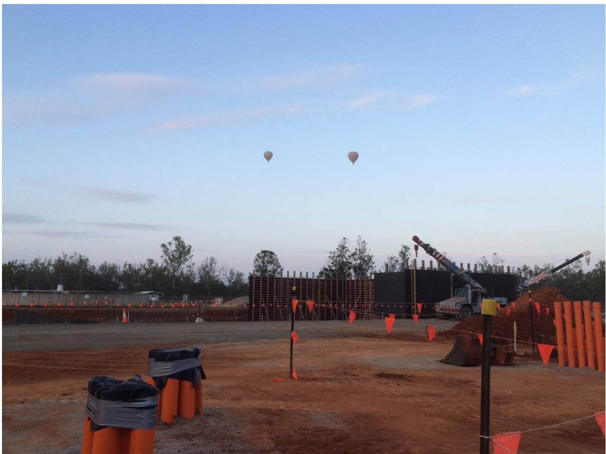
21 September 2016 - Sunrise at the project site; Electrical Conduit to MCC and SBR wall formwork in place
