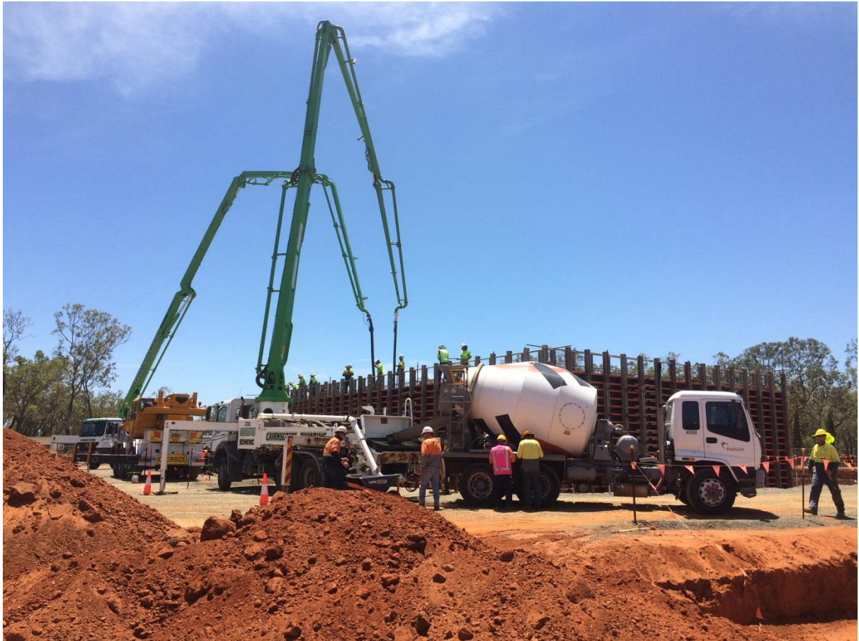
27 September 2016 - Concrete pour for the SBR and Digester walls
