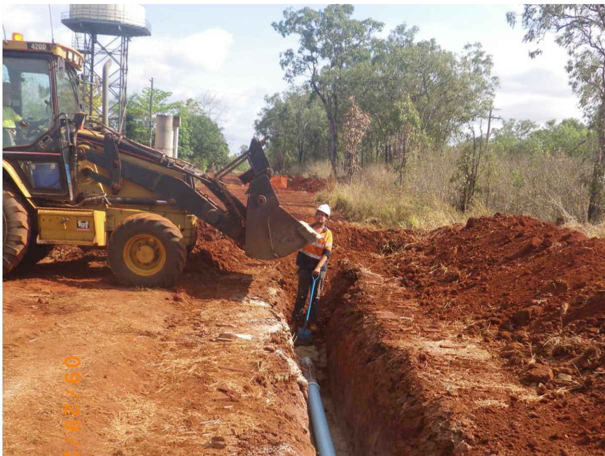
29 September 2016 - Water main installation from Wylandra reservoir to Mareeba Airport
