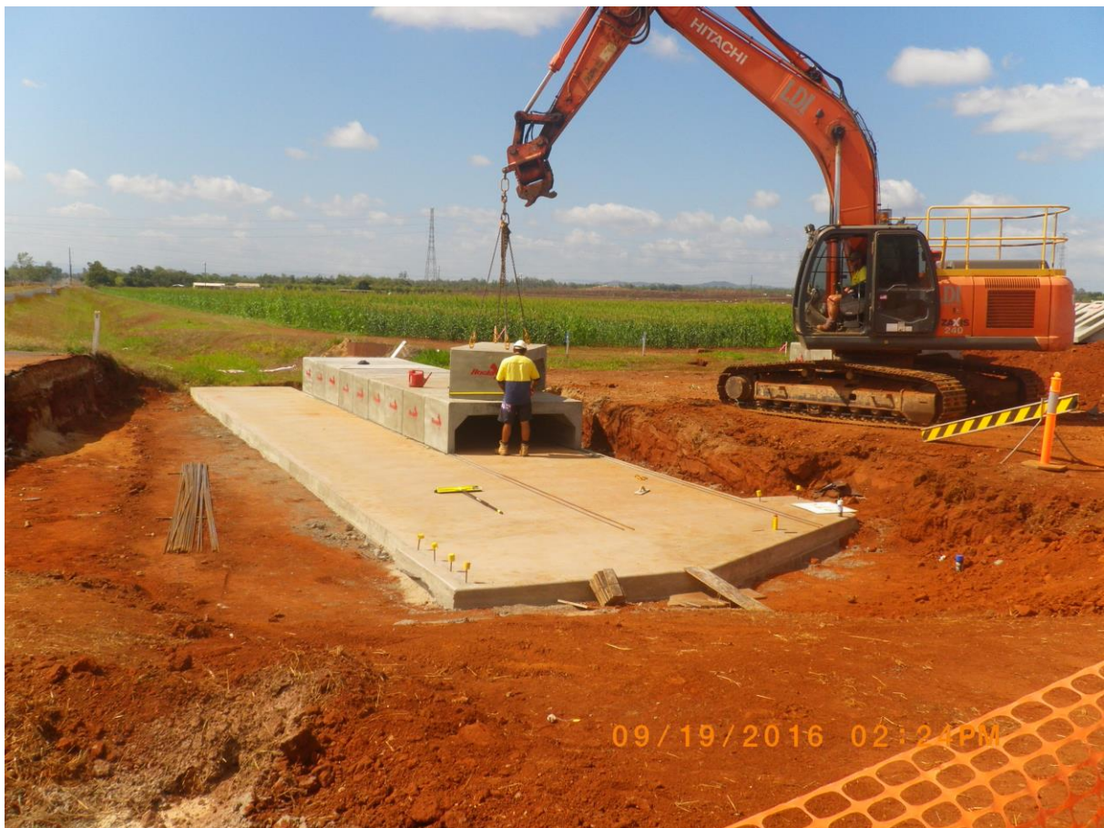
19 September 2016 - Culvert installation at intersection of on Vicary Road and Ray Road
