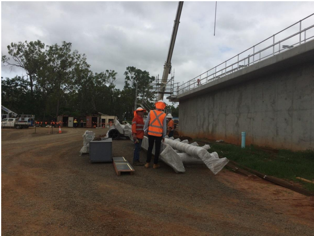
7 February 2017 - Inspection of the Decanters prior to assembly
