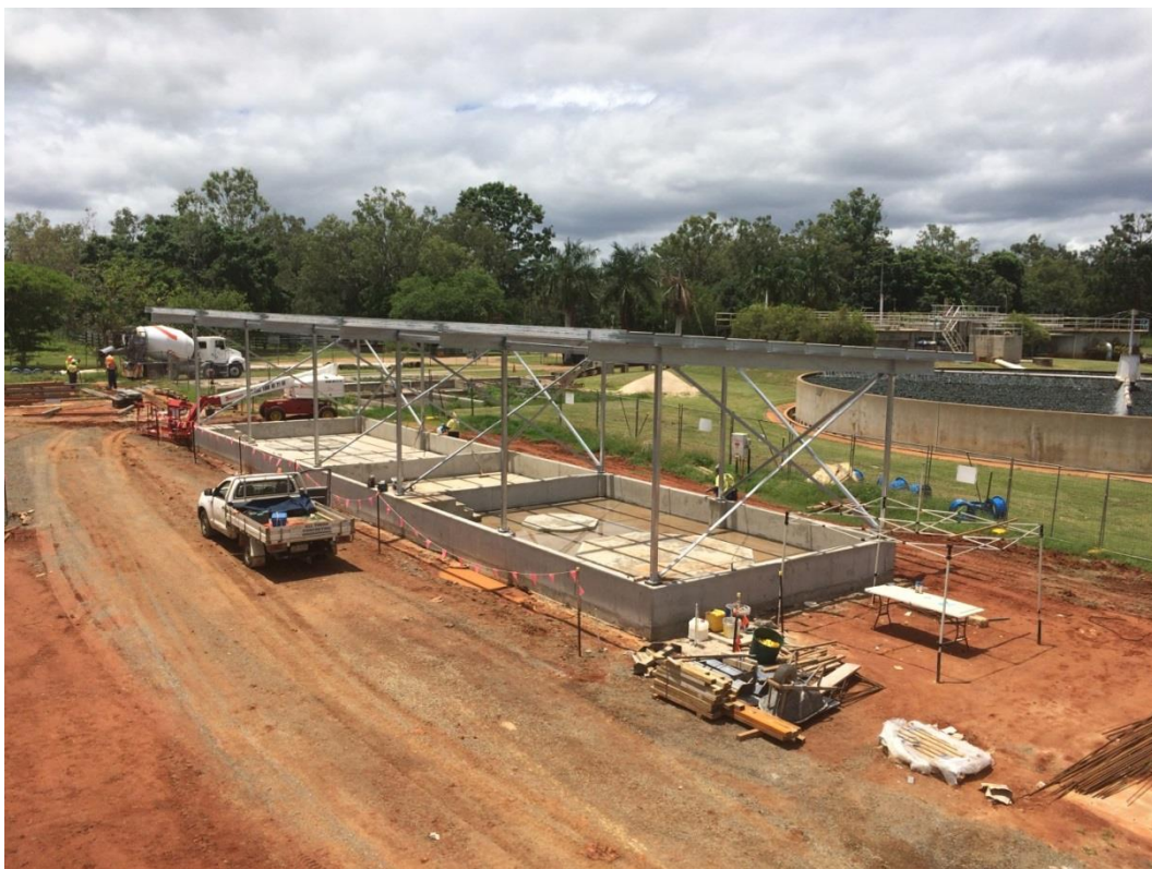
24 February 2017 - Roof framing installed to chemical dosing area
