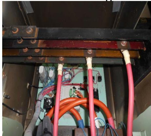
Main Busbar and bus Supports
