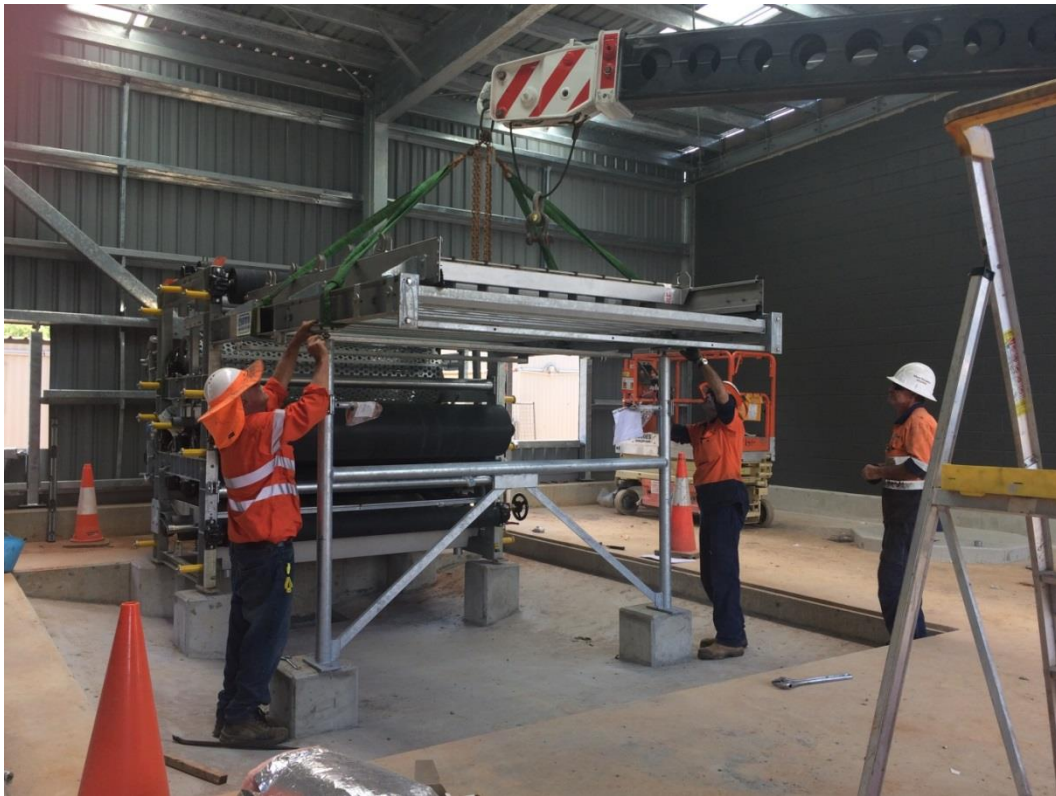
24 February 2017 - Installation of belt filter press in the sludge dewatering building
