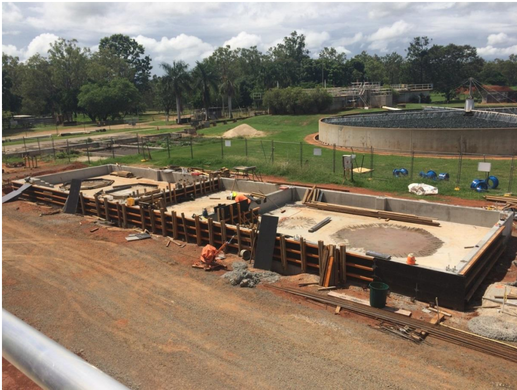
17 February 2017 - Construction of Concrete Bunds for Chemical Dosing Area
