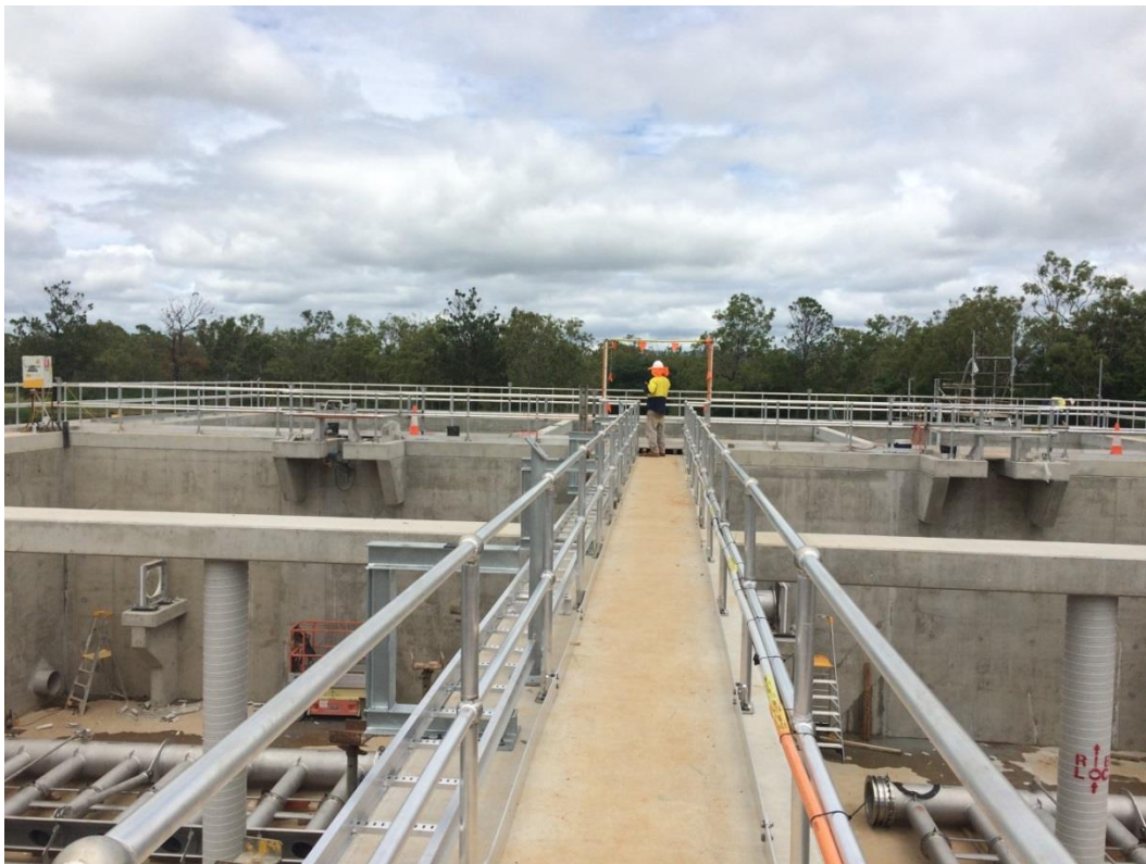
14 February 2017 - Installation of Cable Trays along SBR Walkway; Decanters assembled and stored on floor of SBR
