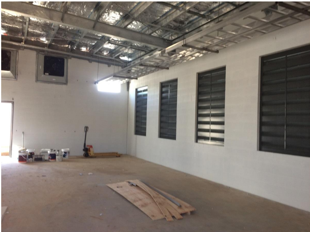
28 February 2017 - Completion of internal painting and installation of louvers to blower building
