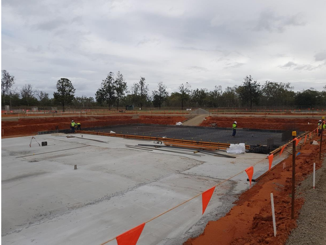
16 August 2016 - Installation of reinforcement for bioreactor (SBR) base slab
