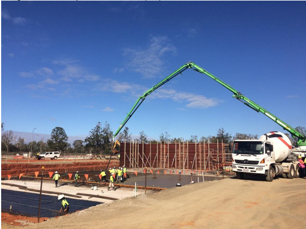
31 August 2016 - Concrete pour No. 2 for bioreactor (SBR) base slab
