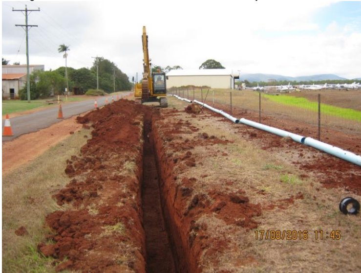
6 September 2016 - Installation of new Fire Main on southern side of Runway
