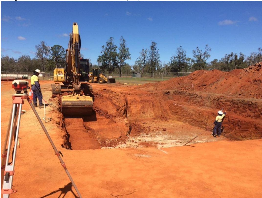
23 August 2016 - Excavation for chlorine contact tank (CCT)
