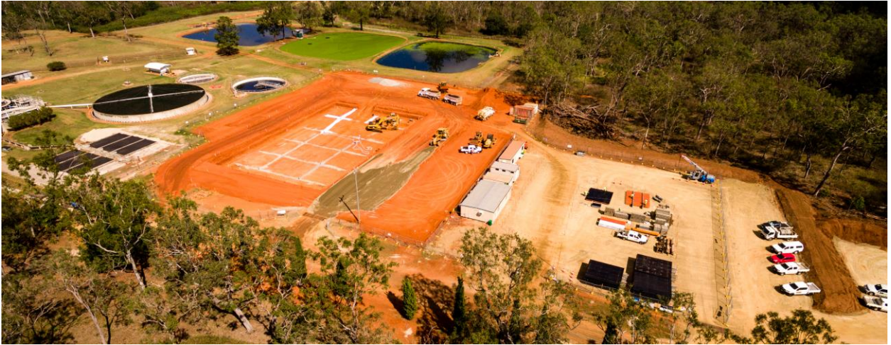
Aerial photograph of Mareeba Waste Water Treatment Plant under construction - 3 August 2016
