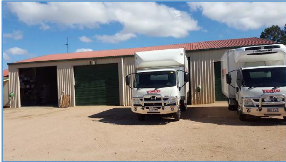
Image 1: Existing four (4) bay shed used to house existing logistics operations.
