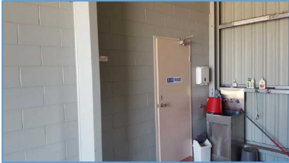
Image 3: Existing access to staff facilities contained within the existing shed.
