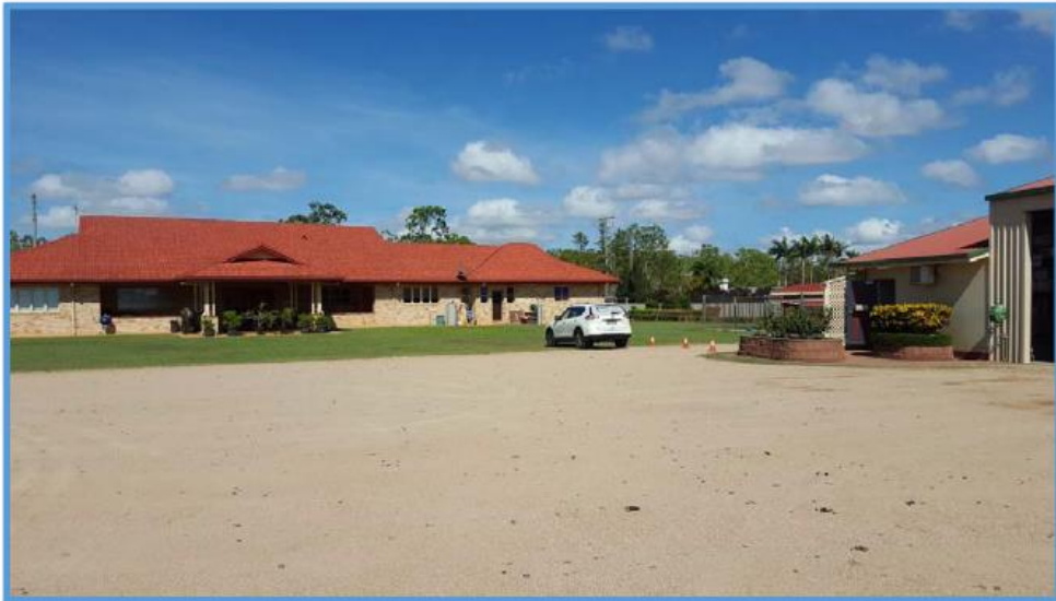
Image 7: Westerly view of the existing development taken from the existing parking/manoeuvring area associated with the logistics company, illustrating the level of separation between the shed and the existing company.
