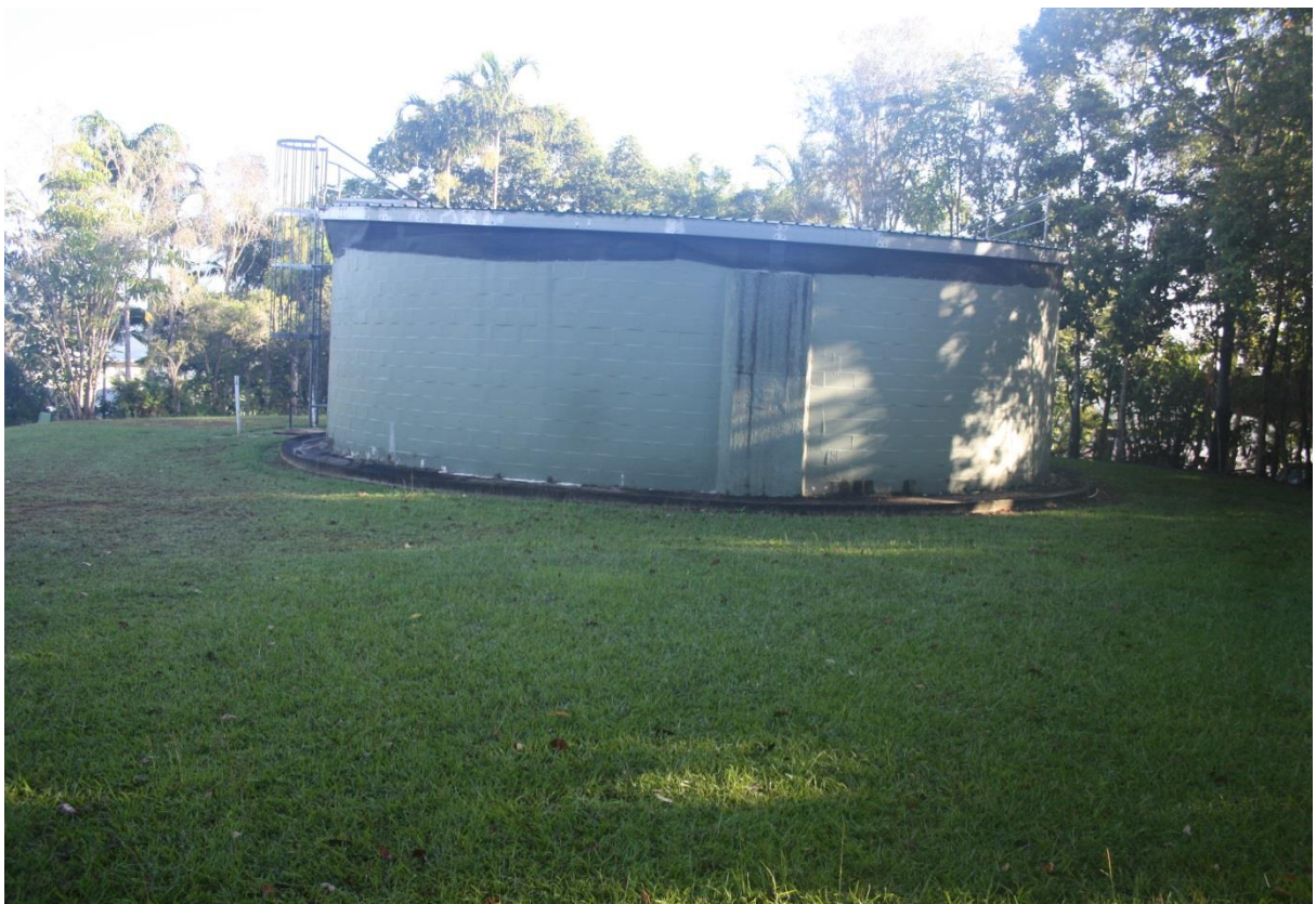
Existing 350 kL reservoir Hilltop Close
