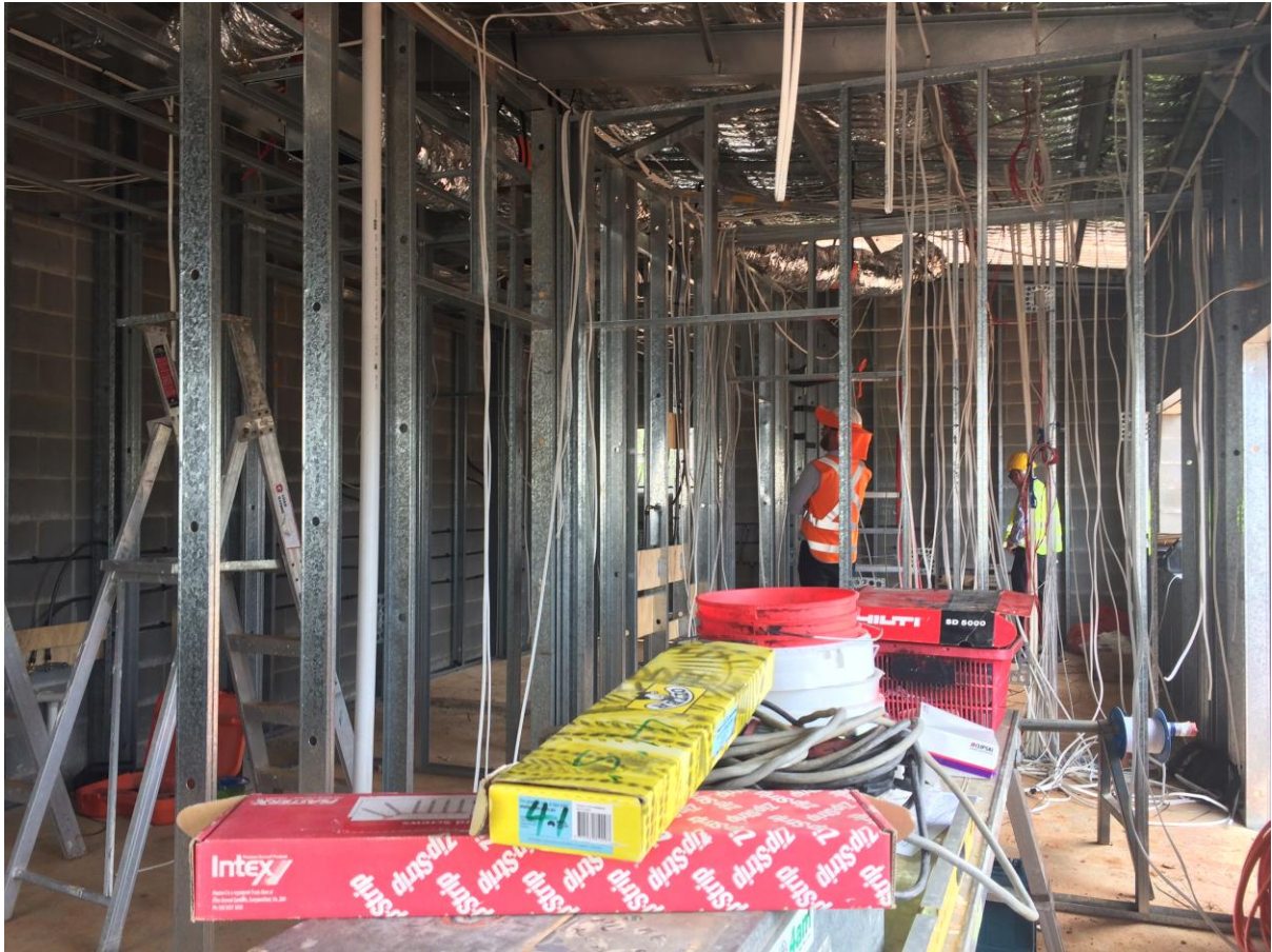
31 January 2017 - Fitout of the MCC Room underway
