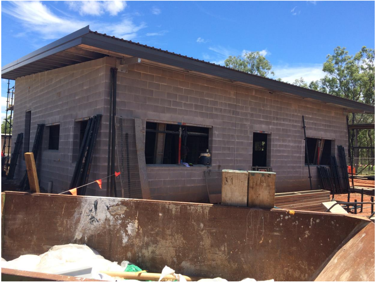
16 January 2017 - Completion of roof installation to the Admin and MCC Building
