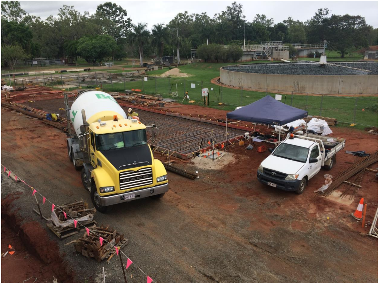
31 January 2017 - Commencement of base slab for Chemical Dosing Area
