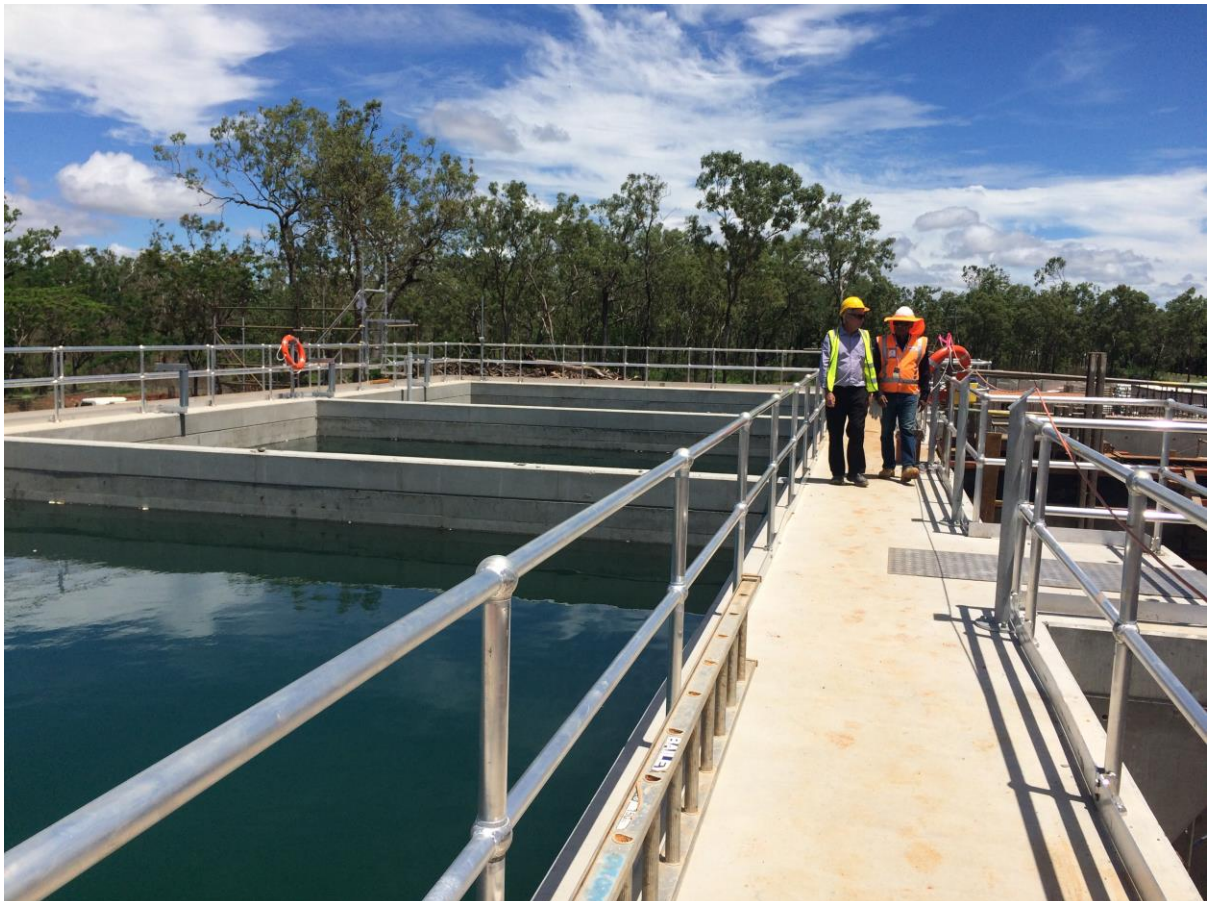
16 January 2017 - Inspection of walkways to sequential batch reactor (SBR)
