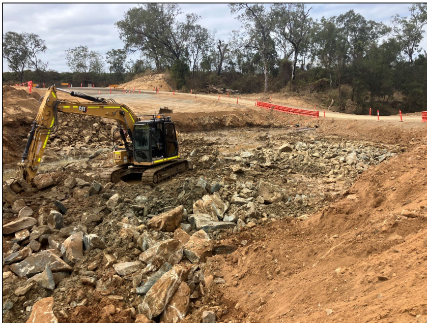
Preparation of culvert base slab subgrade
