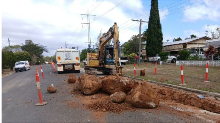
Trenching works and rock on Constance Street
