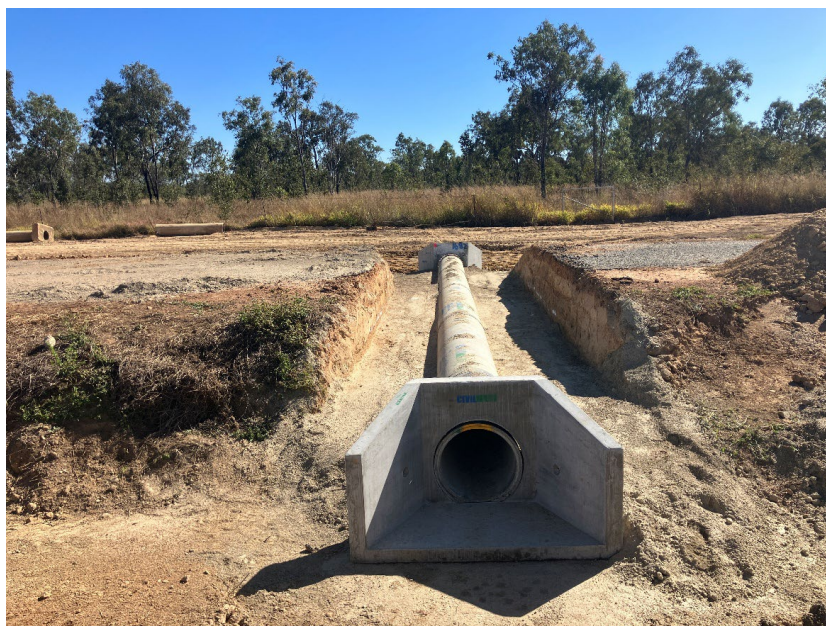
Culvert crossing construction
