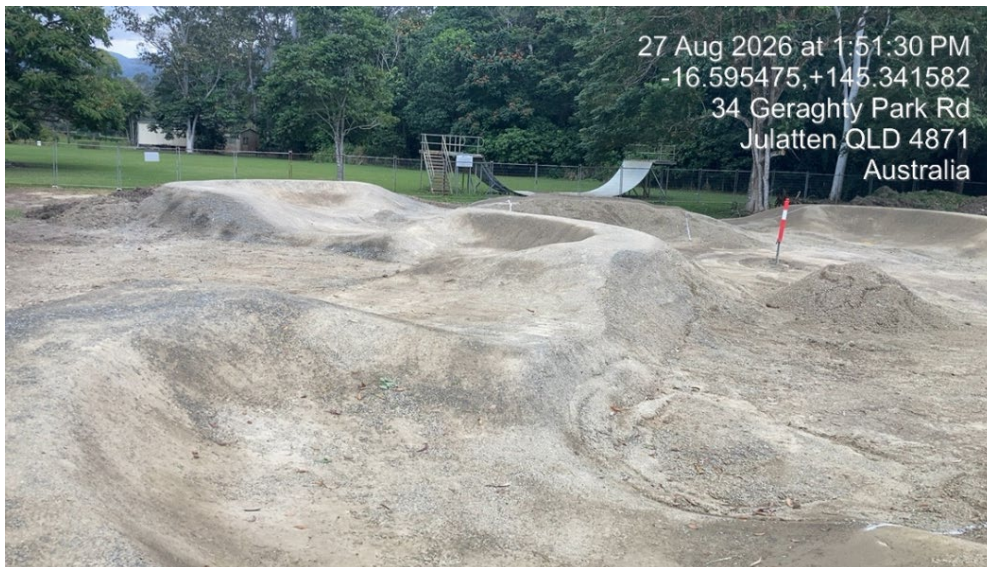
Completed, compacted earthworks for the track - ready for asphalt
