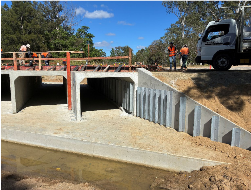
Ada Creek Causeway culverts, wingwalls and apron installed with deck fabrication commenced
