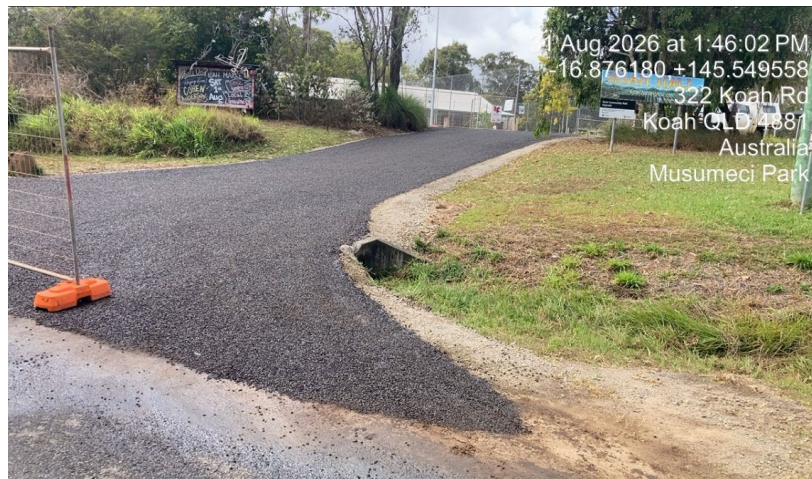
Driveway and crossover – Koah Hall entrance
