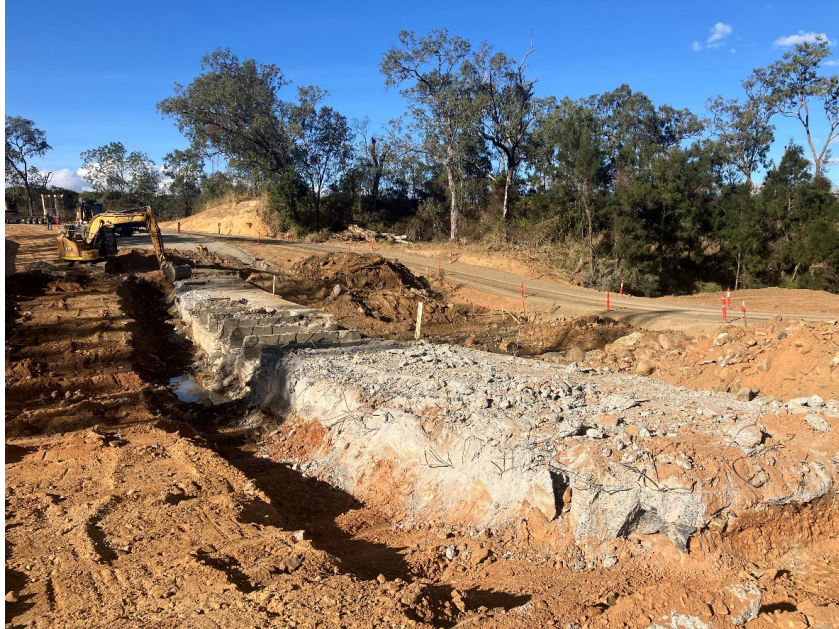
Demolition of existing crossing
