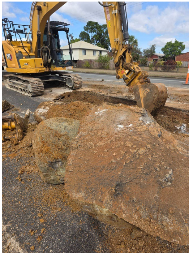
Trenching works on Constance Street
