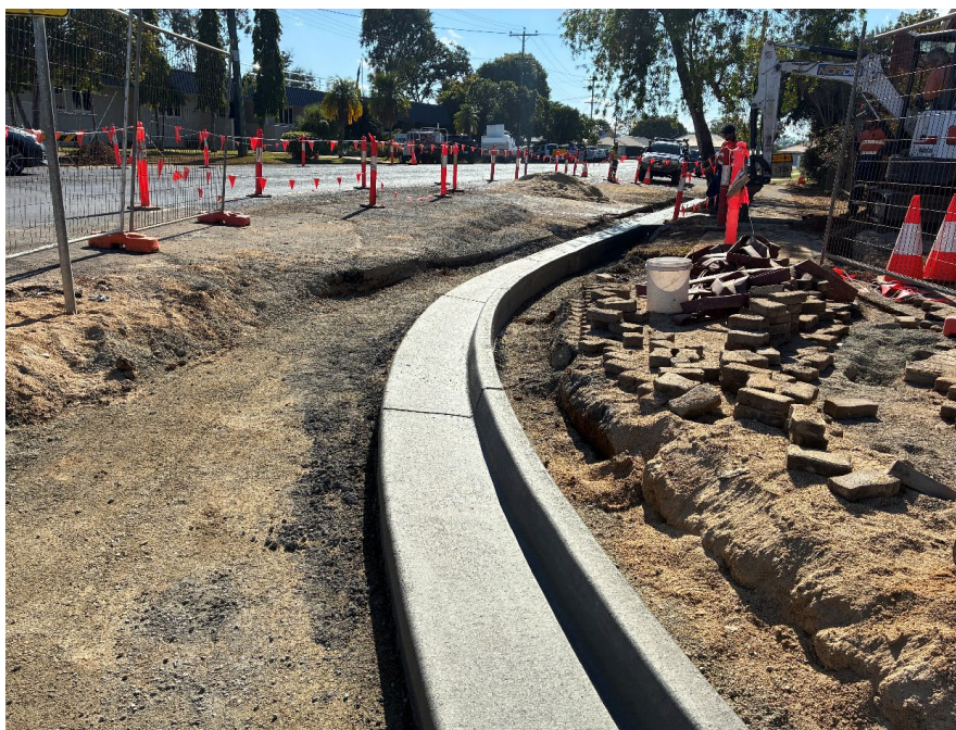
Kerb and Channel Installation on the corner of Walsh and Rankin Streets
