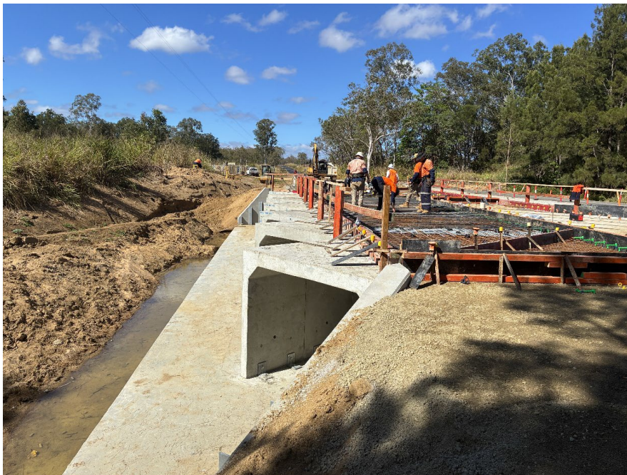
Ada Creek Causeway culverts, wingwalls and aprons installed with deck fabrication commenced
