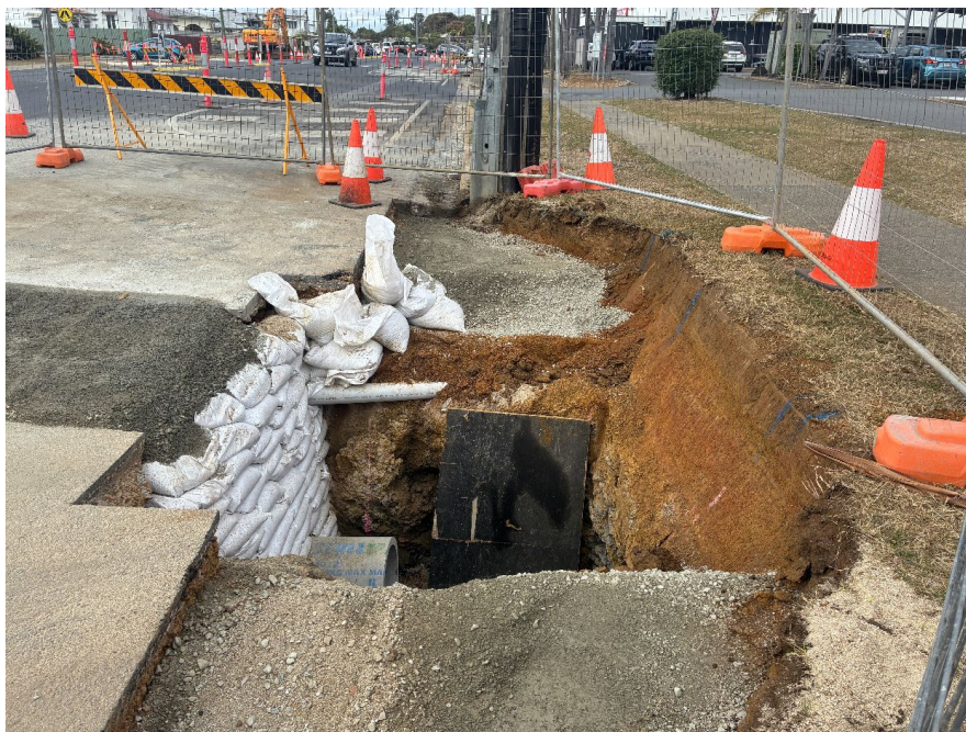
Kerb Inlet Pit Preparation
