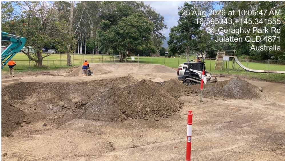
Earthworks for the berms and rolls
