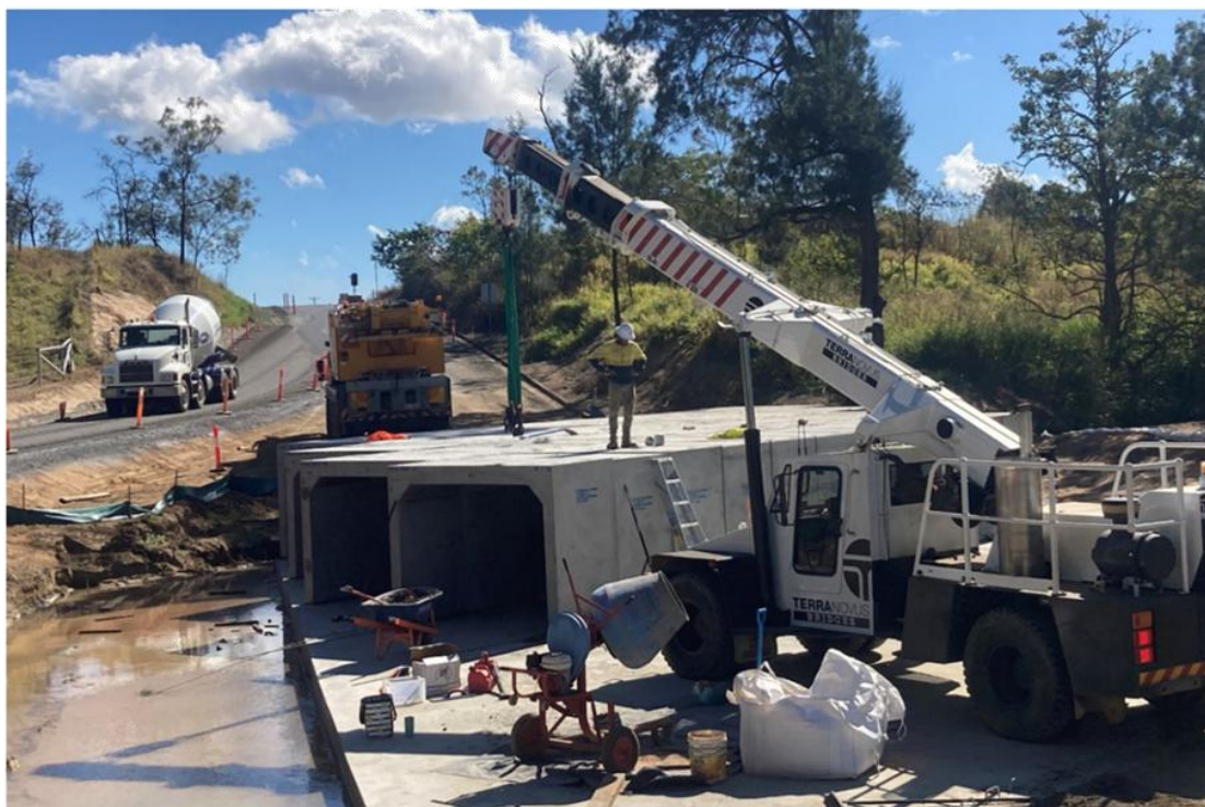
Ada Creek Box Culvert Placement
