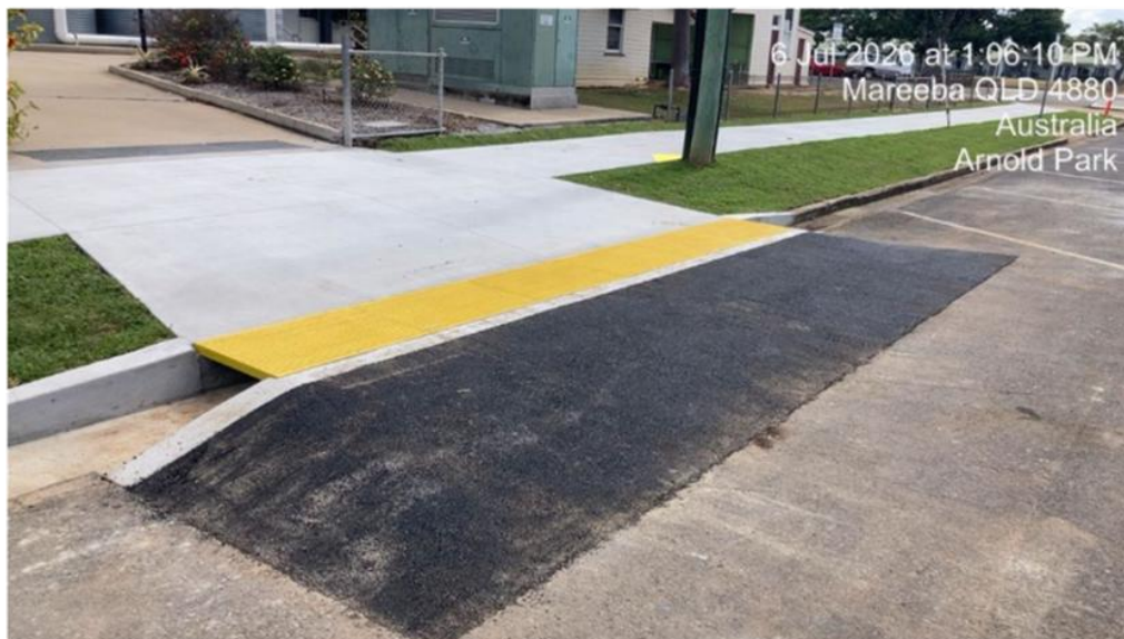
Driveway crossover – Mareeba Courthouse
