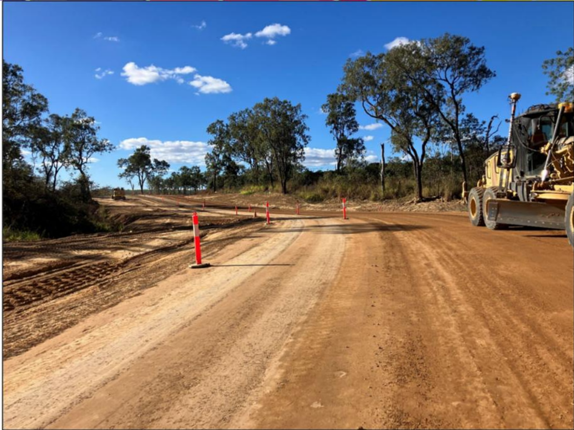
Preparation of subgrade
