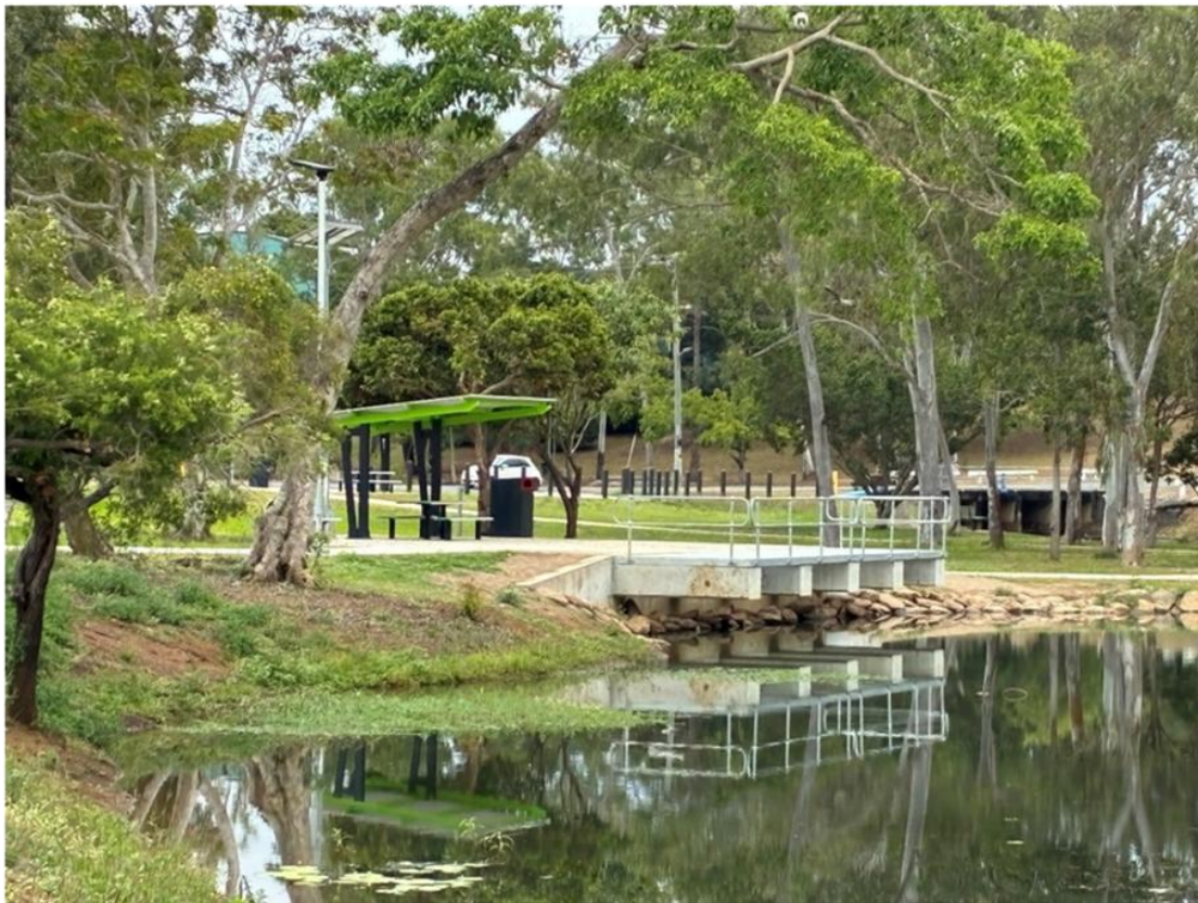
New Viewing Deck where an Interpretive/ Information Sign will be installed
