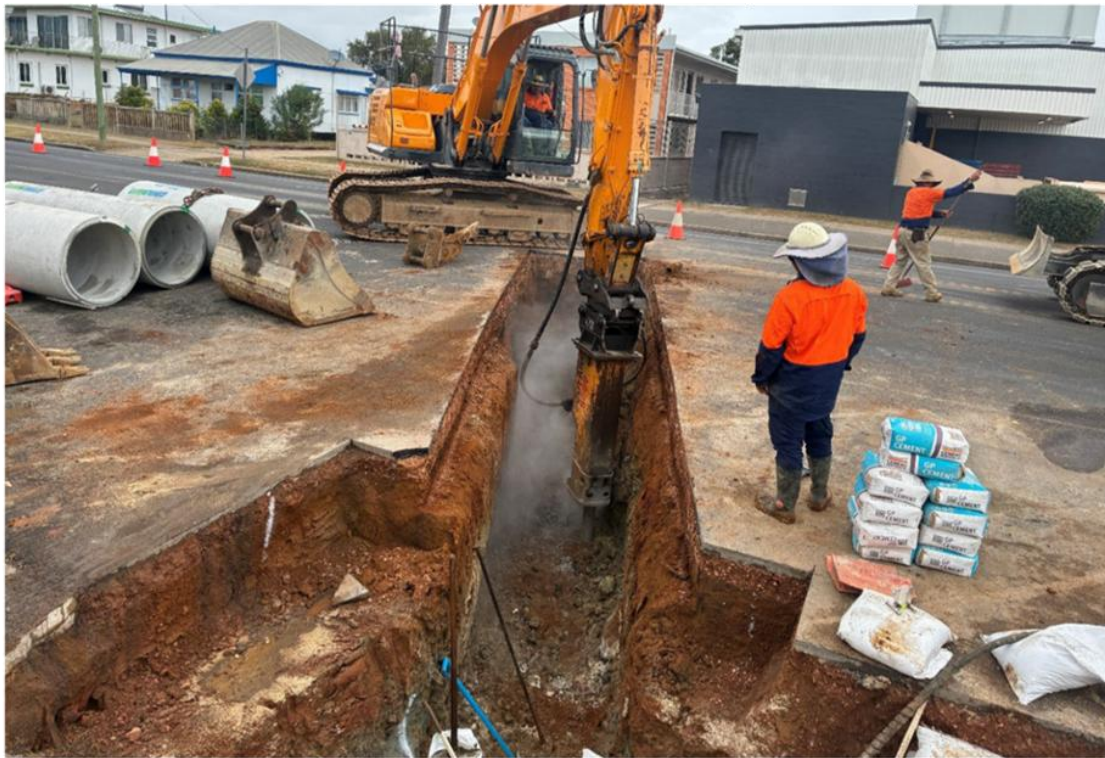
450mm Pipe Crossing & Rock Breaking at the Bottom of the Trench
