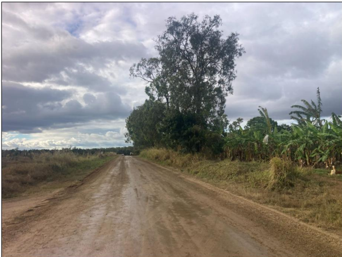
Resheet completed on Slape Road
