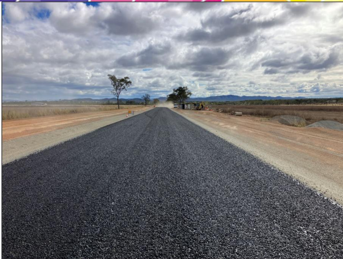
Sealing of Leedingham Road
