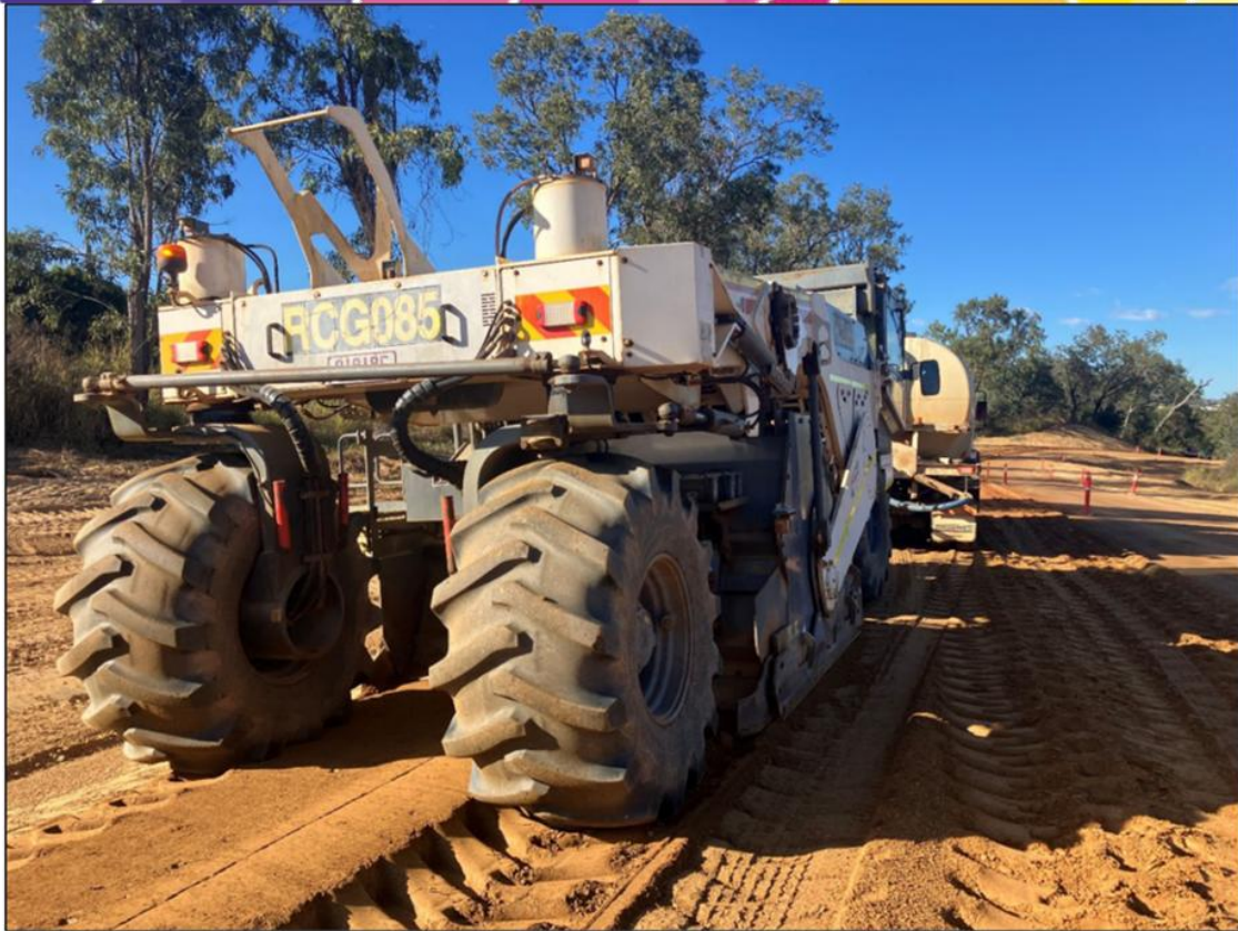
Preparation of subgrade
