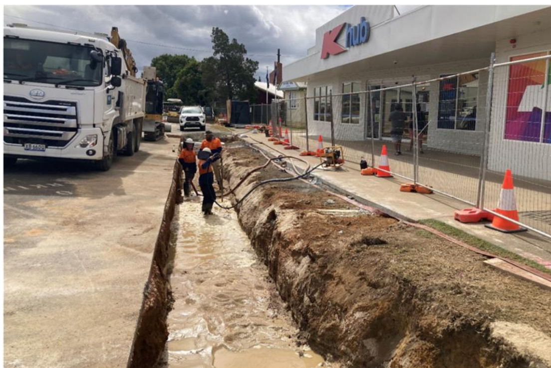
Stormwater Pipeline Installation Sand Backfill & Flooding
