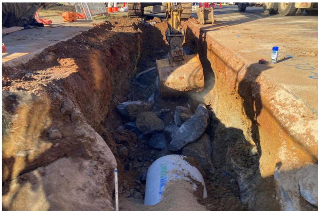
Stormwater Trench Excavation at K-Hub Indicating Rock Being Encountered
