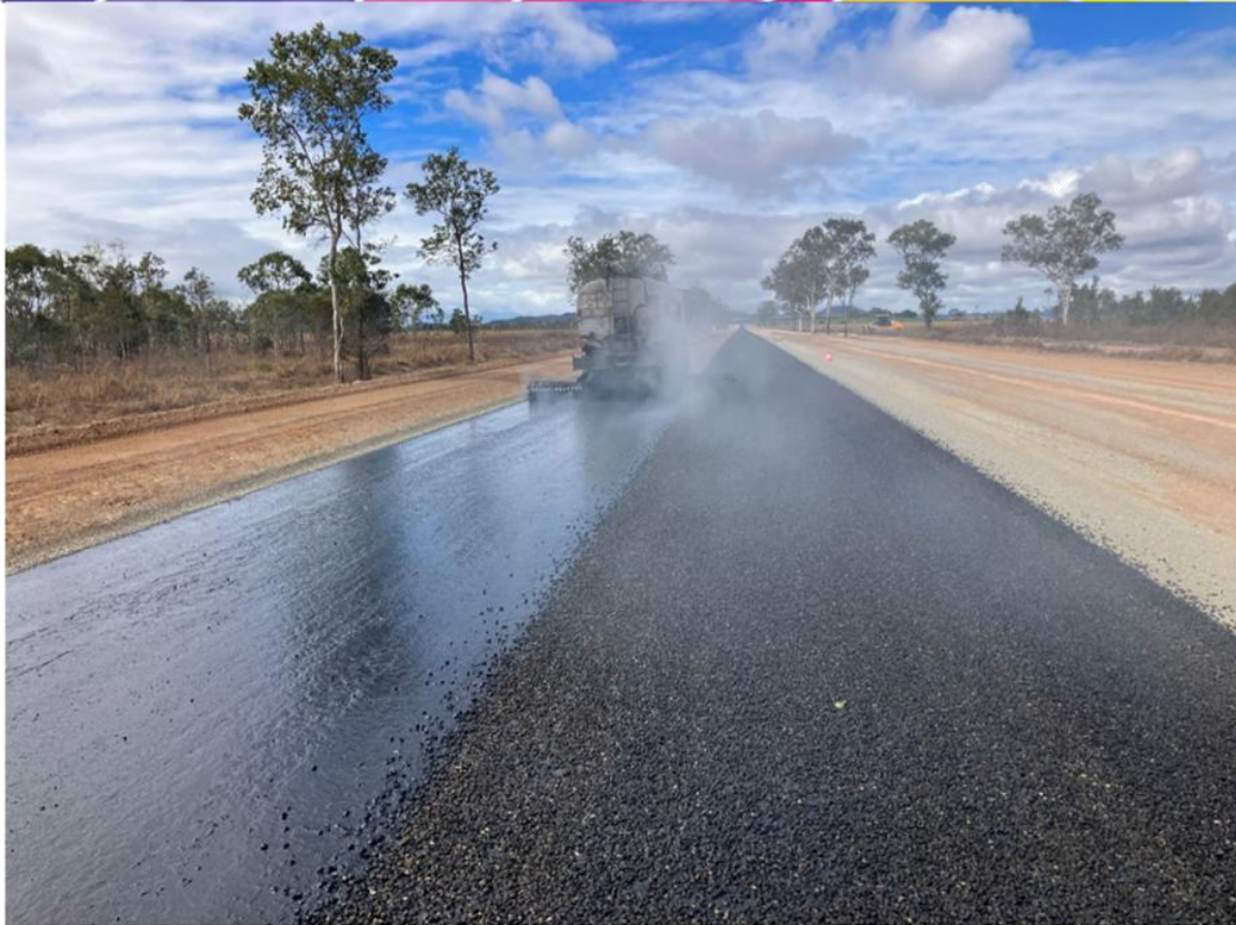
Sealing of Leedingham Road
