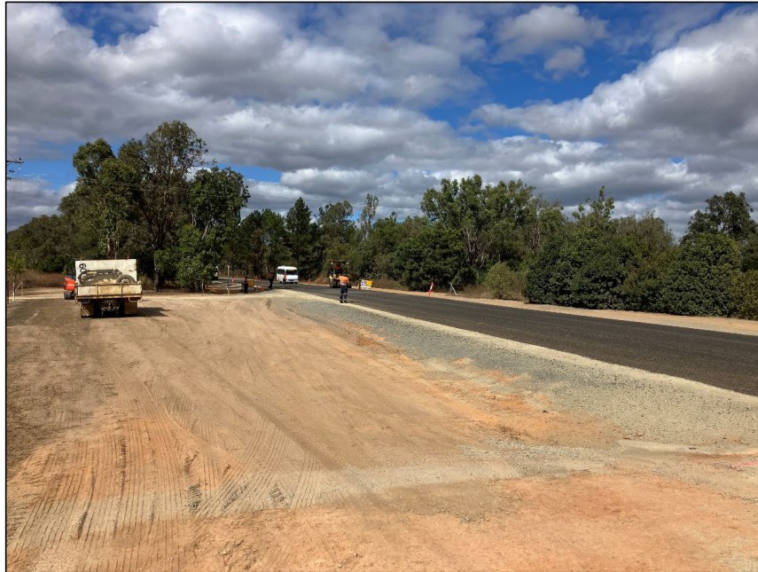
Replacement of failed subgrade
