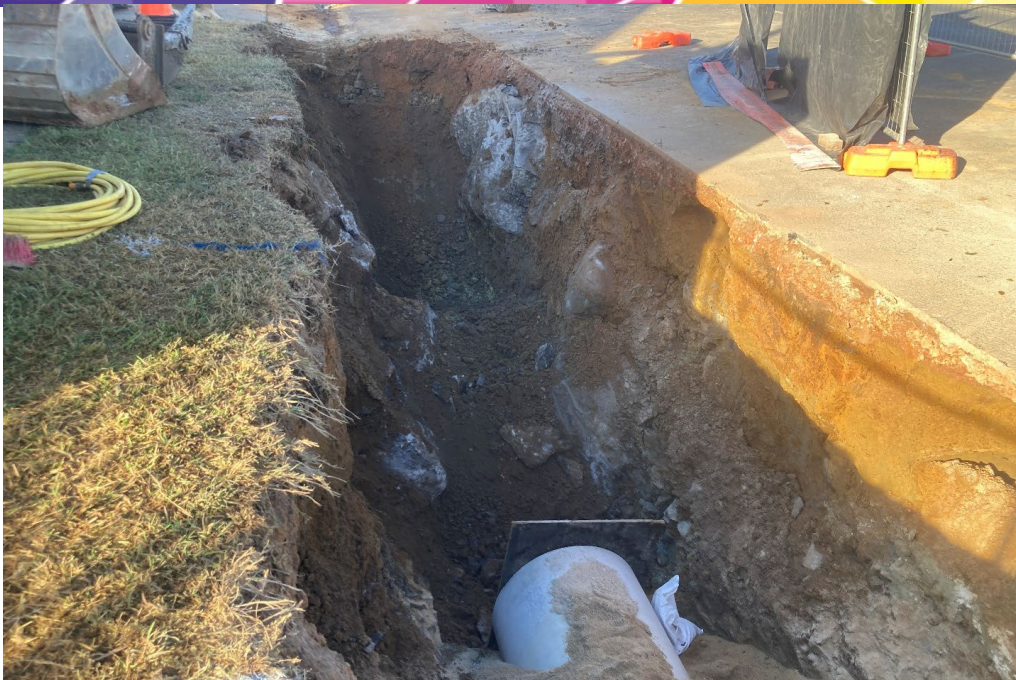
Walsh St Trench Excavation Opposite RSL/ Church Hall Indicating Rock Being Encountered
