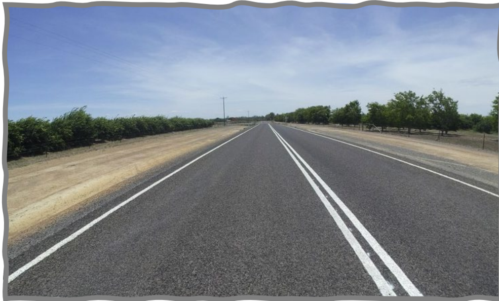
Photo 5 Dimbulah Leedingham Creek Road CH1.65-2.57
