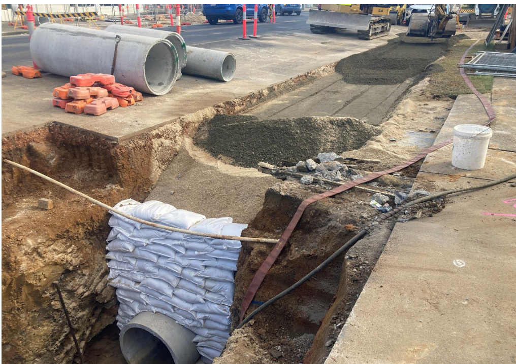
Walsh St Stormwater Installation Sand Backfill & Road-Base Laying & Compaction
