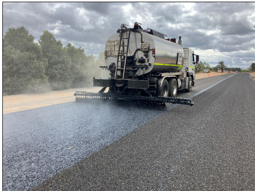
Sealing of Roadway
