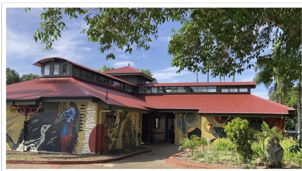
Photo 2 Kuranda Centenary Park Public Toilet Mural and Renewal
