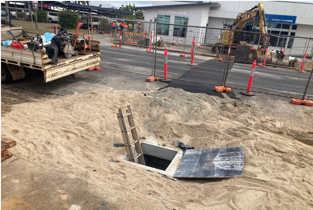
Walsh St Stormwater Pipe Crossing Pit 5/2 > Pit 1/3
