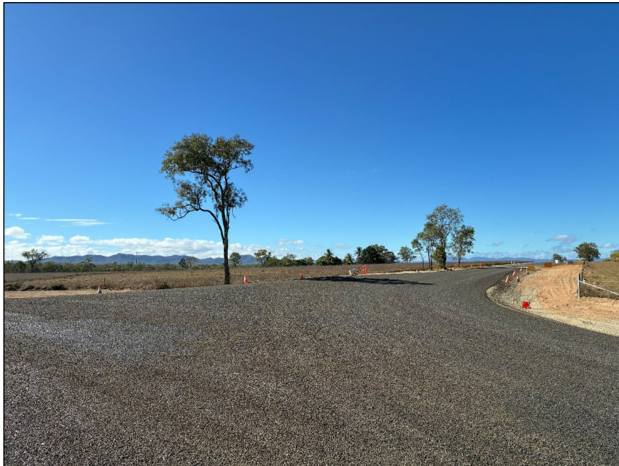
Sealing of Braund/Leadingham Intersection
