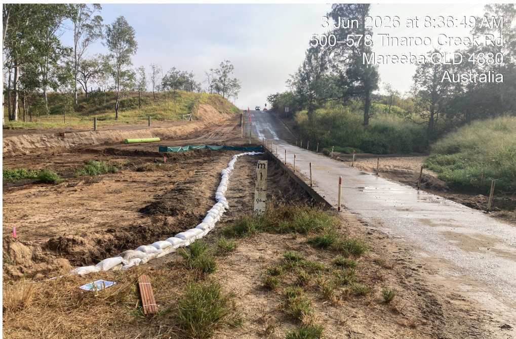
Ada Creek Stream Diversion and Side-Track Construction
