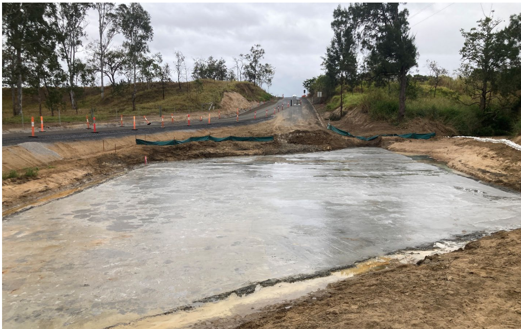
Subbase Blinding Layer Installed in Preparation for Concrete Base Construction
