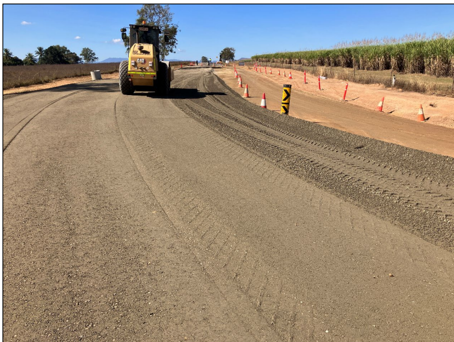
Placement and compaction of pavement
