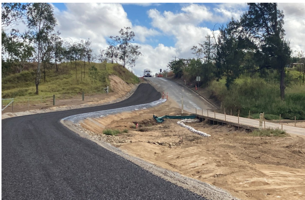
Temporary Side-Track & Traffic Lights Control
