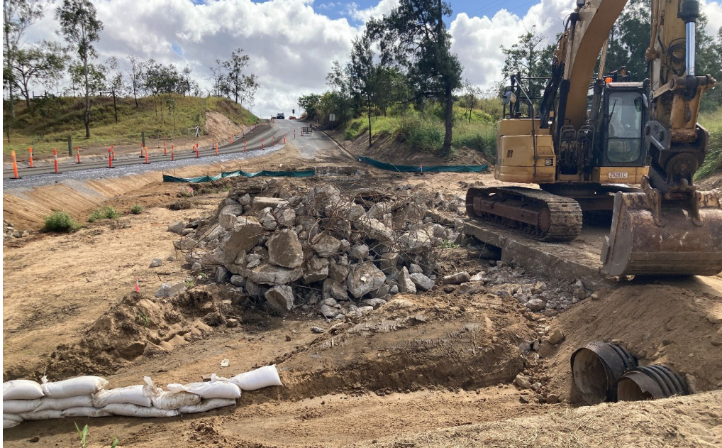
Demolition of the Old Ada Creek Causeway
