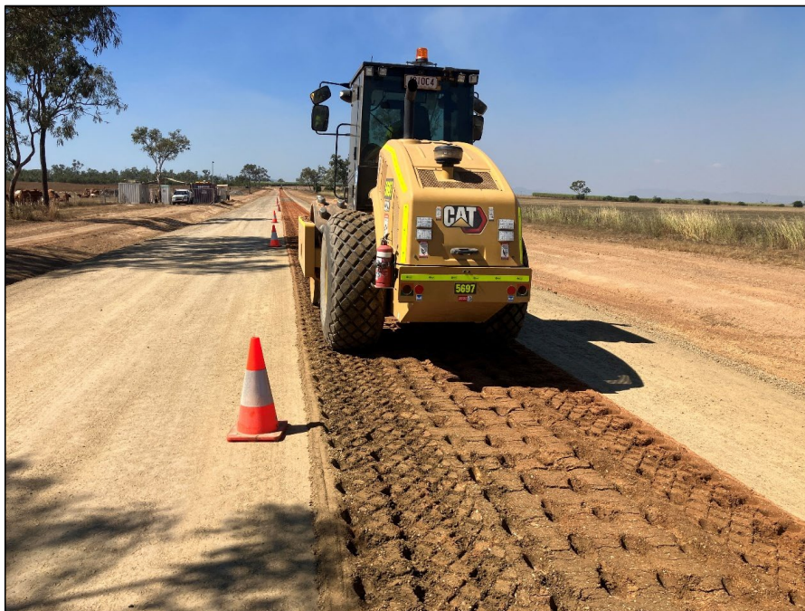
Preparation of Subgrade
