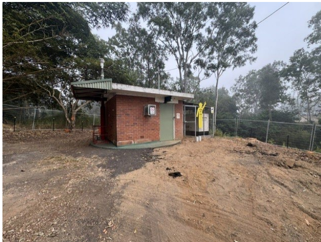
Atherton Street Sewer Pump Station Clearing, Grubbing and Excavation Works
