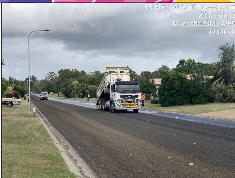
Reseal underway on Ceola Drive, Mareeba
