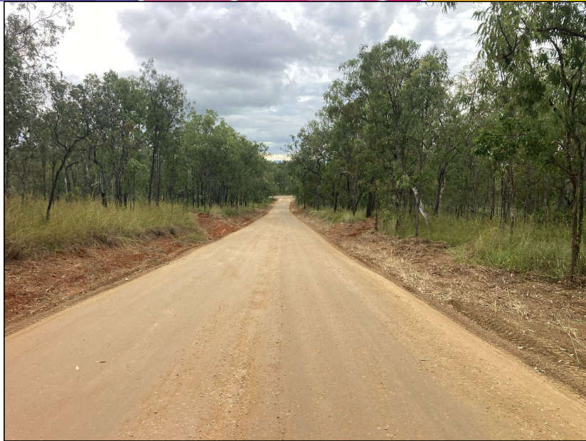
Resheet completed on Tinaroo Creek Road
