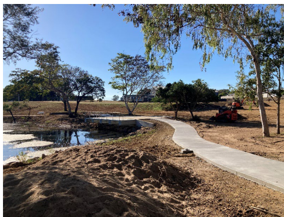
Bicentennial Lakes Northern footpath and viewing deck construction
