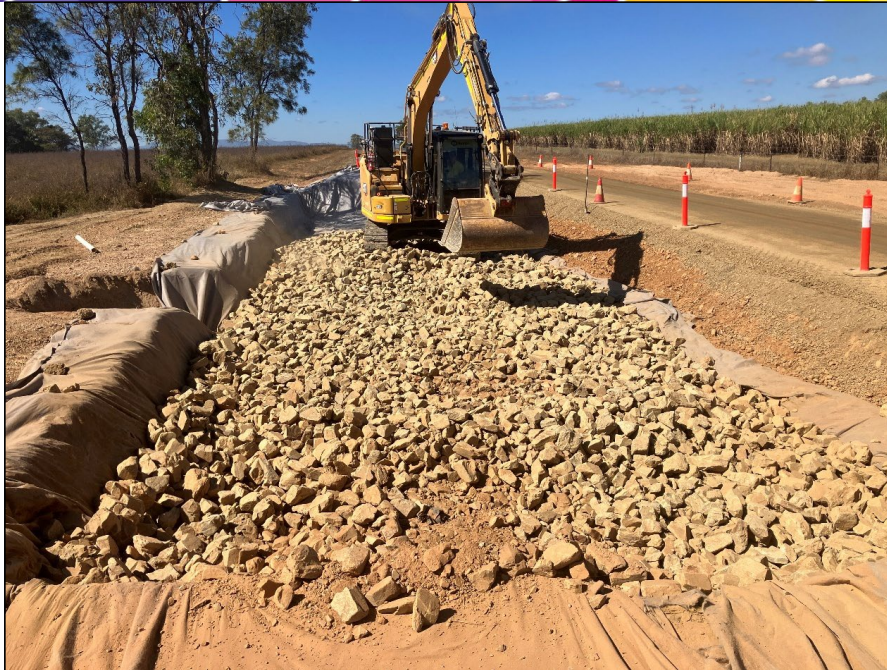
Replacement of failed subgrade
