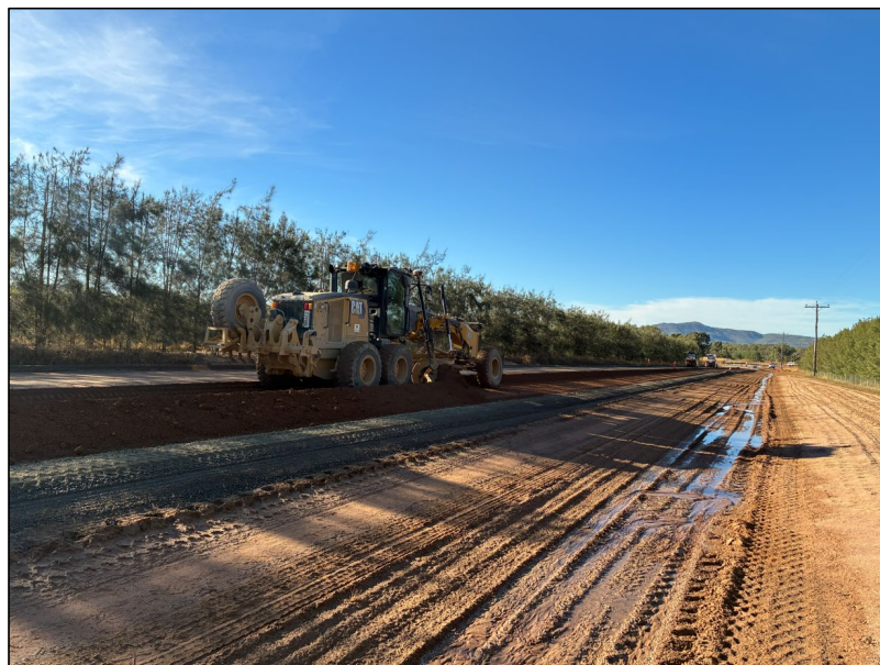
Placement of select fill
