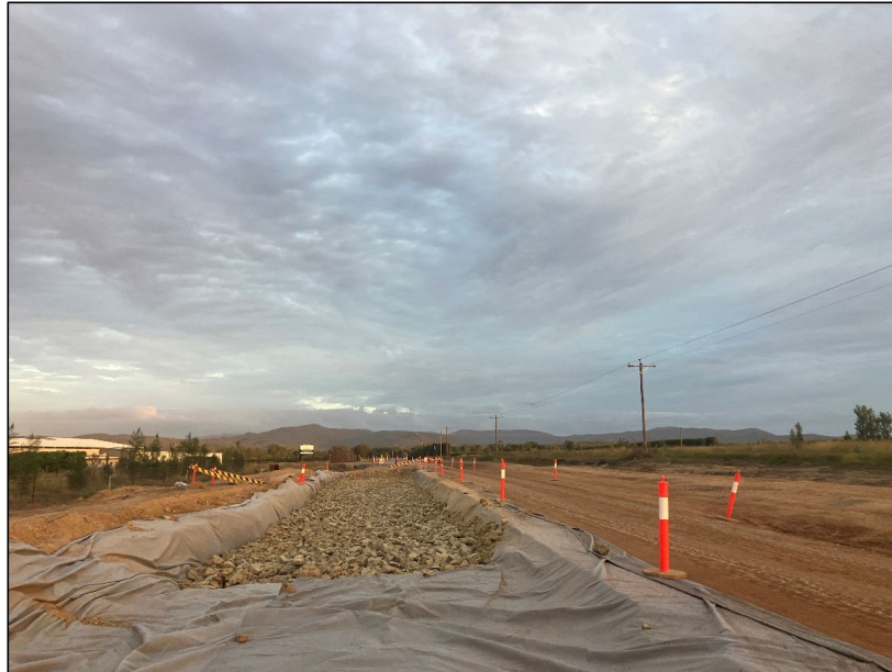
Replacement of failed subgrade
