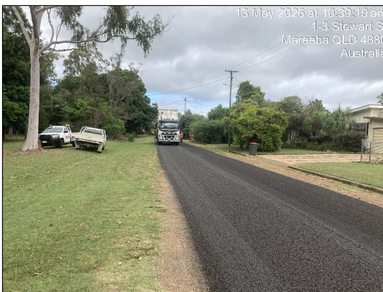
Reseal underway on Stewart Street, Mareeba
