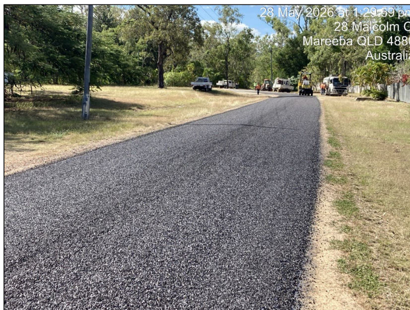
Reseal completed on Malcom Close, Mareeba
