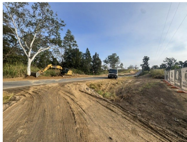
Ada Creek Causeway Upgrade Clearing, Grubbing and Side Track Construction Works
