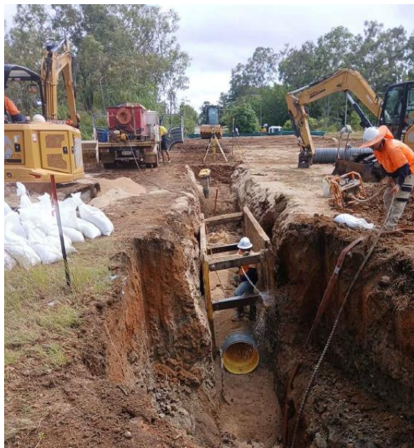
Works continuing along Constance Street towards Keneally Road, reaching Antonio Drive
