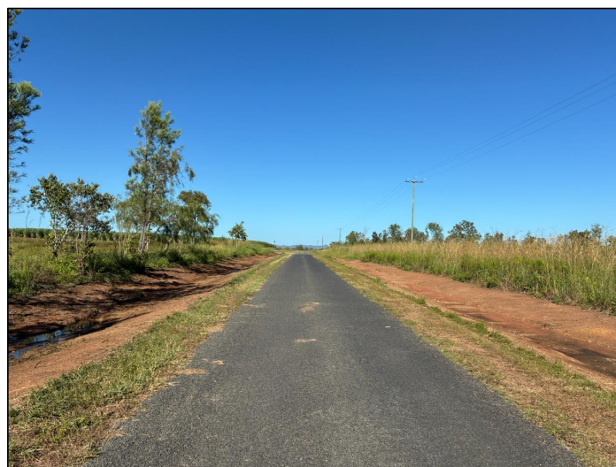
Stripping of table drains
