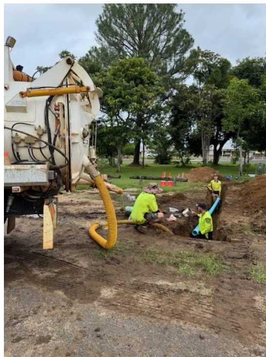
Mammino Street ‘cut ins’ and commissioning works March 2026
