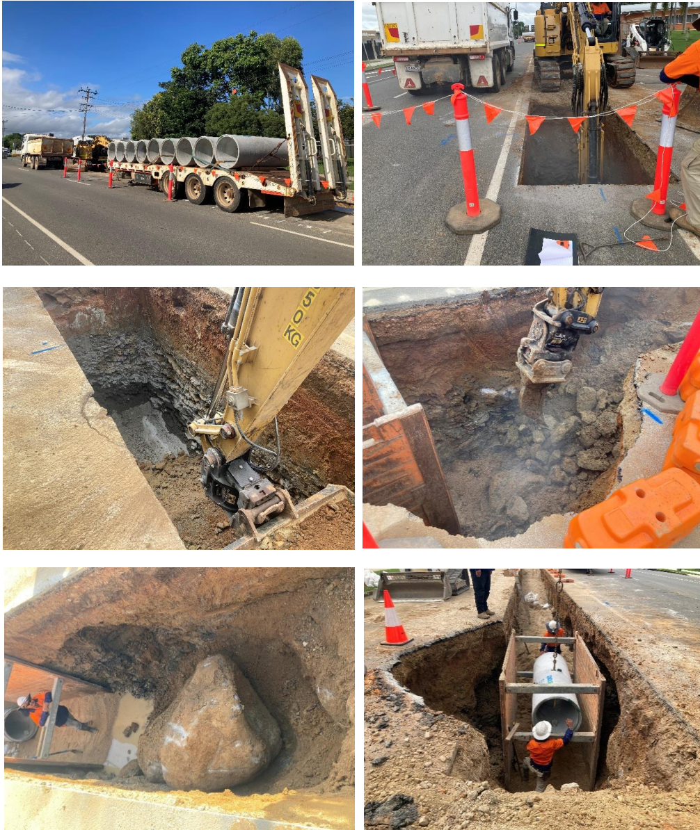
Constance Street Stormwater Pipe Trenching & Installation
