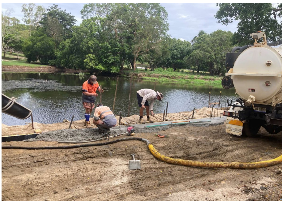
Pouring concrete for the viewing deck footings
