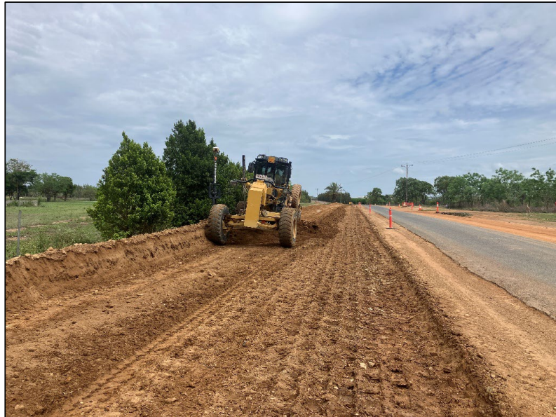
Cart, lay and compact shoulder and embankment fill
