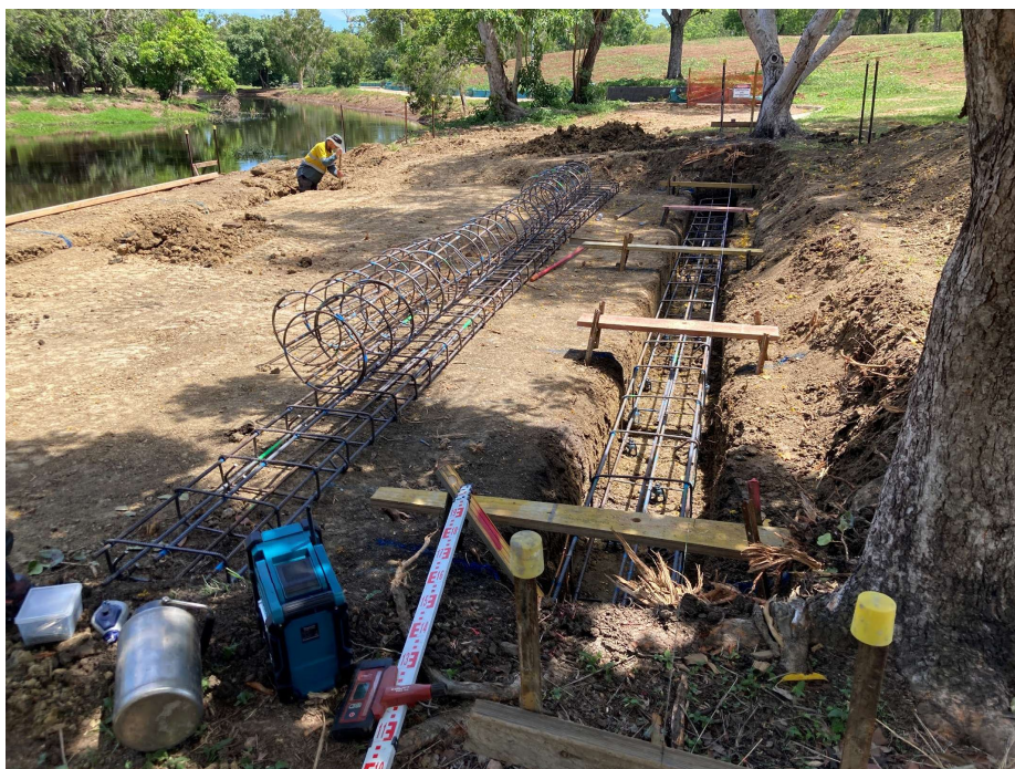
Steel reinforcing and excavation works for viewing deck footings
