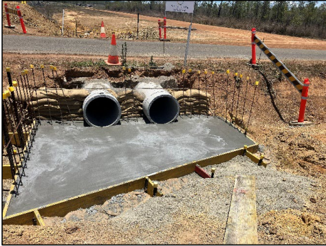
Apron and headwall works on pipe extensions
