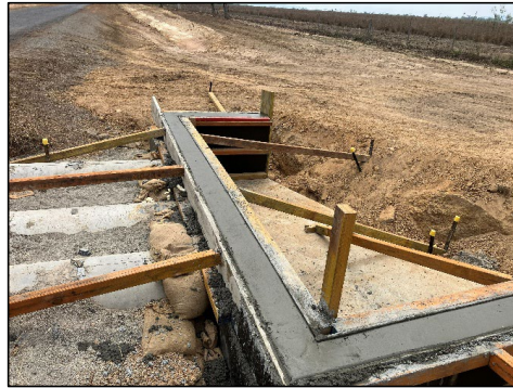
Apron and headwall works on pipe extensions
