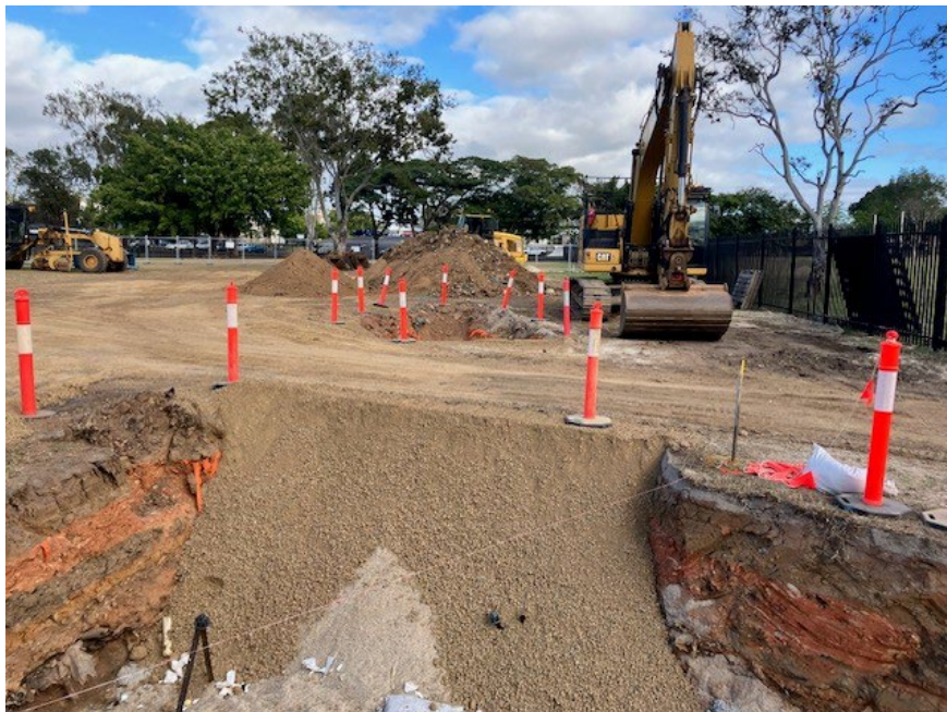
Construction of a new sewer manhole to service new gravity sewer line
