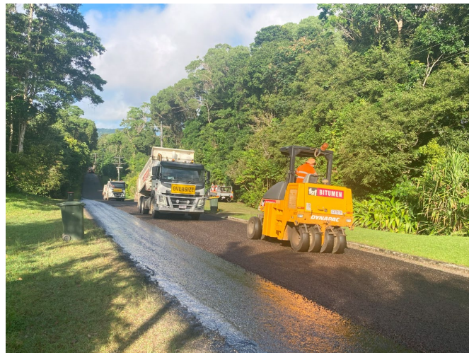
Bitumen Reseal – Barron Falls Road, Kuranda
