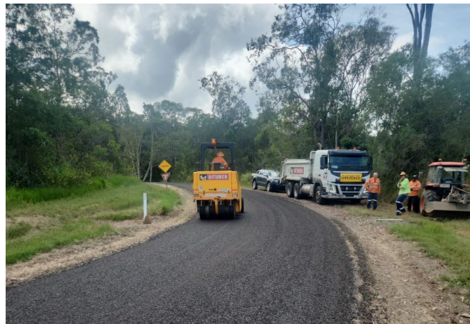
Bitumen Reseal, Bilwon Road, Bibbohra
