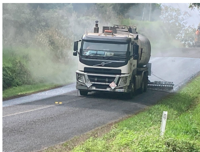
Bitumen Reseal, Speewah Road, Speewah
