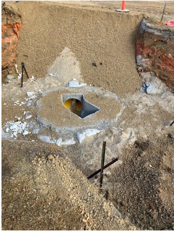
Construction of a new sewer manhole to service new gravity sewer line
