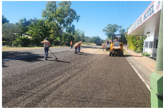
Bitumen Reseal, Tower St, Chillagoe
