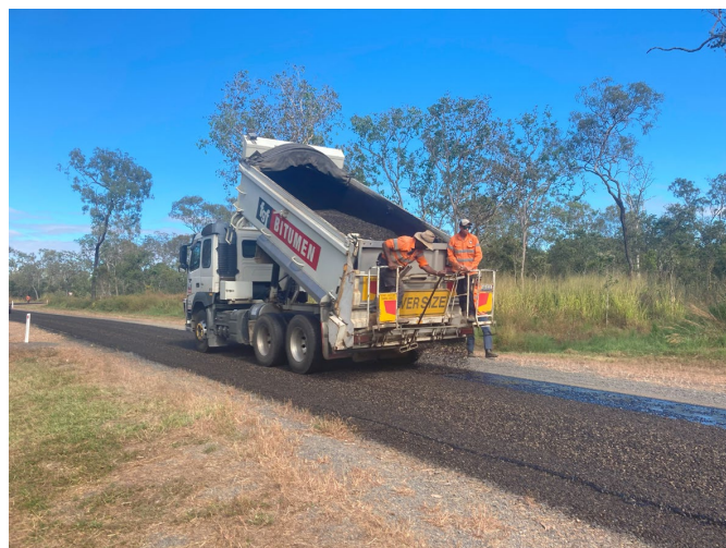
Bitumen Reseal, Volkman Road, Arriga
