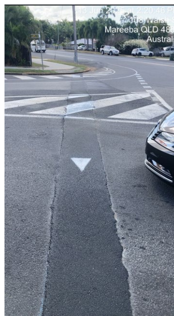
Walsh and Lloyd Street intersection. Bitumen reinstatement
