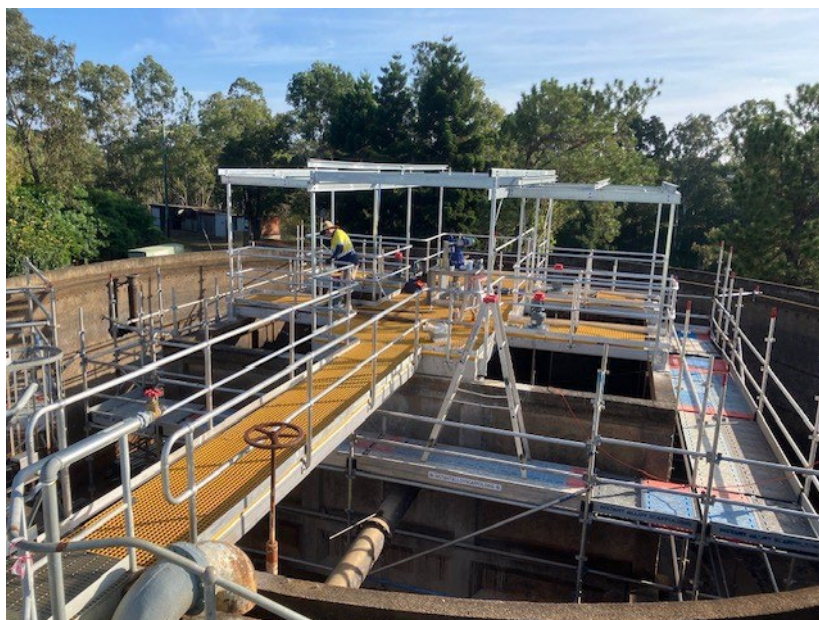
Installation of new walkway and chemical mixers.
