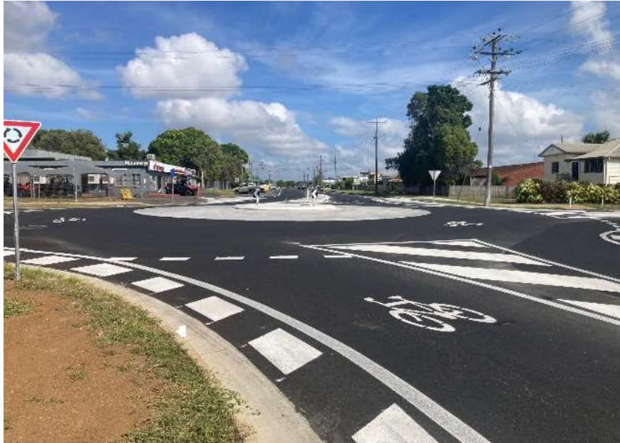
Line Marking and Road Furniture Installation
