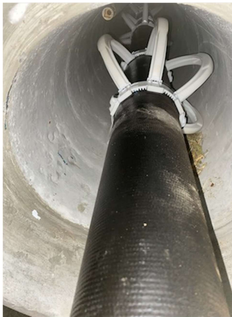
Byrnes Street crossing nightworks near Jacobsen St.
