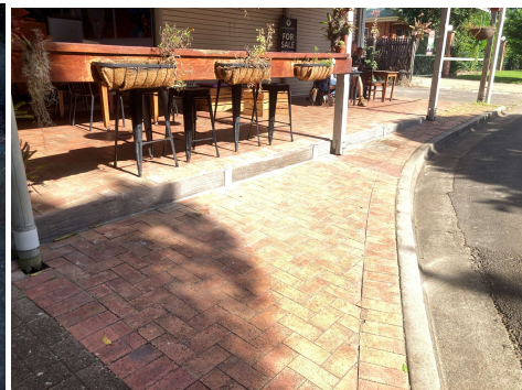
Sleeper Replacement & Paver Repair
