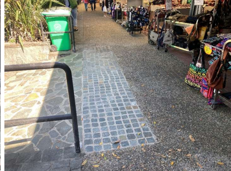
Dismantling, Reprofiling & Relaying a Section of Footpath & Ramp in Lower Coondoo Street
