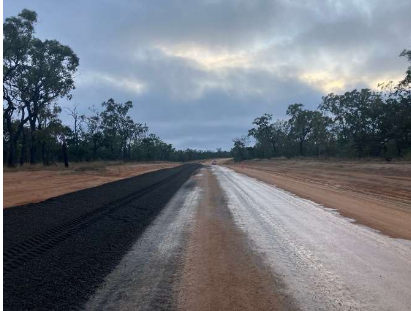
Moisture conditioned rill of 2.1 Road Base Gravel.
