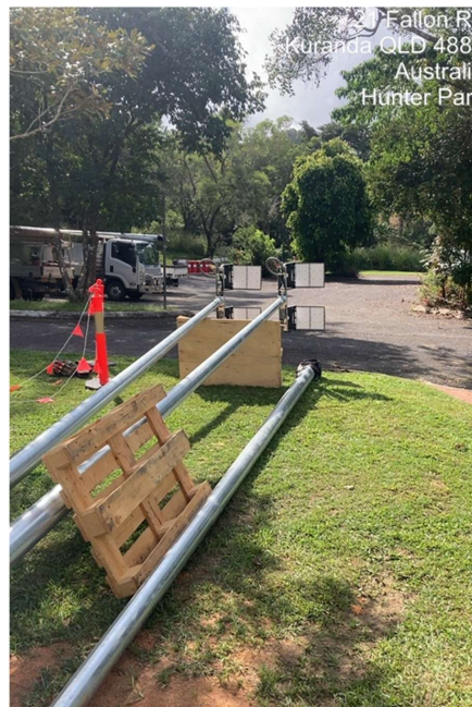
New light poles and LEDs ready for installation
