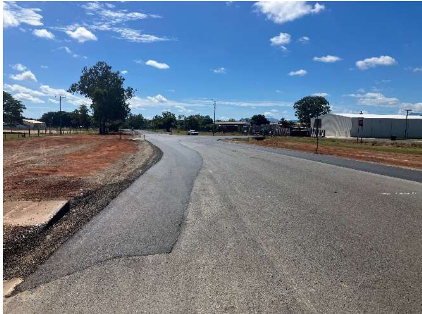
Asphalt Overlay Reynold St Intersection
