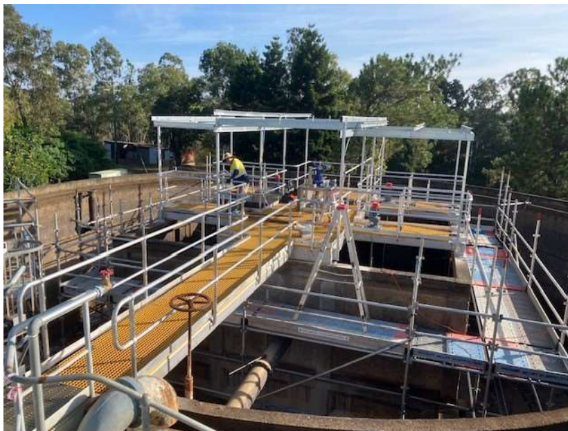
Installation of new walkway and chemical mixers.
