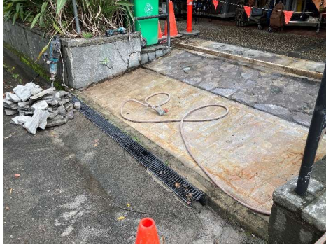
Dismantling, Reprofiling & Relaying a Section of Footpath & Ramp in Lower Coondoo Street
