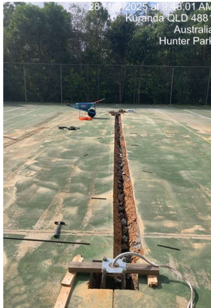
Trenching, cabling and footings for new light poles
