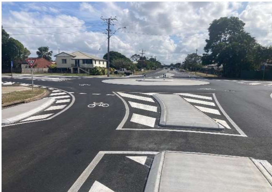
Line Marking and Road Furniture Installation
