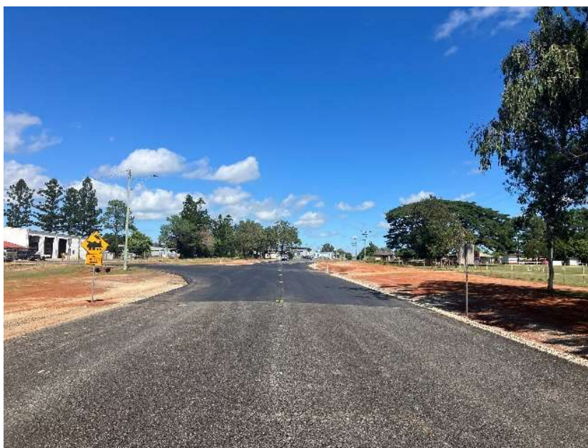
Asphalt Overlay Reynold St Intersection
