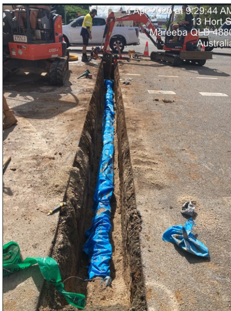
Installation of 100mm Ductile Iron pipe. Hort Street, Mareeba
