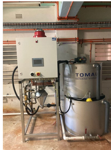
Installation of new chemical dosing equipment.
