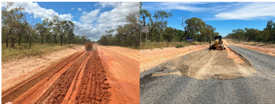
Watering existing subgrade prior to trimming
