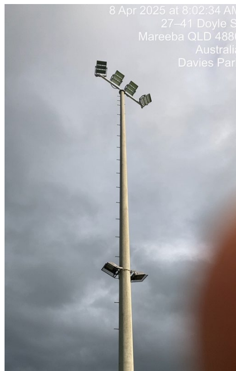
Completed headframe and luminaires
