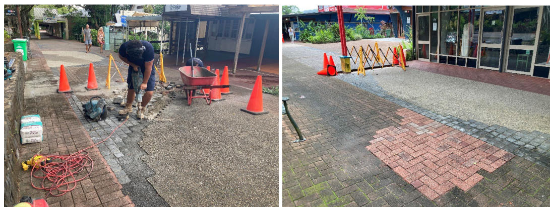
Replacement of Displaced Slab in Front of the Chemist - Corner of Coondoo & Thongon Streets
