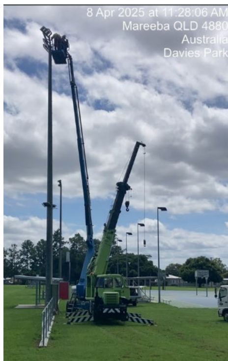
Installation of headframes
