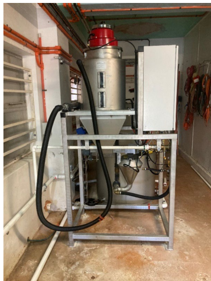
Installation of new chemical dosing equipment.
