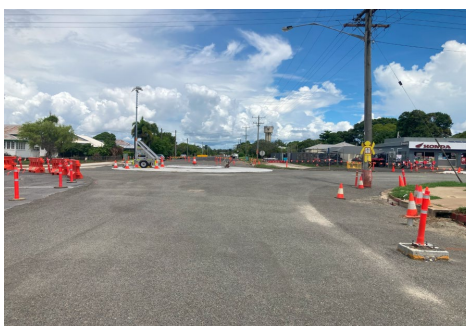
Base gravel – laid and compacted
