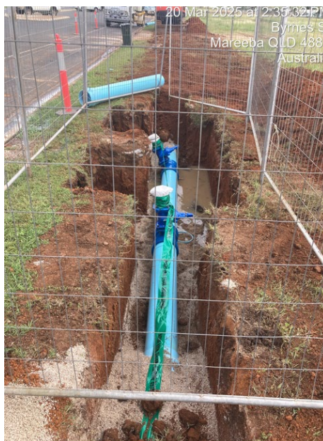
T-intersection with sluice valves. Byrnes St, Mareeba.
