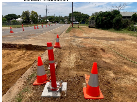
Completed rag bolt installation
