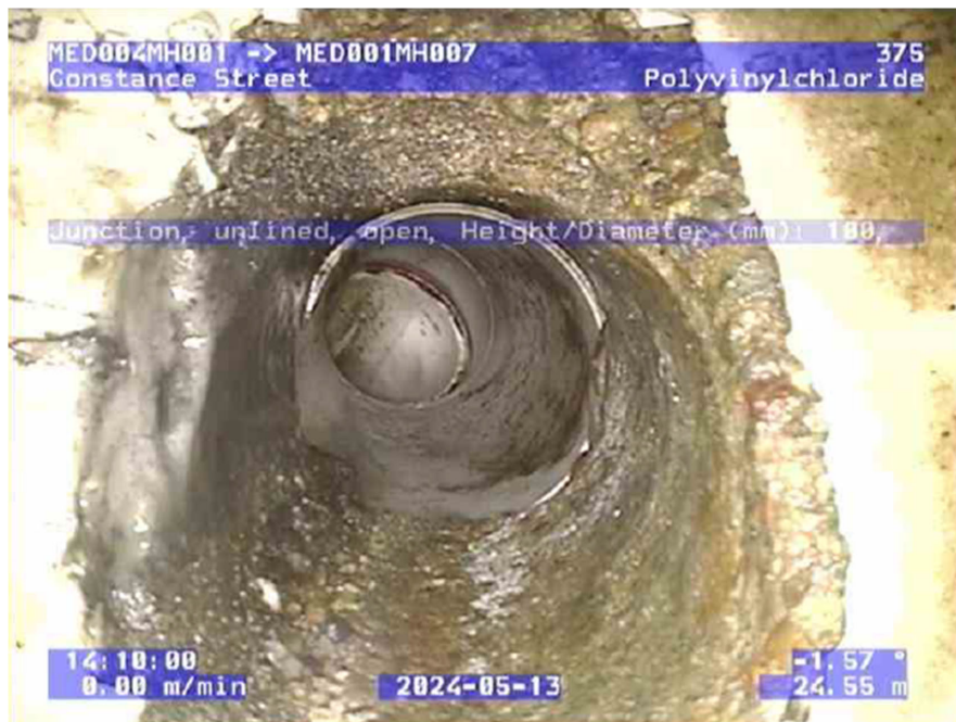
Captured image of identified defective sewer junction
