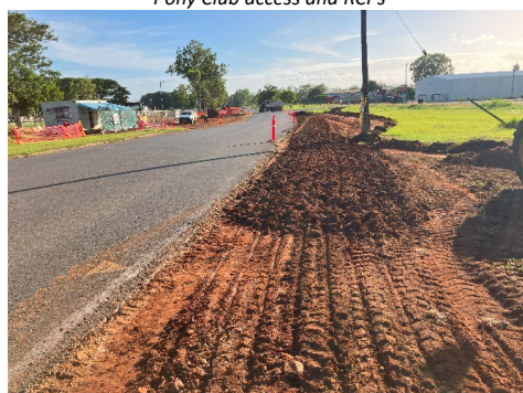
Drainage excavation – Reynolds Steet side
