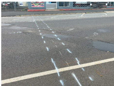
Marked trench for conduit
