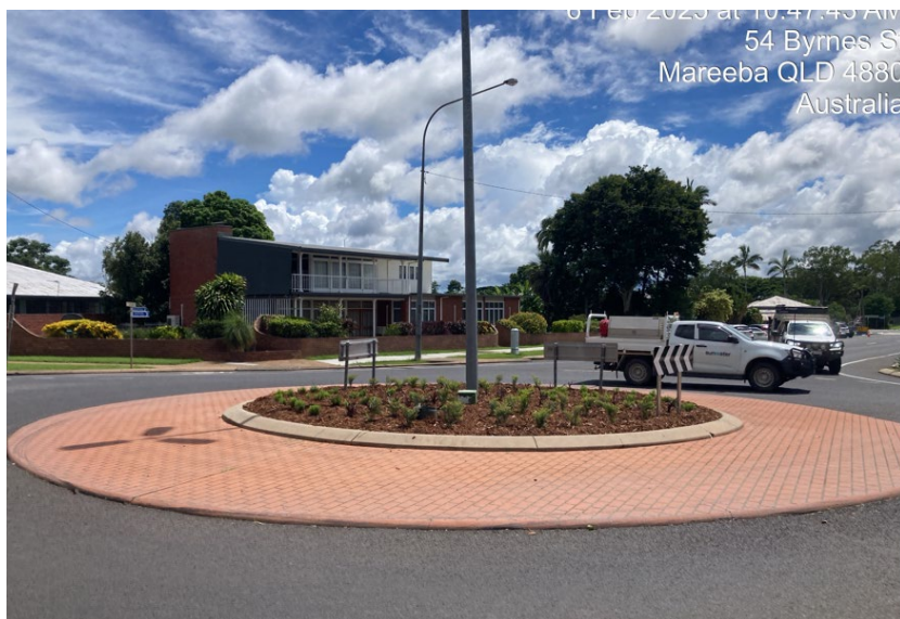
Location 4 – Roundabout, Byrnes Street.
